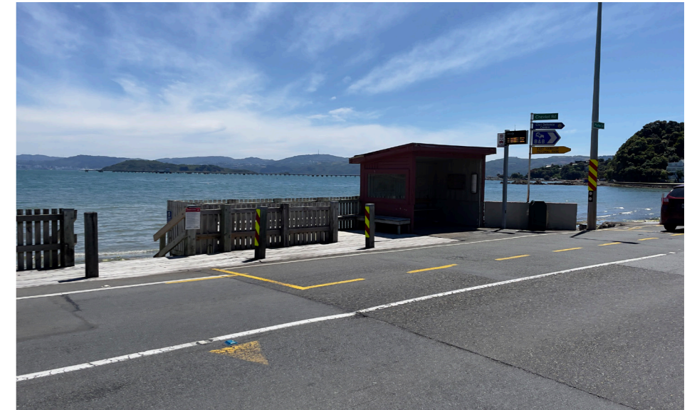
Figure 1.30 Whiorau Bay Bus Stop
