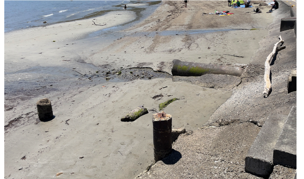
Figure 1.6 Existing stream and culvert in Whiorau Bay
