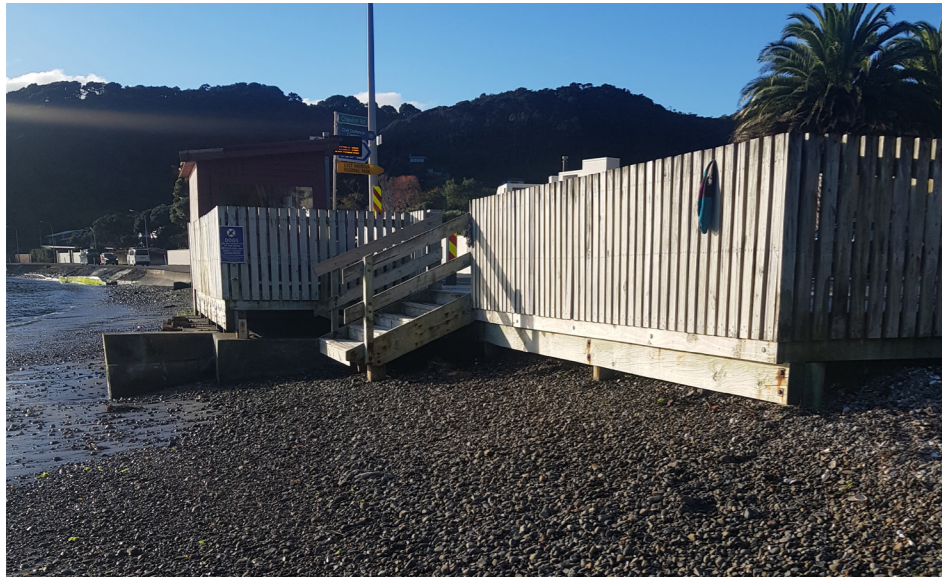
Figure 1.7 Decking structure around existing bus stop.
