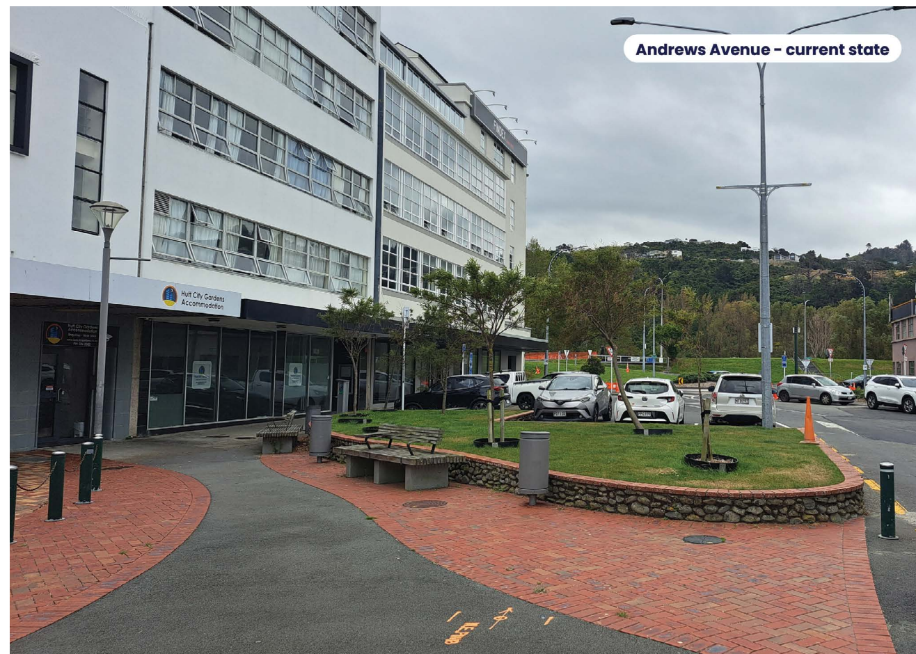
Figure 5.3.1 Existing condition of Andrews Avenue
