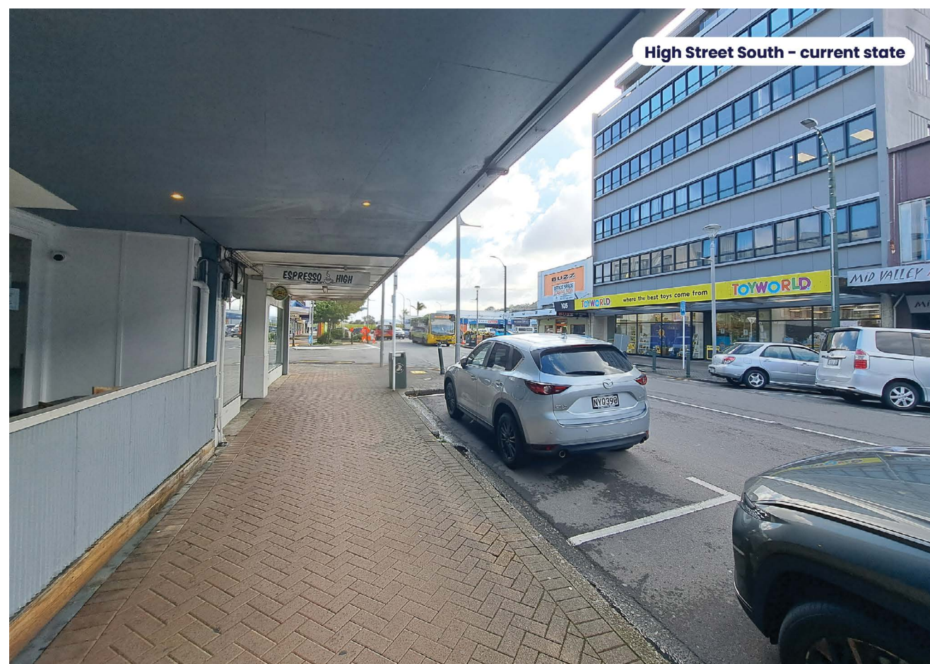
Figure 5.1.1 Existing condition of High Street South
