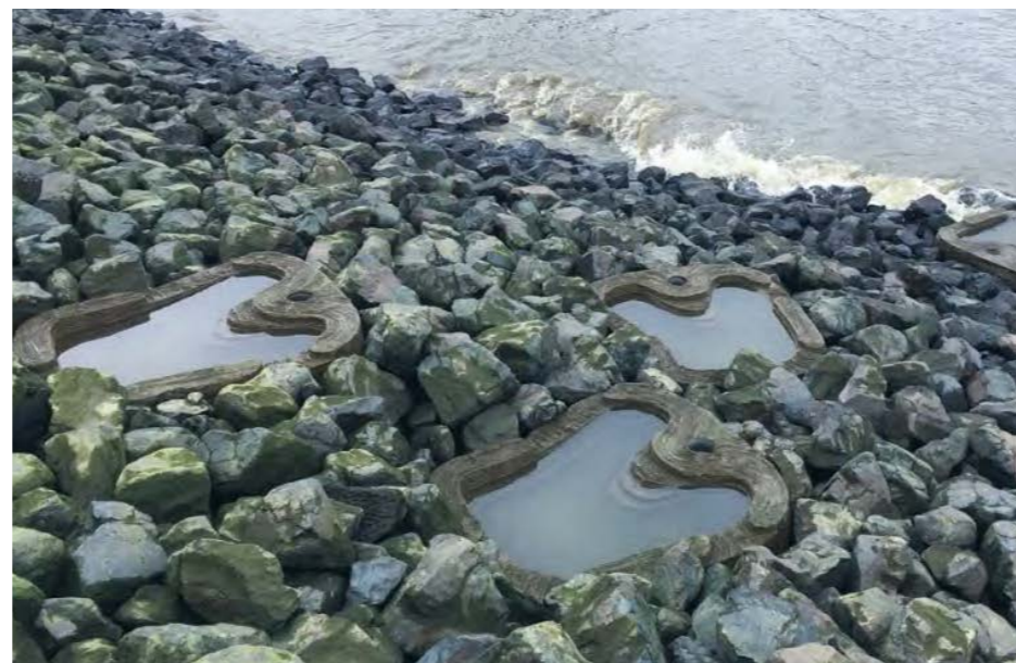
Figure 1.22 Tide pools installed in rock revetment. Ref SHRP
