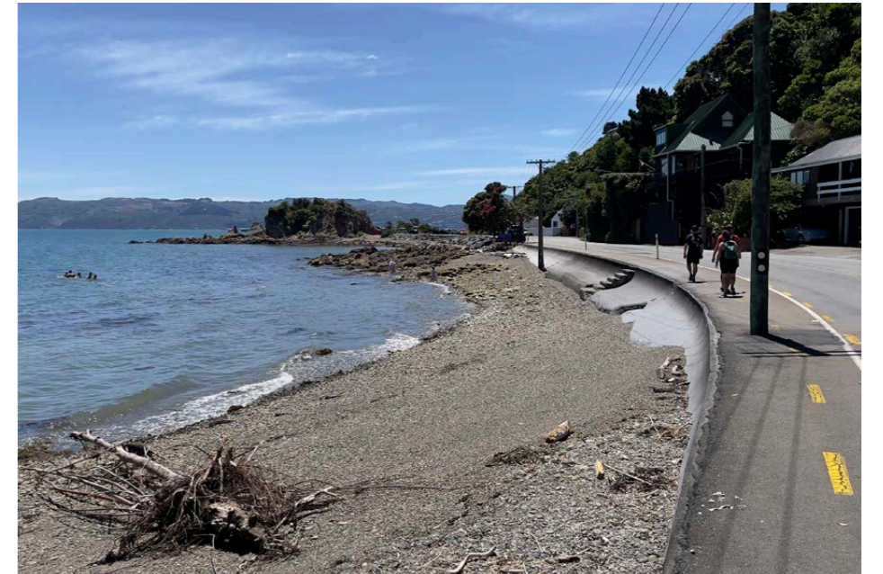
Figure 1.6 Existing seawall at Mahina Bay.
