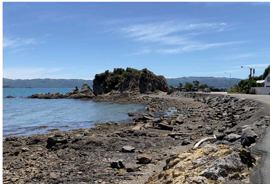
Figure 1.7 Existing revetment and rocky outcrop at north Mahina Bay.
