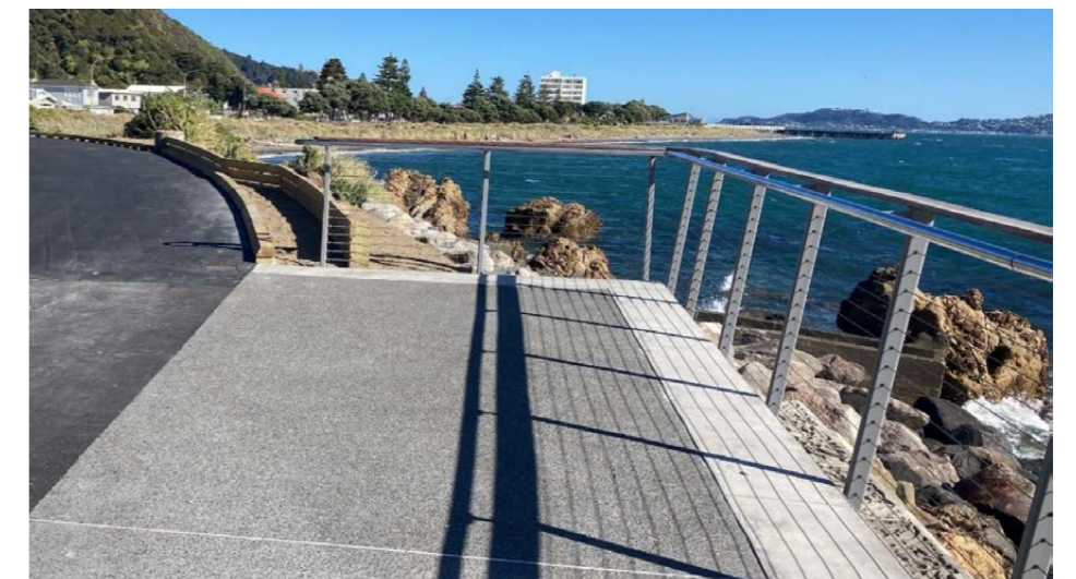
Figure 1.18 Completed balustrade at southern end of Mā-koromiko.
