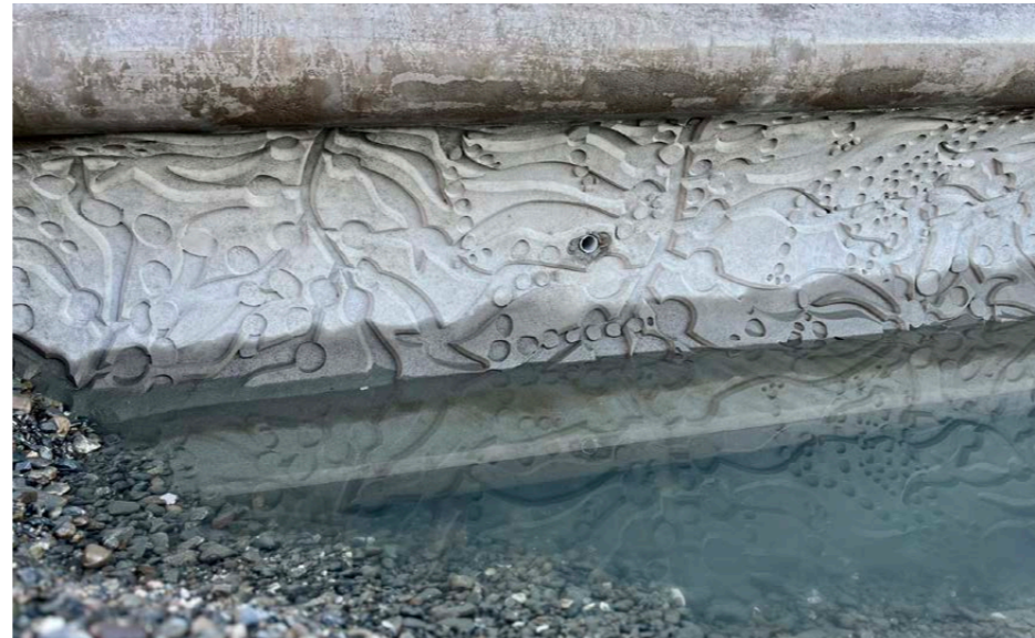
Figure 1.19 Photo of texture applied to curved seawalls vertical faces.
