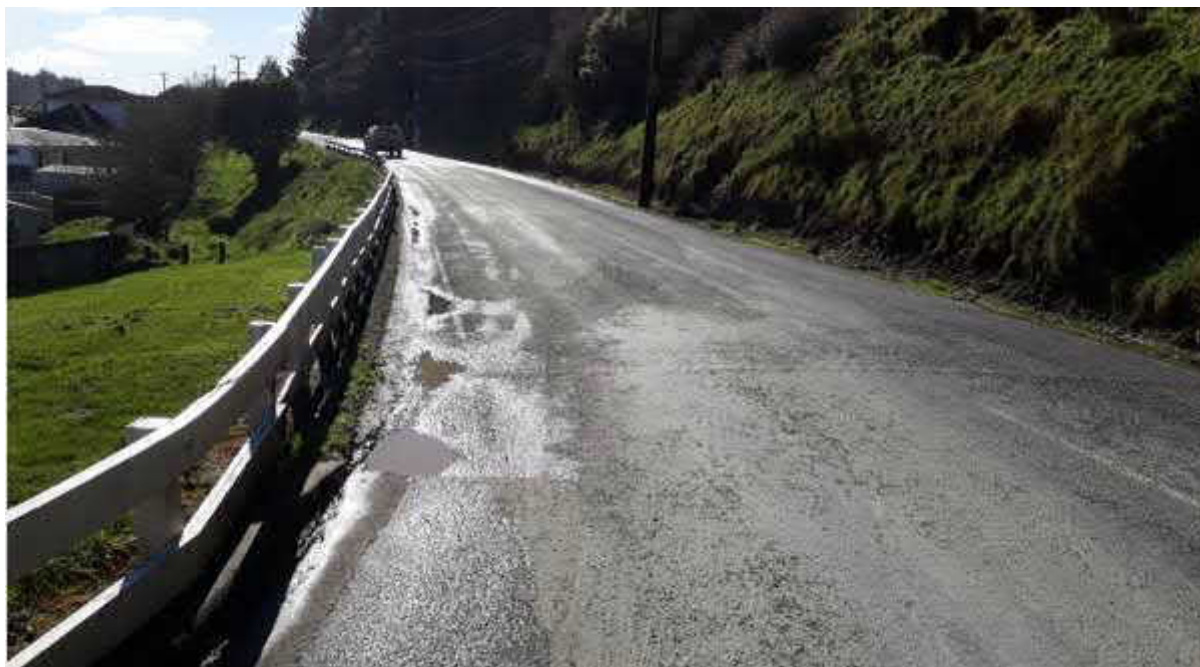
Figure 3 – Coast Road, looking north from the cleanfill access towards Parenga Street
