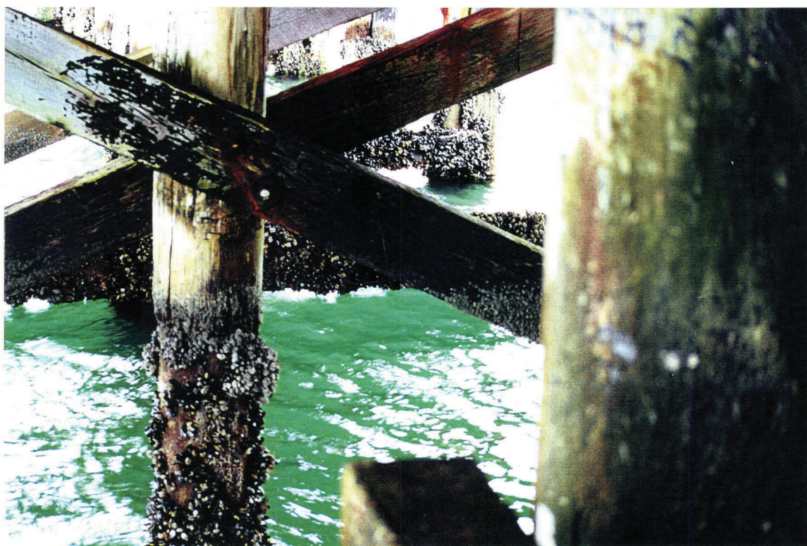
Photo 4: Typical view under Central Head (Looking South)
