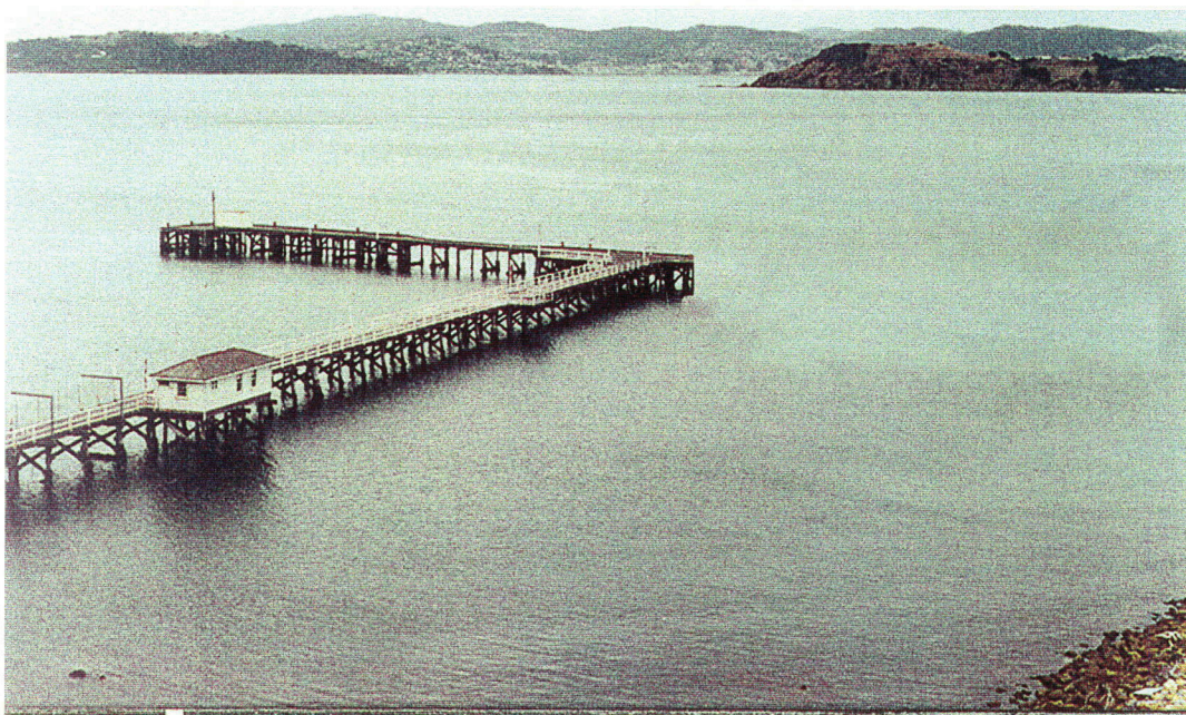
Option 3A Demolish North Head
