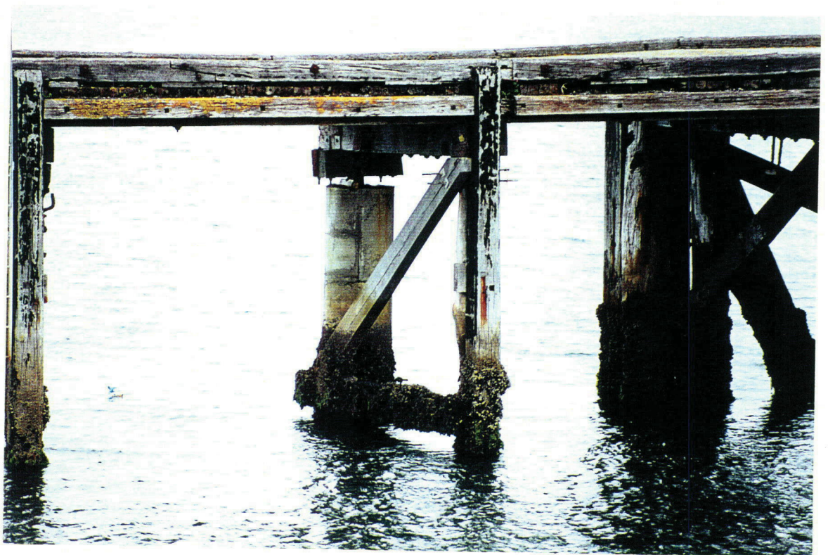
Photo 2: North Head Note Concrete jacket on pile AA41
