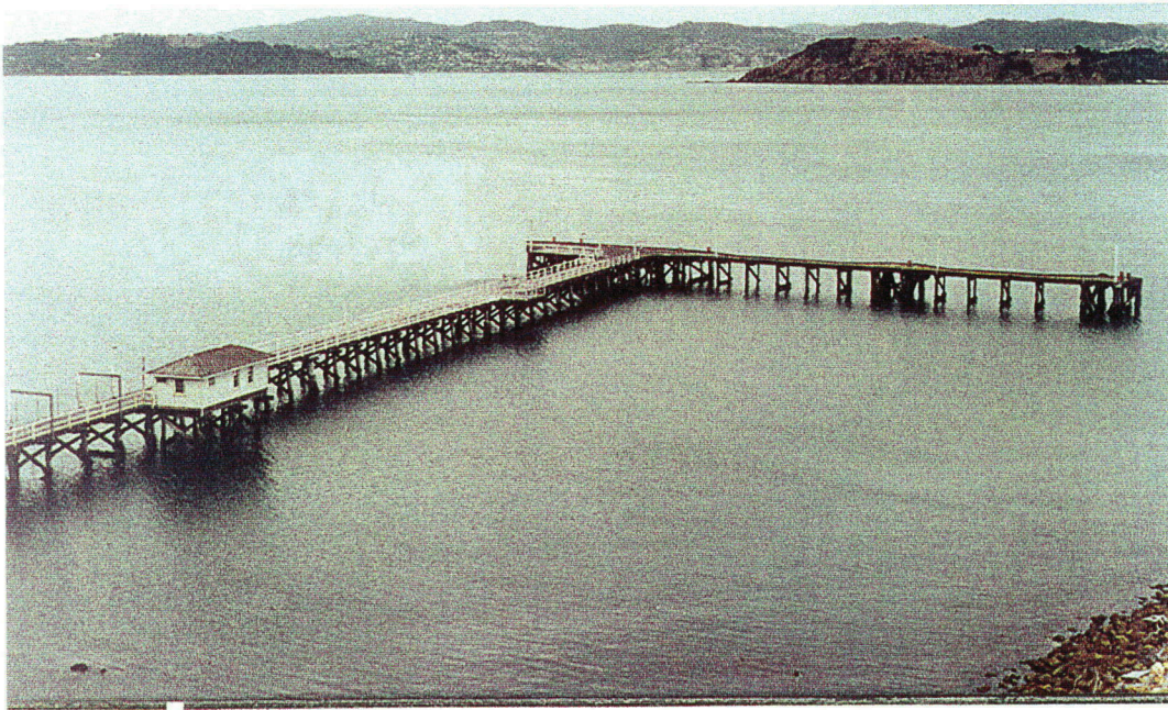
Option 3B Demolish South Head
