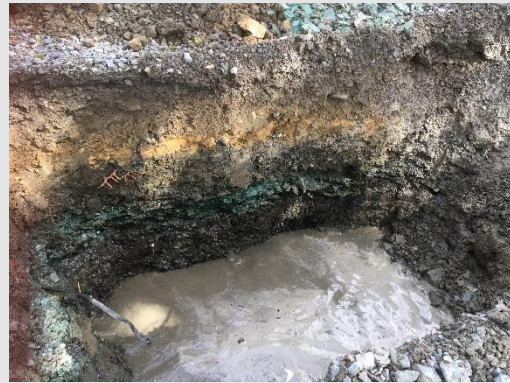
Photo 6: Location L31 – glass layer visible (Zone 4)
