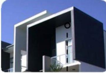
Horizontal shading device (overhangs) on north facing
