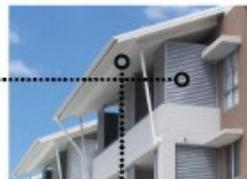
Horizontal Shading device (overhangs) on north facing windows
