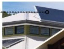
Eaves and moveable vertical shading device (external venetian blind) on east or west facing windows
