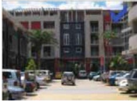
Current building on prominent site
