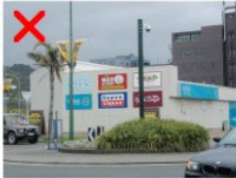
Current building on prominent site
