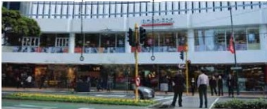
Example of a Street Frontage Type 1 - Borders - Wellington CBD
