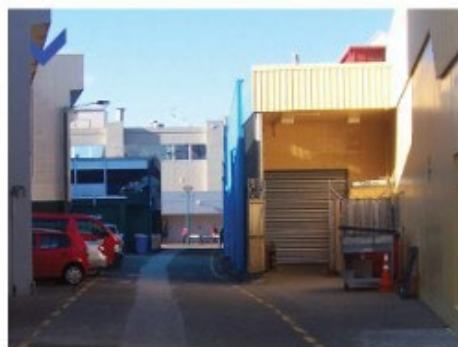
Loading zone at the rear of the buildings and accessed by a rearlane
