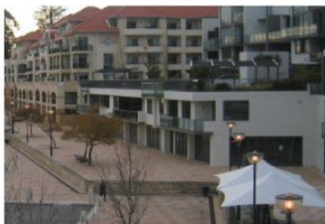
Riverfront (Core) future character - river promenade, active and sheltered frontages to reserve, residential above retail (shops, cafes and/or restaurants) and terrace garden
