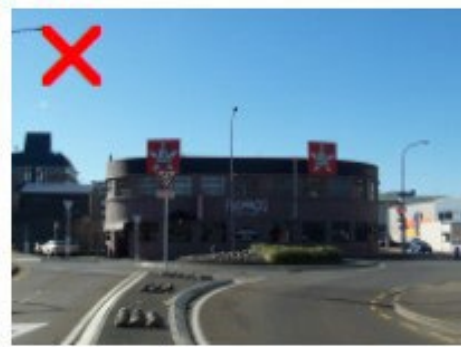
Current building on prominent site
