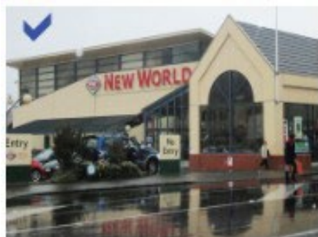
Signage below roofline
