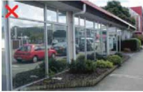
Reflective windows do not offer visual connection between interior and exterior - "cannot see through"
