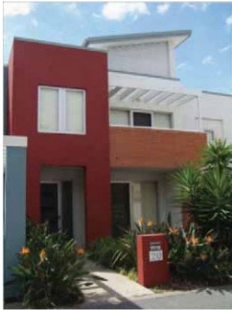
Small front yard, porch, balcony, living spaces and windows fronting the street
