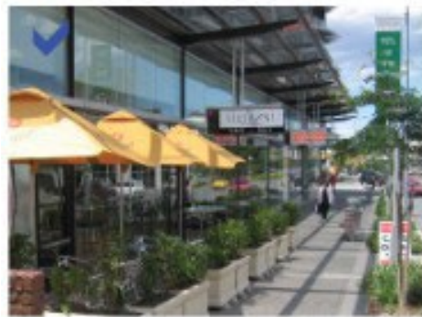
Signage attached to the verandahs
