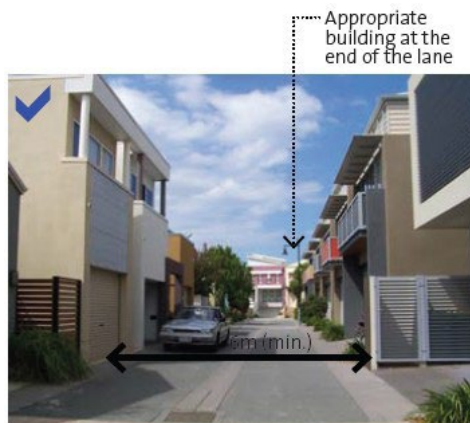
Rear lanes in medium density residential developments. "Eyes on the lane" - studios above garage with balconies and windows facing the lane. Landscaping, lighting and screened bins also enhance its appearance
