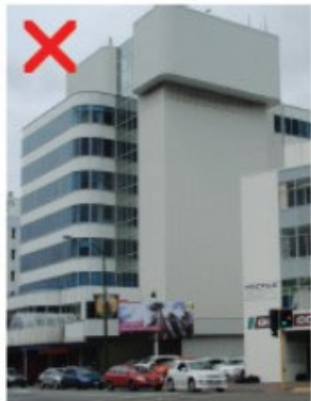
Taller building - blank side wall
