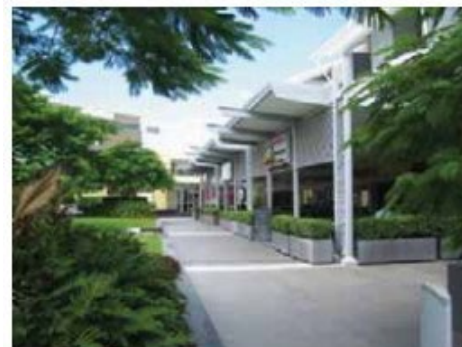
Riverfront (Core) - restaurants fronting onto the promenade and the park, continuous verandahs, high quality landscaping, vertical screens for shade in summer; appropriate signage and quality materials
