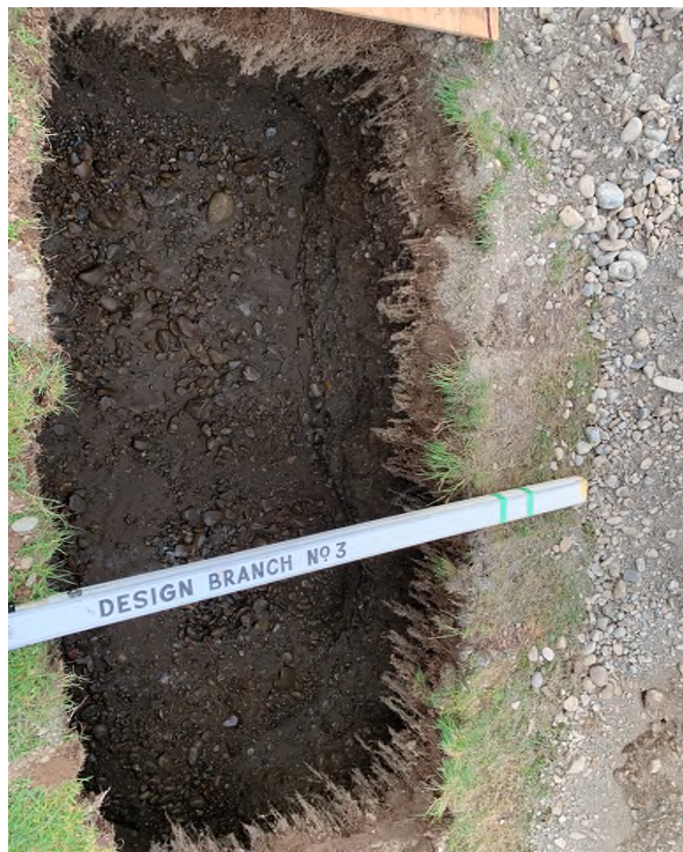
Above: View of excavated pit at test location 3 at completion
