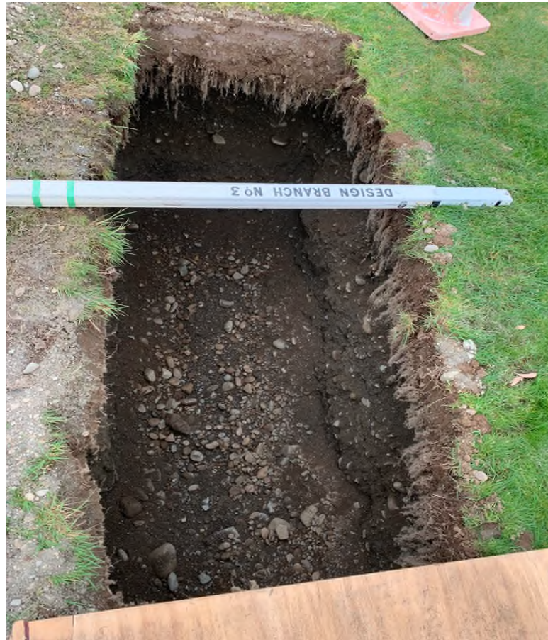
Above: View of excavated pit at test location 3
