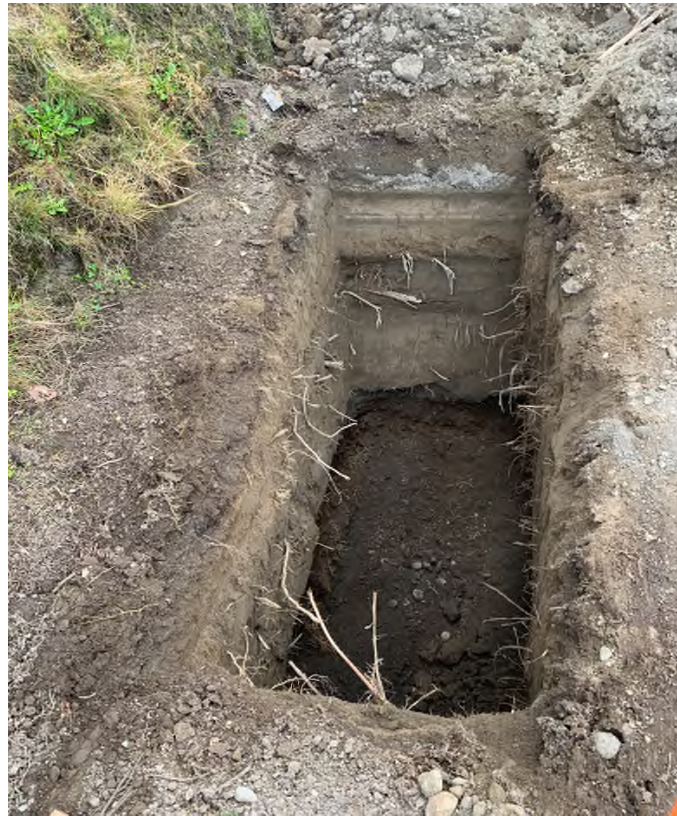
Above: View of excavated pit at test location 1
