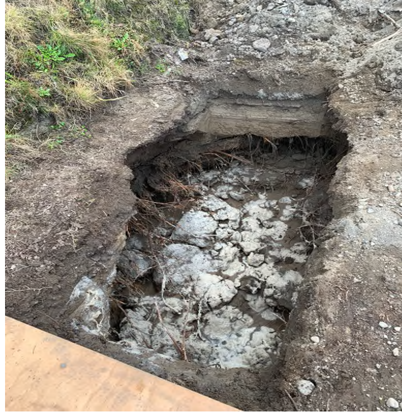
Above: View of excavated pit at test location 1 at completion
