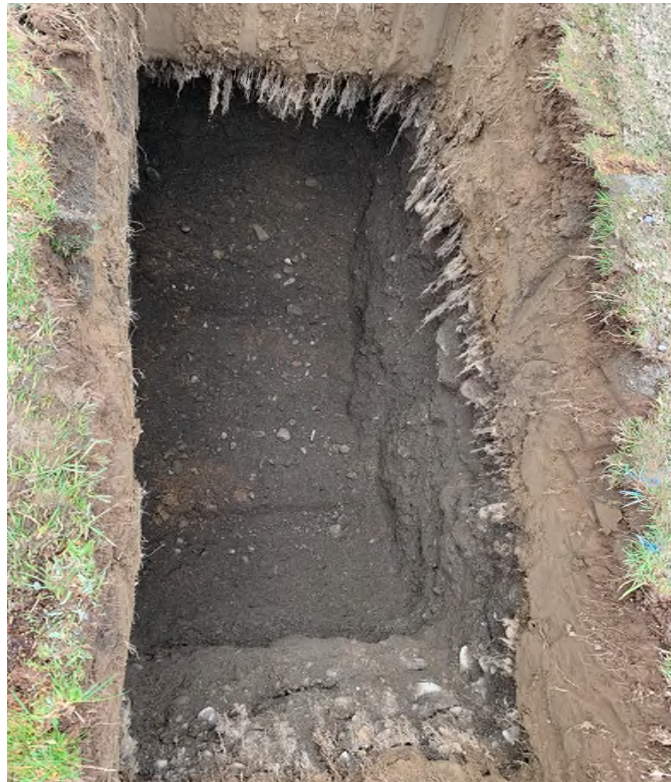
Above: View of excavated pit at test location 2
