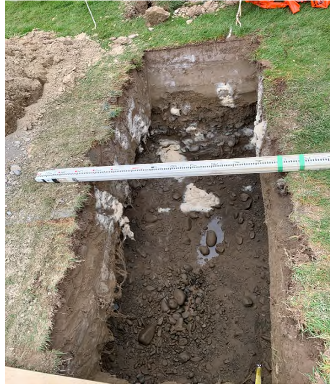
Above: View of excavated pit at test location 2 at completion
