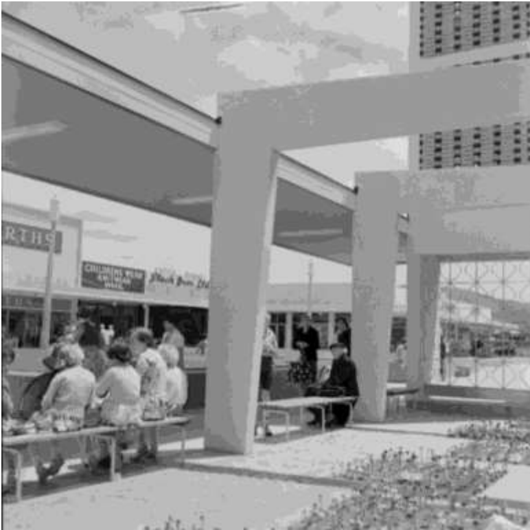
Figure 17: Exterior courtyard showing ornamental garden, veranda, screen and cantilevered beams, circa 1960. Source: Alexander Turnbull Library, EP/1959/4122-F
