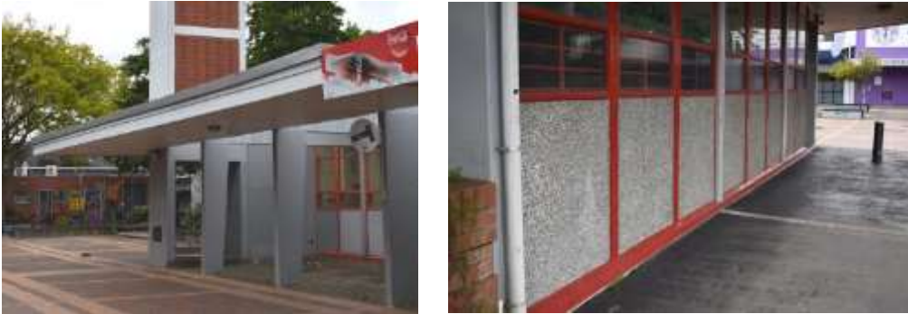
Figures 2 and 3: south-western elevation (left) with cantilevered beams and courtyard; north-western elevation (right) with stone aggregate panelling.
