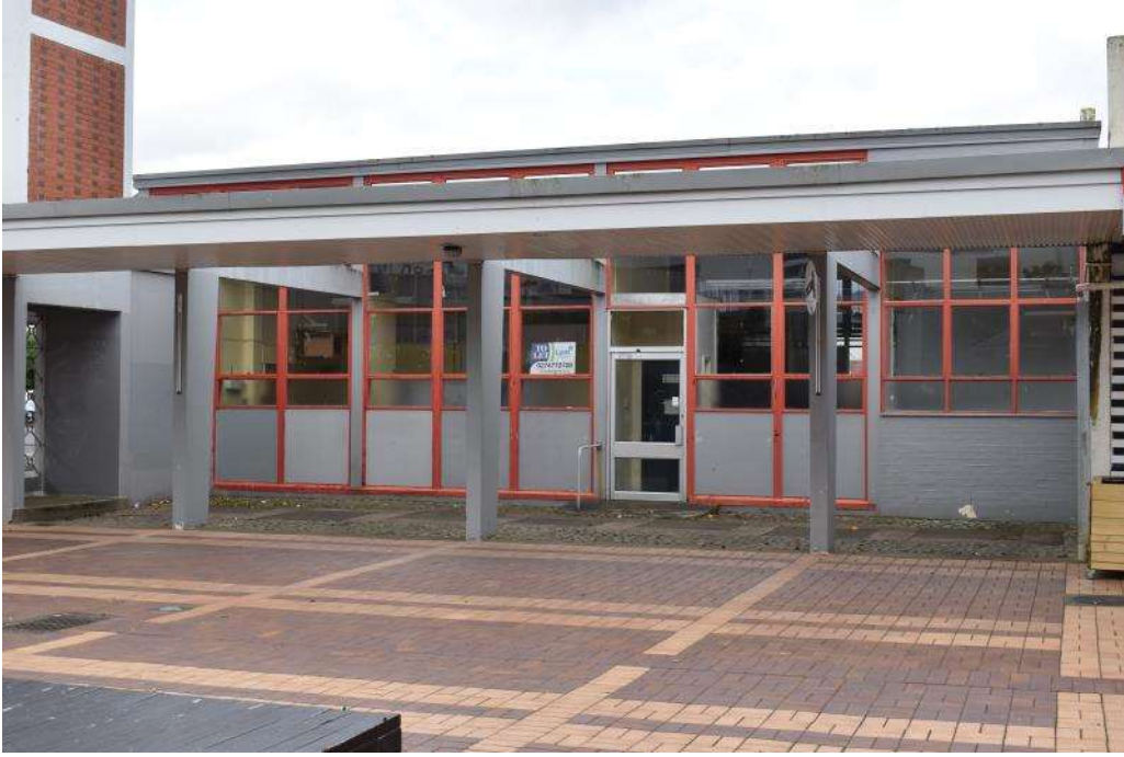
Figure 19: south-western elevation. This side of the building was the mailroom. The door in the centre opens onto the parcel collection area.
