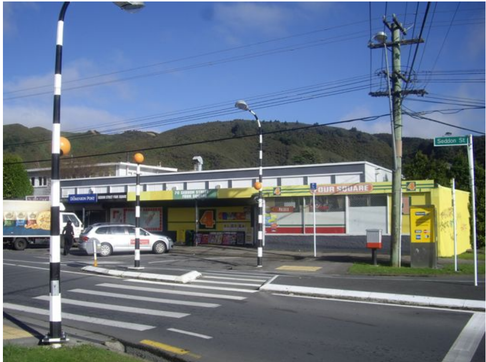
Figure 17: Seddon Street shops (Source: Ben Schrader)
