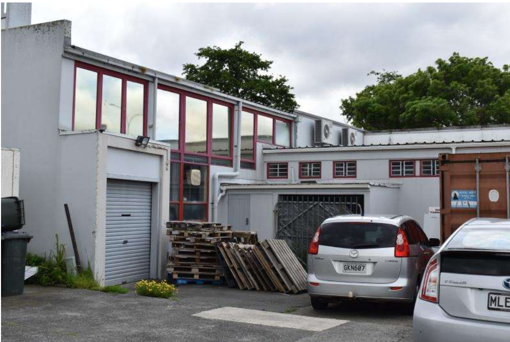
Figure 20: the rear of the building showing the mail dock (indicated by the roller door) and bicycle storage room (small lean-to with the large gate behind the stacked pallets).
