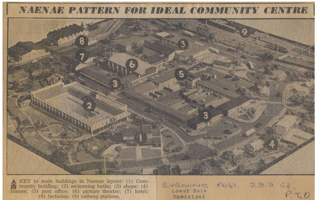
Figure 8: Model of Naenae community centre, 1953, as published in the Evening Post (Source: Hutt Valley Heritage Centre, Petone)
