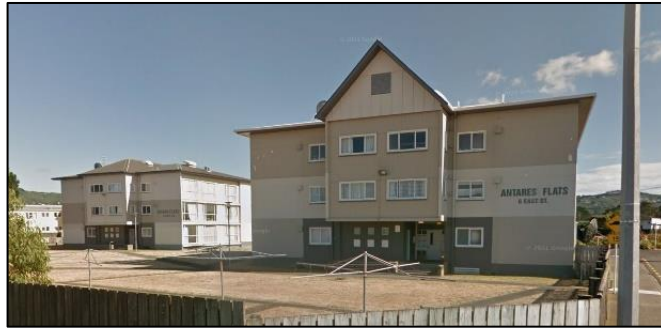
Fig. 16 Remodelled Star flats at 82 Adelaide Street.
