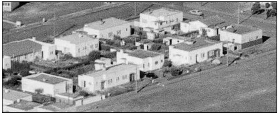
Fig. 10 Single dwellings and duplexes as constructed at 81–91 Adelaide Street
