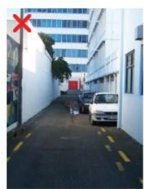
Rearlane is too narrow to allow for parking on one side. It obstructs trucks movement
