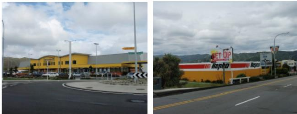
Existing character - large surface of car parking fronting the streets; bulky buildings; large signage; poorly landscaped; and dominating colours
