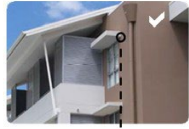
Eaves and moveable vertical shading device (external venetian blind) on east or west facing windows.
