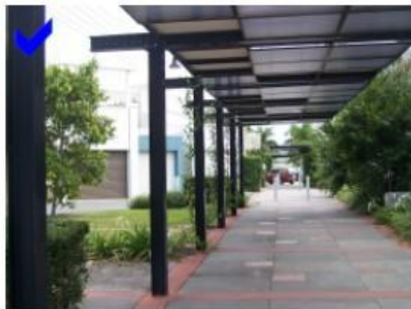
Covered walkways that allow for planting to grow up and over the structure
