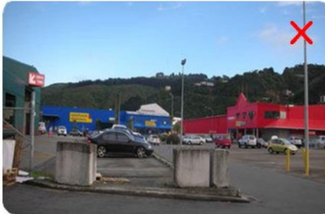
The sites in the western-most area of Petone are large and surface parking predominates. The subdivision of these sites over time to provide new streets, open space and increased intensity of use is intended.
