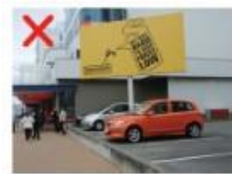
Signage not related to the building
