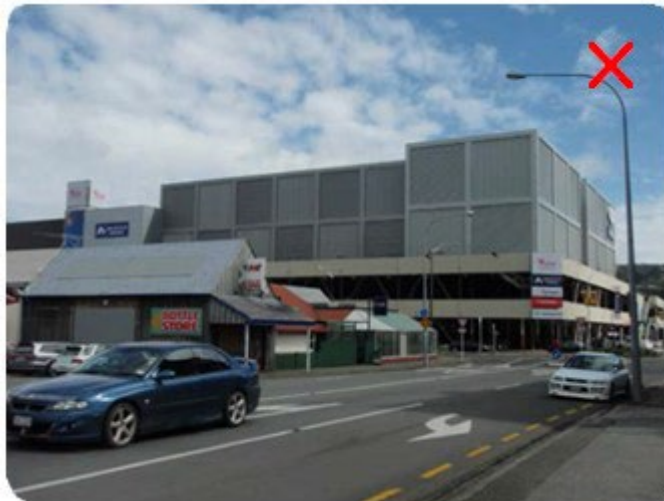
Car parking structure dominates the streetscape; inactive street edge and elongated blank walls.
