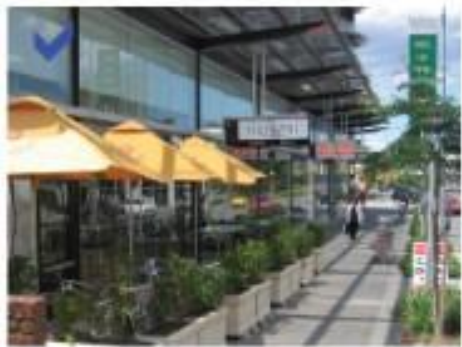
Signage attached to the verandahs
