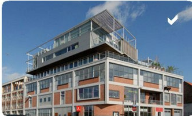
Building with an addition on top that is higher at the corner.
