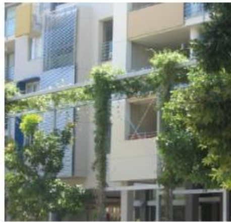
Green structure as part of the facade
