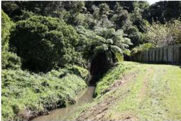
Image 3: Existing Waiwhetū Stream at end of Balgownie Grove
