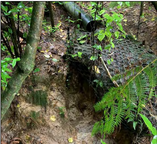
Figure 59: Stormwater discharge during no flow.
