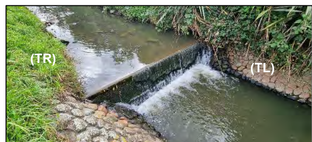
Figure 54: Weir located downstream of site.
