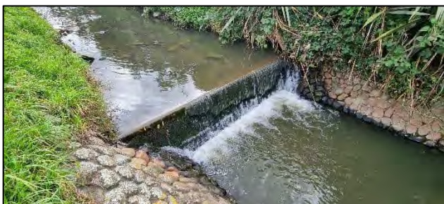
Figure 82: Weir downstream of site within Waiwhetū Stream
