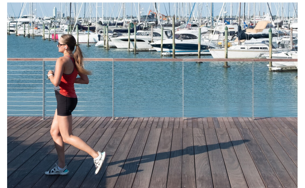
Figure 1.28 Example of a coastal balustrade with timber top rail and wire lines to reduce visual impact. Ref; Westhaven Promenade, Auckland. By Landlab.
