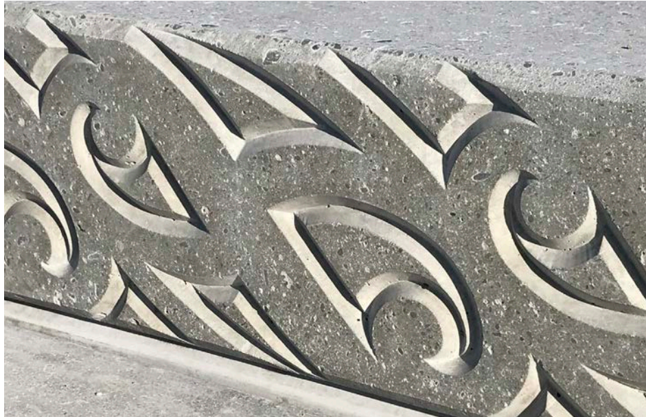
Figure 1.31 Example of a concrete texture incorporating cultural expression that could be used on a seawall design.
