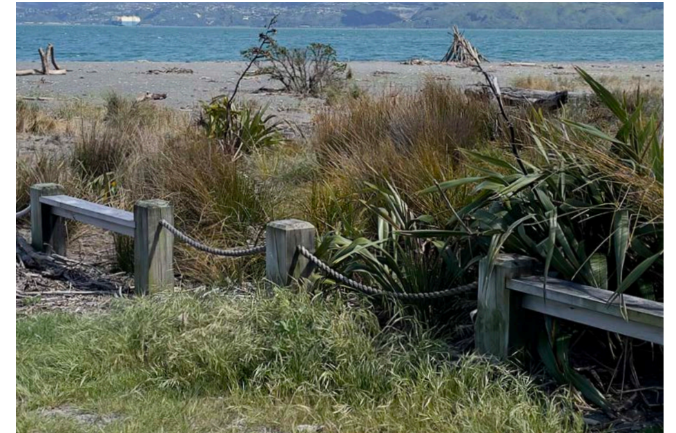
Figure 1.21 Example of rope fencing to bird habitat areas to minimise pedestrian movement
