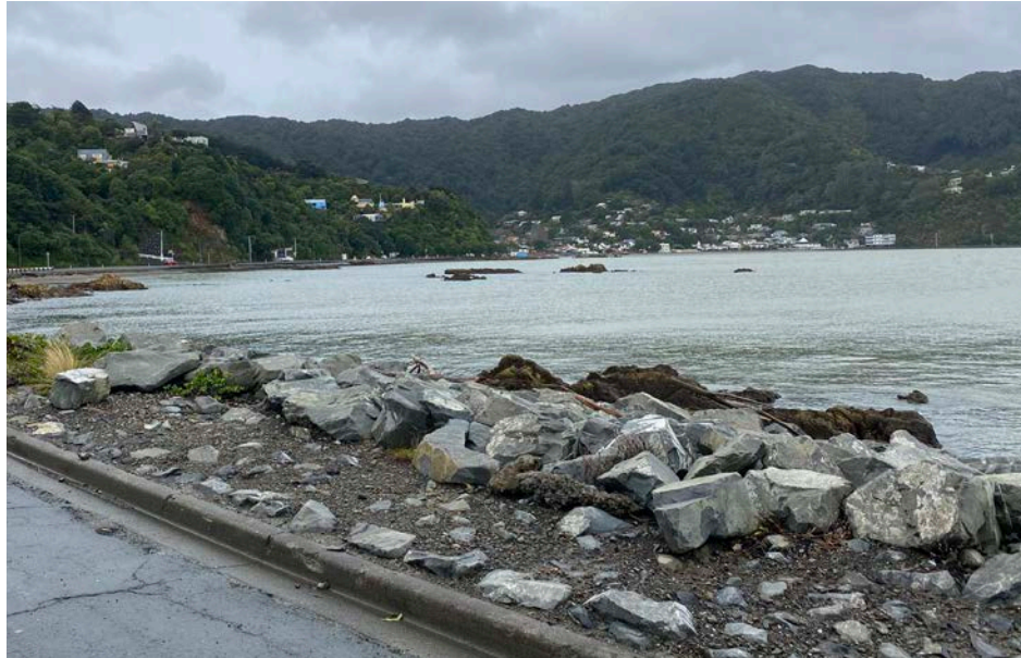
Figure 1.12 Point Howard/ Ngau Matau Revetment
