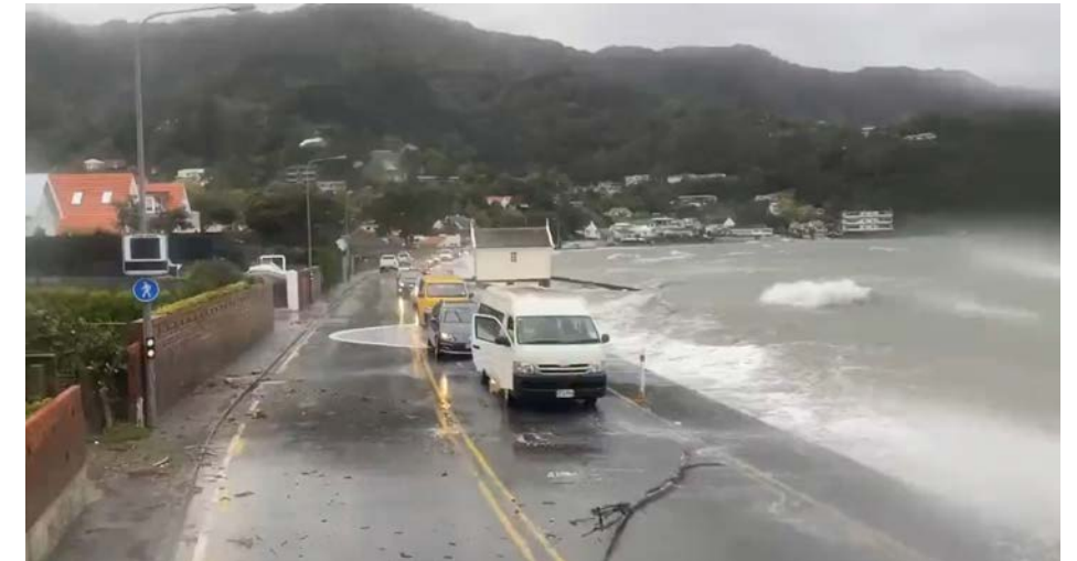
Figure 1.6 Recent storm event showing debris across road and waves lapping the road
