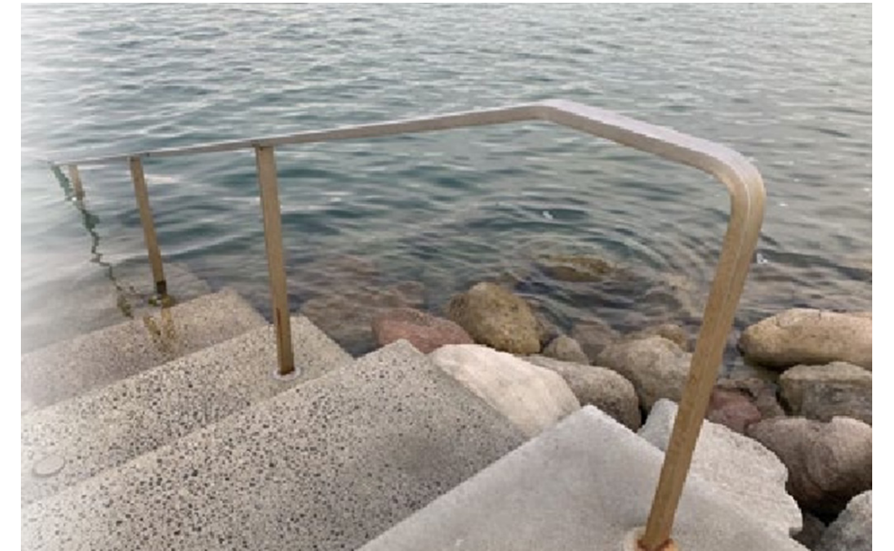
Figure 1.29 Example of a handrail for steps into a coastal environment. Ref; Stantec
