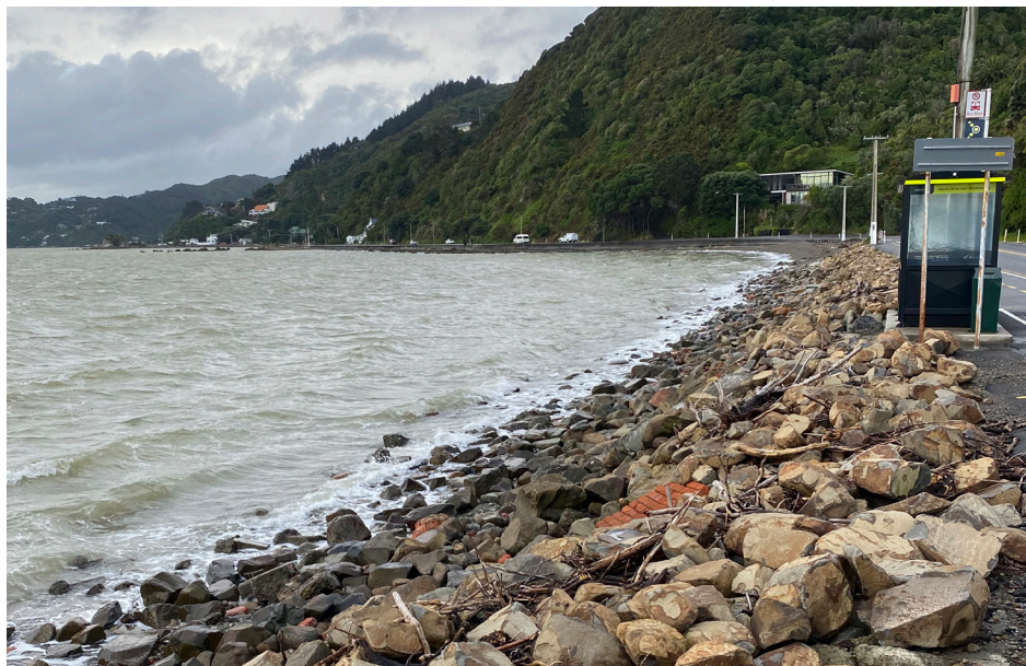
Figure 1.14 Sunshine Bay Revetment
