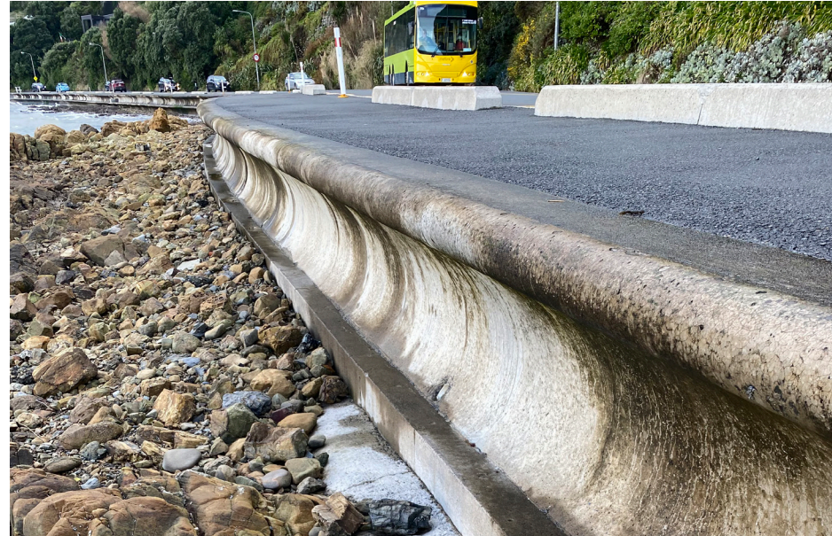
Figure 1.13 York Bay Seawall
