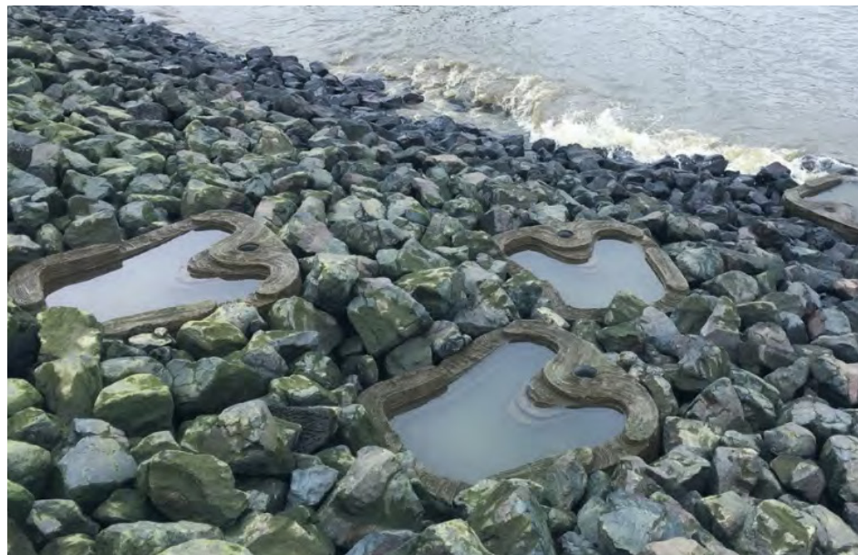
Figure 1.30 Tide pools installed in rock revetment. Ref SHRP
