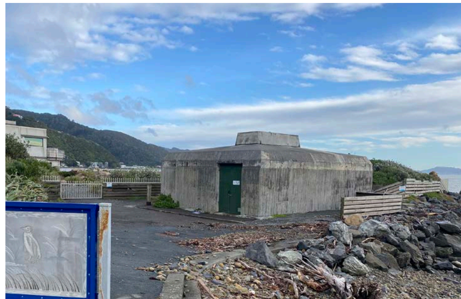
Figure 1.15 Pump Station at Sunshine Bay/ Days Bay
