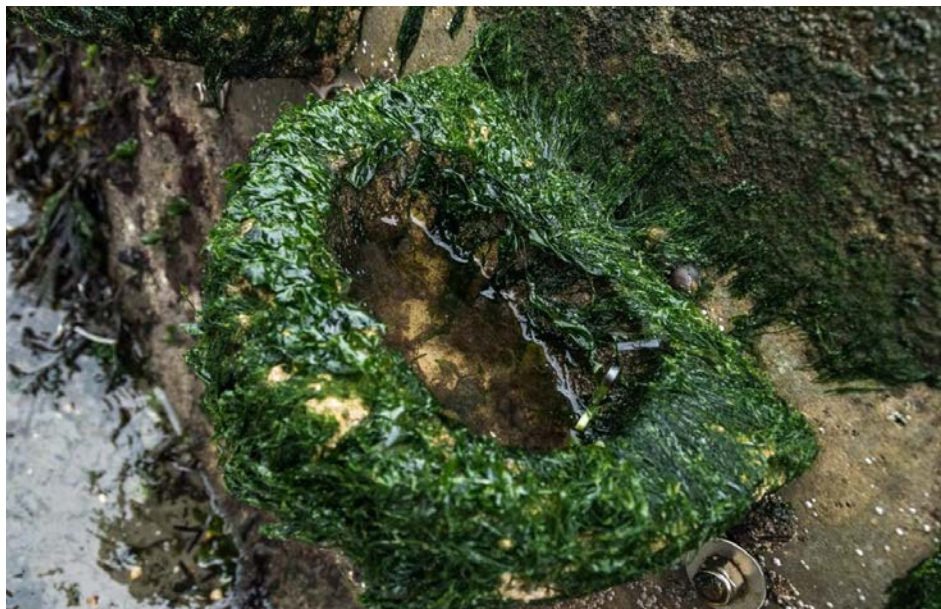
Figure 1.32 Artecology 'Sandown' Vertipool installed on a seawall. Ref SHRP
