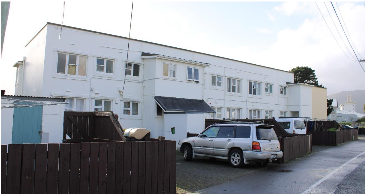
Figure 1: The two-storey flats at 2-6 East Street, Petone.
