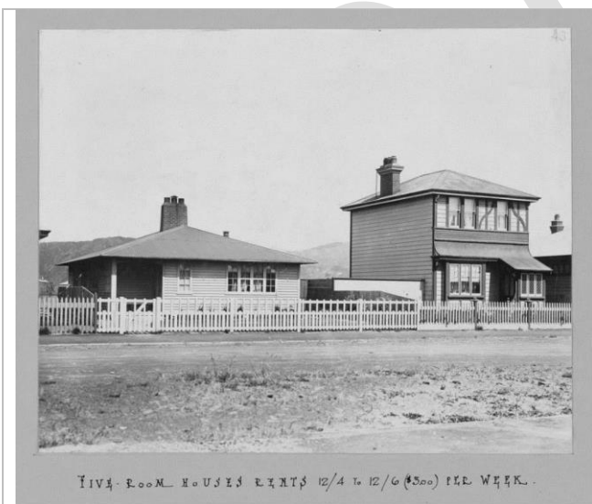
Figure 6: 4 (left) and 6 (right) Patrick Street – built in 1906 as part of the Heretaunga Settlement scheme. Source: Harvard Art Museums
