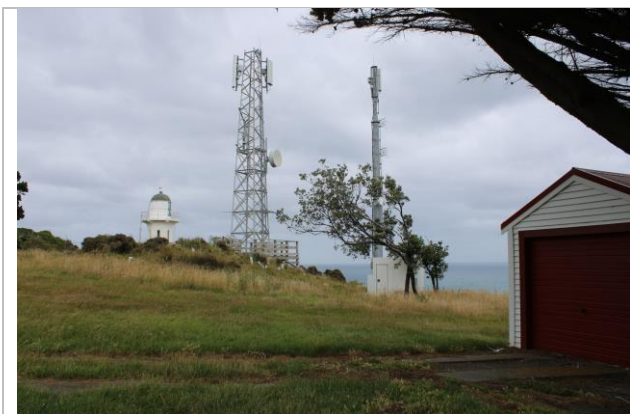
Figure 14: Radio mast and cellphone towers on the site.
