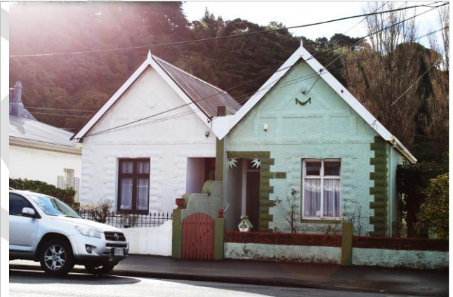
Figure 6: Semi-detached building on Riddlers Crescent.
