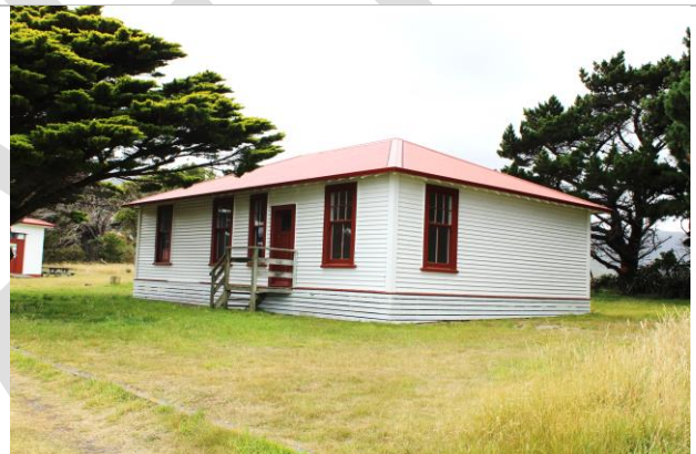
Figure 11: One of the 'keepers cottages, restored by the Friends of Baring Head conservation group.
