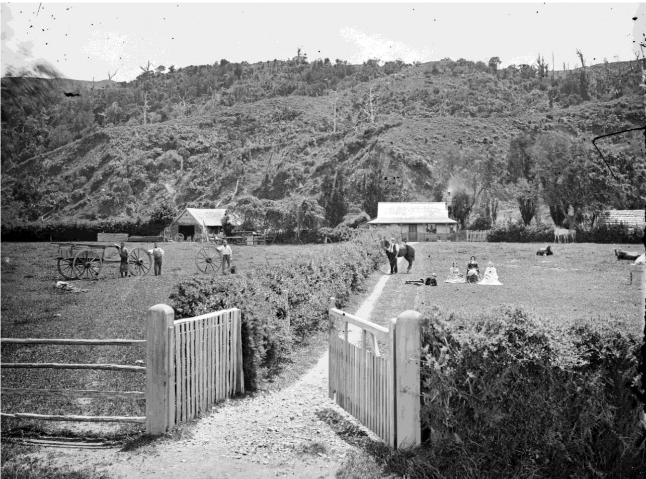
Figure 1: Collett's Farm, later to become Riddlers Crescent, with HNZPT Category I Collet House pictured, 1874. Source: Te Papa Archives, ID: D.000029
