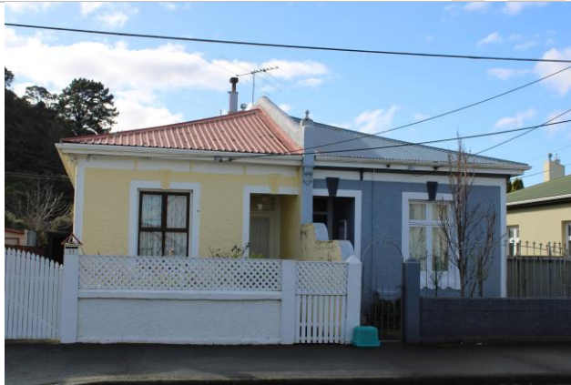
Figure 5: Semi-detached building on Riddlers Crescent.
