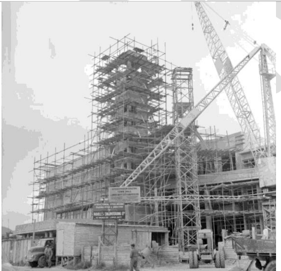
Figure 11: The buildings under construction, 1956. Source: ATL, ID: EP/1956/0335-F
