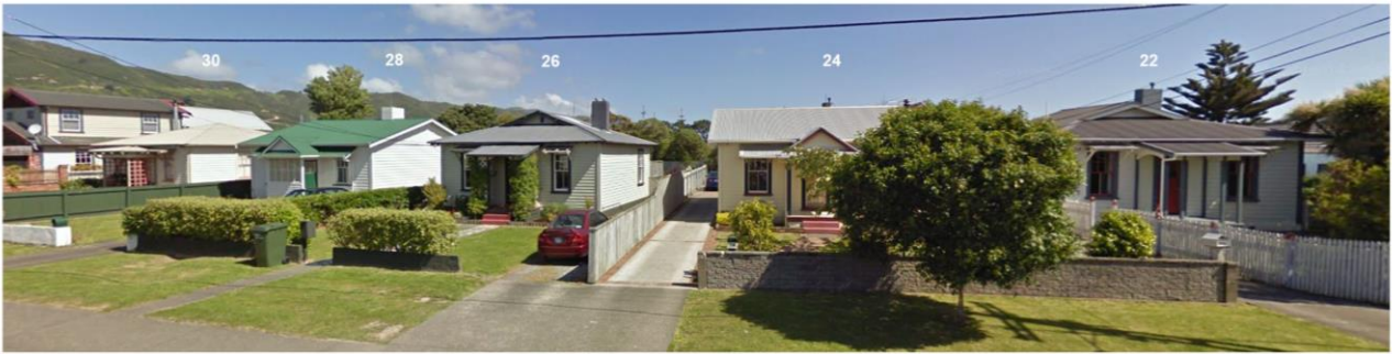
Figure 7: Panoramic street capture showing the buildings which comprise the Elizabeth Street section of the Moera Railways Heritage Area.
