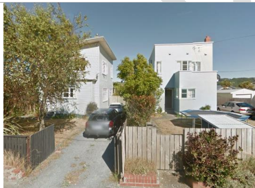
Figure 8: Flats on Adelaide Street.
