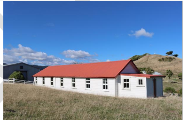
Figure 7: The barracks building in 2021, hastily erected in 1919 in preparation for the expected casualties of the influenza pandemic after WWI and used during WWII for POW's.
