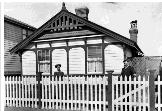
Figure 8: 2 Patrick Street, built in 1906 as part of the Heretaunga Settlement scheme, photographed in 1908. Source: ATL, ID: PA1-O-195-20-2
