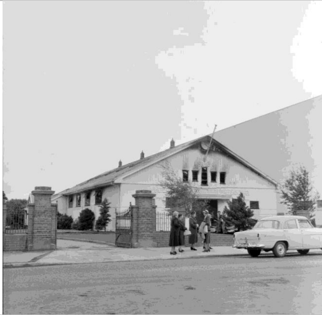
Figure 15: The original Horticultural Hall prior to fire damage, photographed in 1957. Source: ATL, ID:
