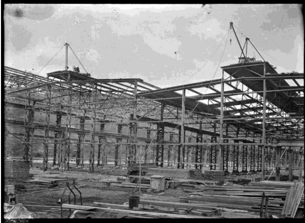
Figure 3: The Hutt Railway Workshops under construction in 1928.
