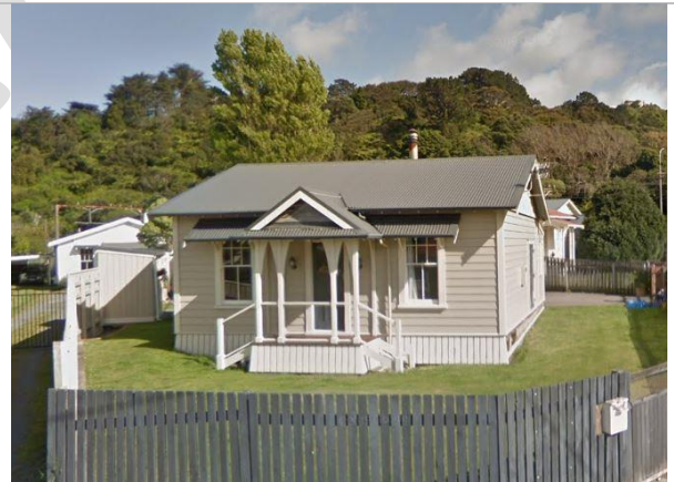
Figure 6: 107 Railway Cottage on Hutt Road.
