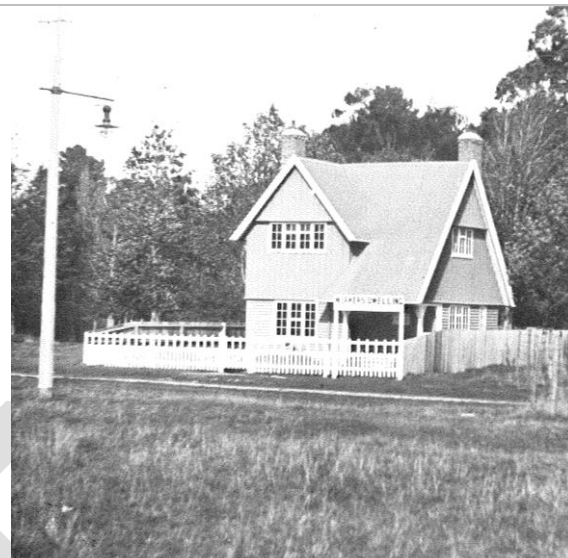
Figure 5: Full-scale 'Workers Dwelling' built for the International Exhibition at Christchurch held between November 1906 and April 1907, designed by Samuel Hurst Seager and Cecil Wood. Source: HNZPT 1984 Booklet
