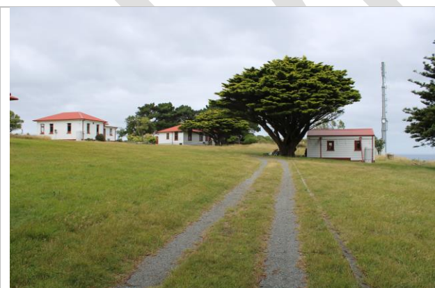
Figure 12: The original road leading towards the collection of buildings.
