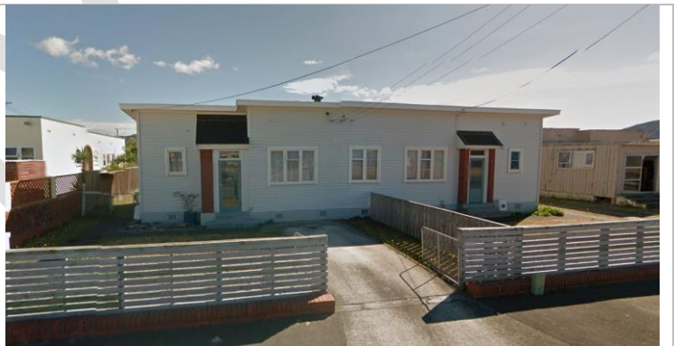
Figure 9: Flats on Adelaide Street.
