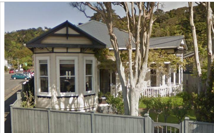
Figure 7: 101 Villa on Hutt Road
