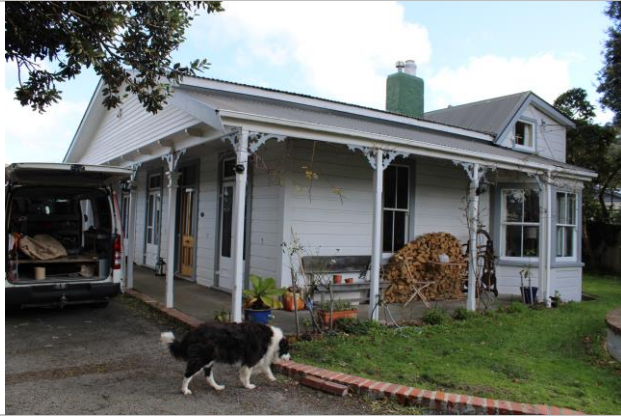
Figure 9: Collett House on Riddlers Crescent.
