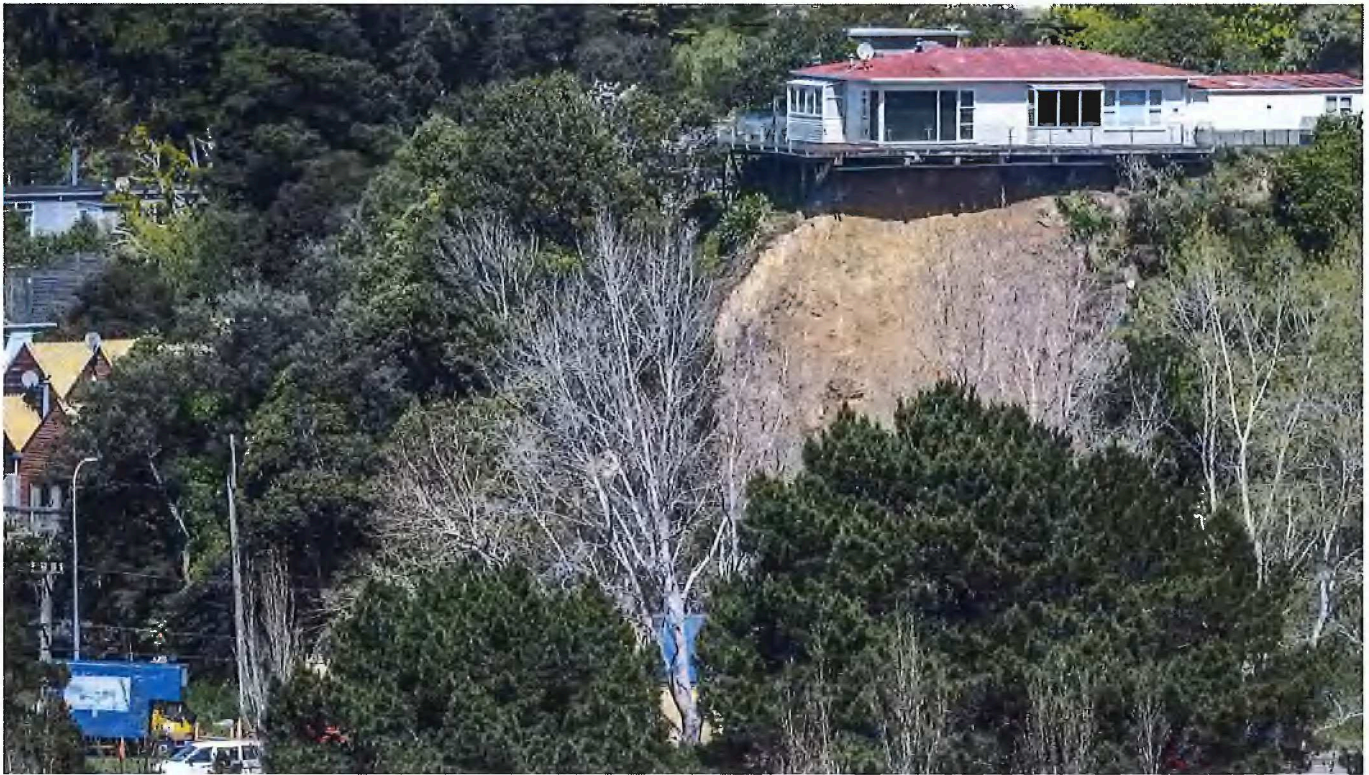
Stokes Valley slip on Council land (house has since been demolished 2023)
