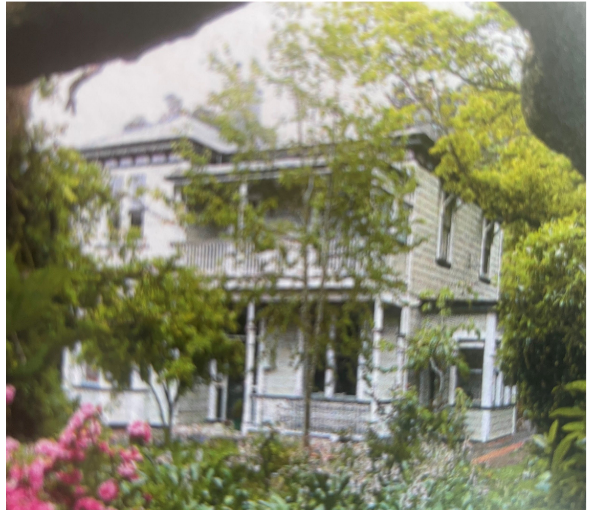
2 Bridge St, Melling Not included in the proposed heritage areas
