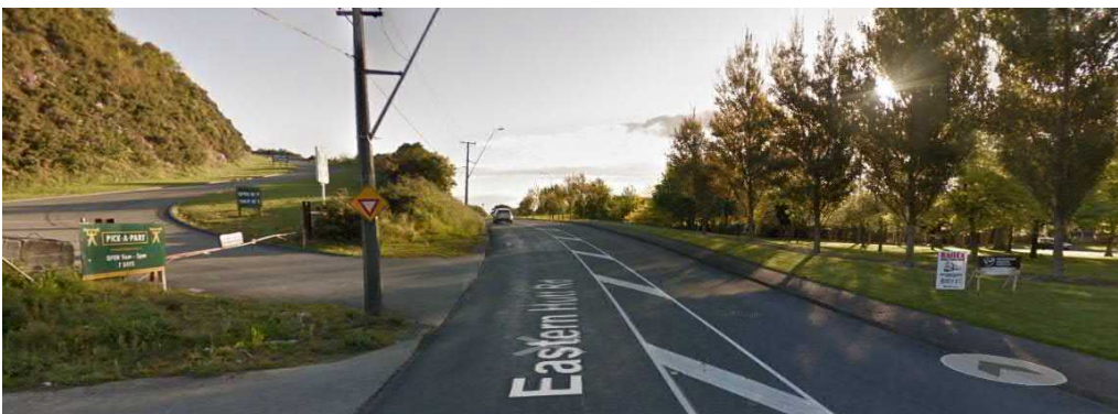
Figure 21 - Existing entranceway to Pick a Part site
