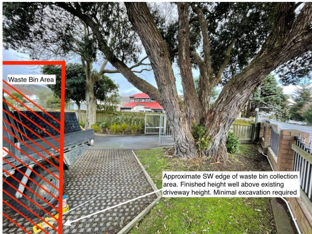
Appendix 21: Attached approximate edges and finished height of waste bin collection area
