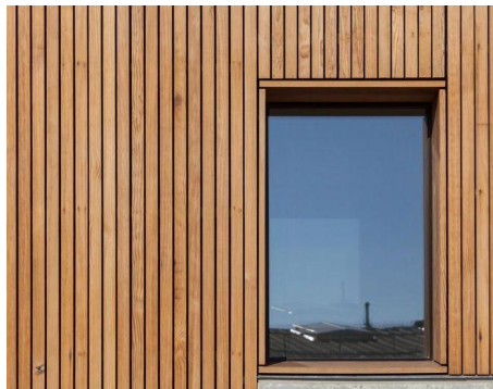
Figure 31: Timber Wall Cladding
