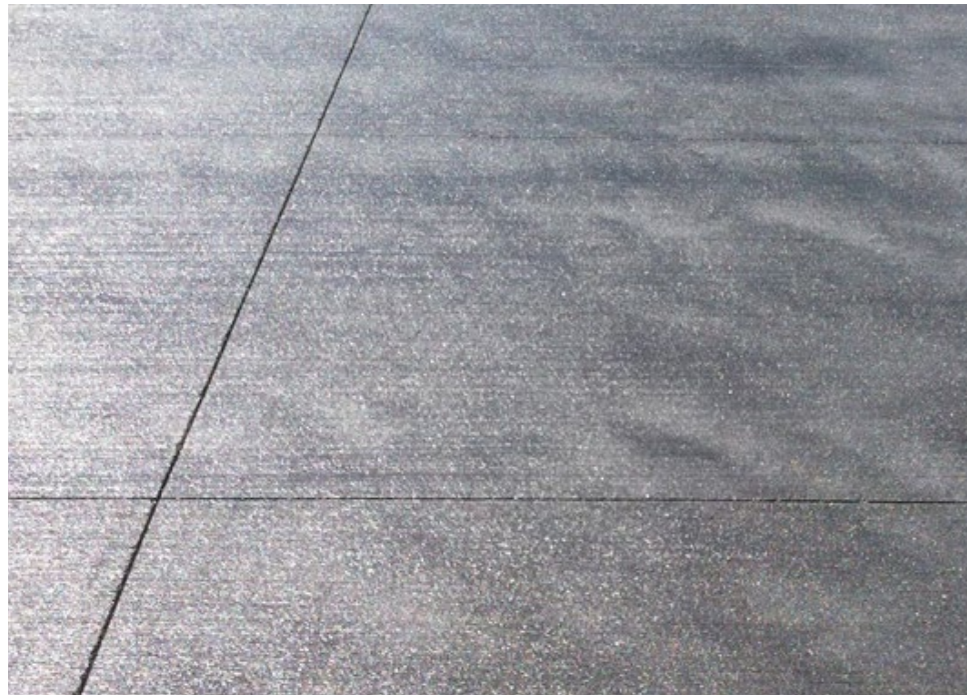
(A) Brushed concrete - U5/U6 Deep textured wire broom finish - 3% black oxide
