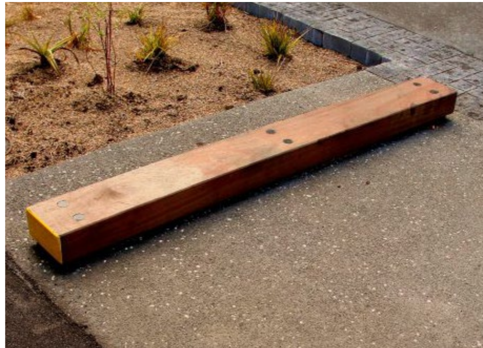
Wheel stops - 1800L x 200W x 125Dmm Hard wood timber wheel stop bolted to ground with parking number attached, or similar approved
