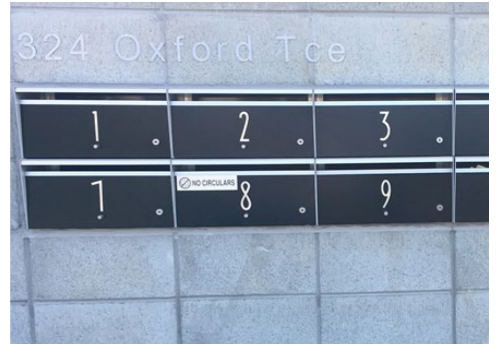
Letterboxes - Lockable wall-mounted letterbox set - colour black or silver with large numerals placed on each letterbox, Letterboxes to be grouped in the cafe area
