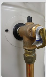
TPR position - top of cylinder
