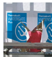
On arrival of doors and windows, cut Watergate at each opening on a 45° angle away from each corner. Pull the Watergate flaps inside and fasten to the inside of frame.
