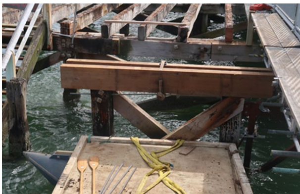
6. New capping beam and stringer beams installed
