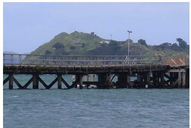
Figure 5: Ramping of final bents on approach
