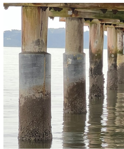
Figure 10: Piles with FRP jackets at Petone Wharf
