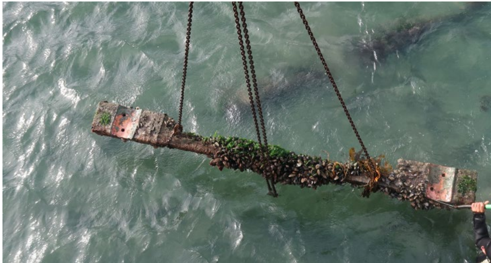
3. Bracing & walers inspected and removed if in poor condition
