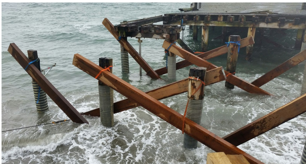
5. Bracing & walers replaced if needed
