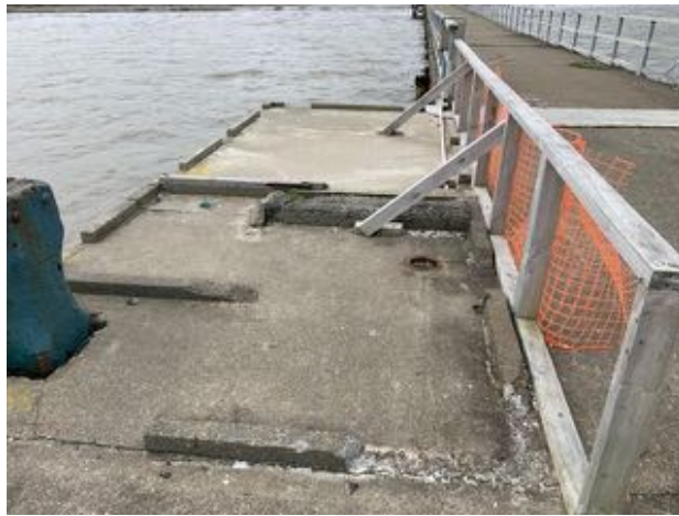
Figure 42. Remaining foundations on the wharf head. Source: Calibre Consulting Ltd.
