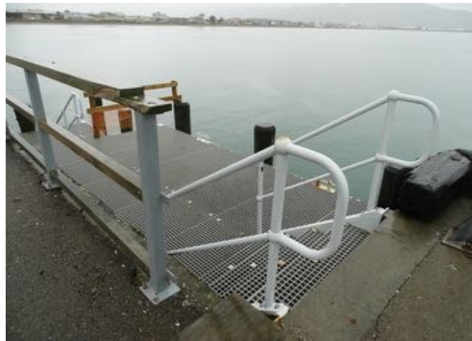
Figure 90. The current steel mesh access platform
