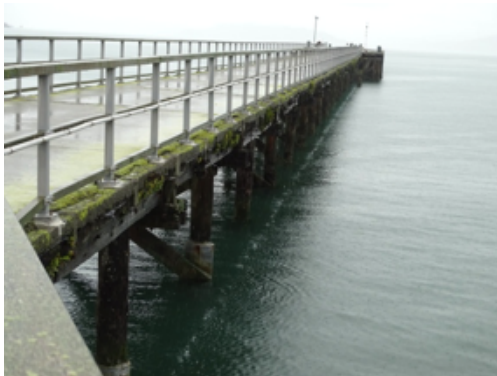
Figure 33. The structure below the approach as seen from the cart refuge
