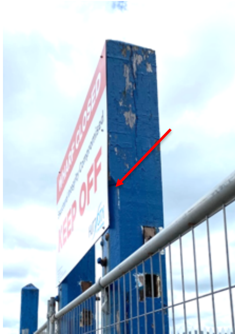
Figure 53. Possible original central post, note stop chamfer detail.
