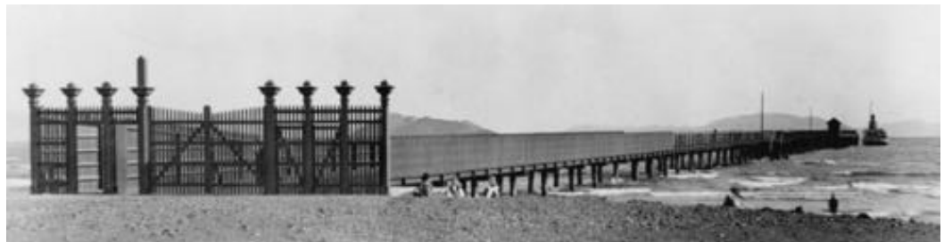
Figure 55. The Petone Wharf, 1909, showing the original entrance gates and side fence down the wharf. Source: ATL 1/2-002541-F
