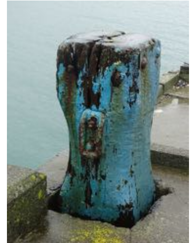
Figure 41. An original timber bollard on the head
