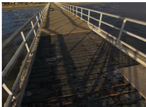
Figure 67. Test portion of concrete decking removed showing original decking, 2018. Source: Google Street View, December 2021
