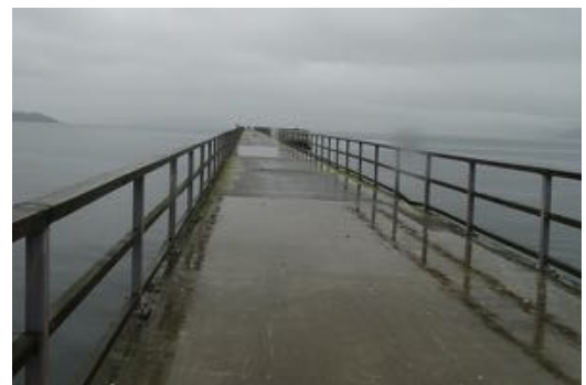
Figure 68. Concrete and asphalt decking on the approach of the wharf, 2021
