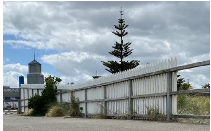
Figure 60. The current fence as viewed from on the wharf. Note the palings decrease in height from The Esplanade in the first few bays.
