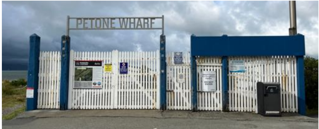
Figure 51. The Petone Wharf entrance in November 2021. Source: Calibre Consulting Ltd.
