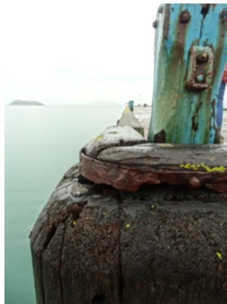
Figure 96. Existing timber corner fender and metal kerbing on the head.
