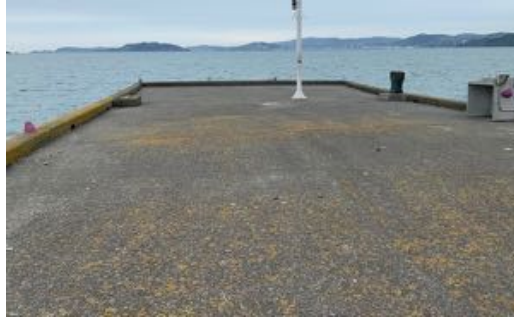
Figure 69. The concrete decking on the wharf head. Source: Calibre Consulting Ltd.
