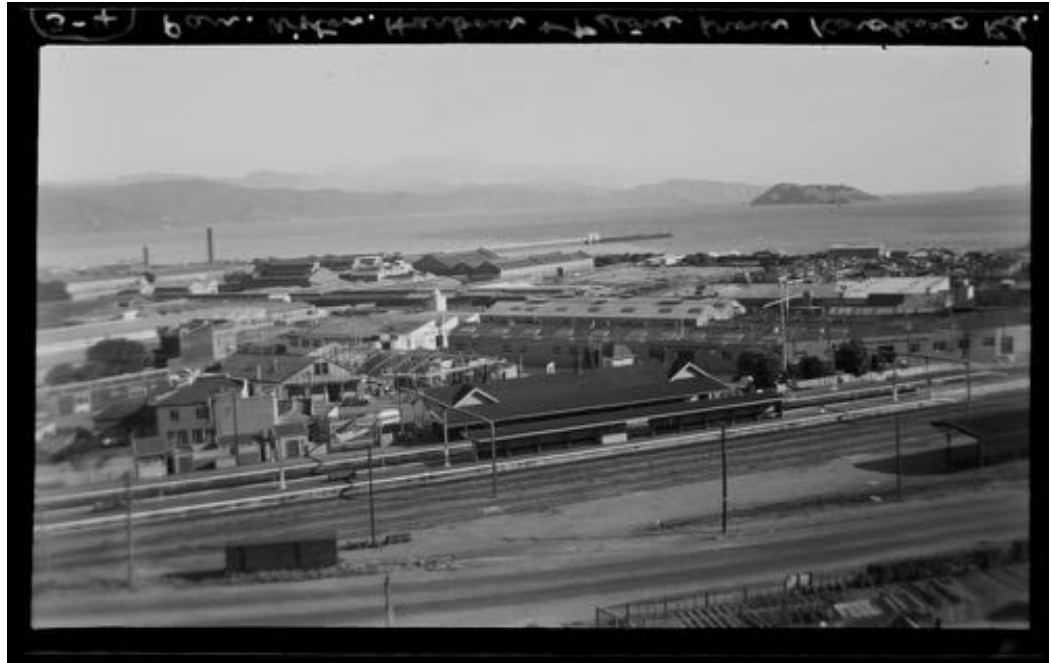
Figure 22. View over Petone with the Petone Wharf in the background, 1954. Source: Te Papa A.007780
