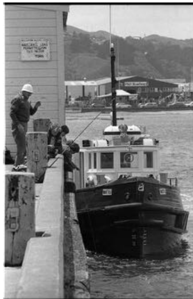
Figure 82. The Petone Wharf, 1982, showing the eastern modified office buildings. Source: ATL EP/1982/0270/30A
