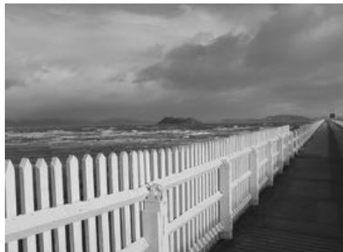
Figure 57. The Petone Wharf 2002 with the balustrade original structure. Note the arris rails. Source: Whaka, "Storm Wellington Harbour", 2002, Photograph. Accessed 09-11-2021 https://commons.wikimedia.org/wiki/File:Storm_Wellington_Harbour.JPG?fbclid=IwAR0KGchDL-7VH9s-ucMYzhx5WAizfXo5Jlg1dxJDe_n3NjIOHmcR9Bzbe94
