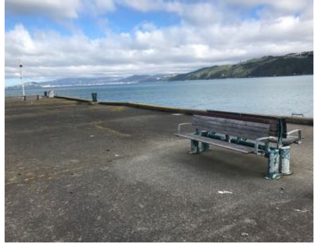
Figure 92. The bench seats on the wharf head, 2017. Source: Calibre Consulting Ltd.
