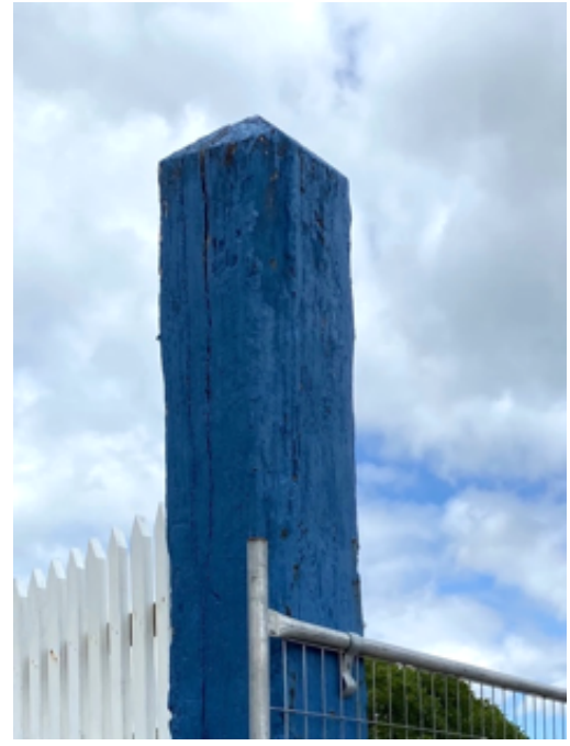
Figure 54. Likely non-original outer post, note rough timber
