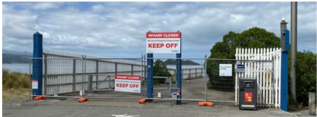
Figure 52. The Petone Wharf entrance, January 2022, with gates, fencing, and two posts removed
