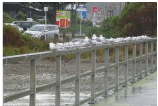
Figure 64. Current metal and timber balustrade, 2021
