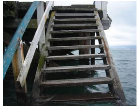
Figure 75. The stairs from the cart refuge, 2009. Source: Calibre Consulting Ltd., 2009
