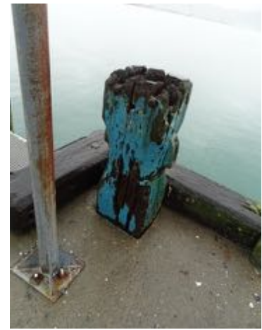
Figure 43. Timber kerbing at the north-east corner of the head
