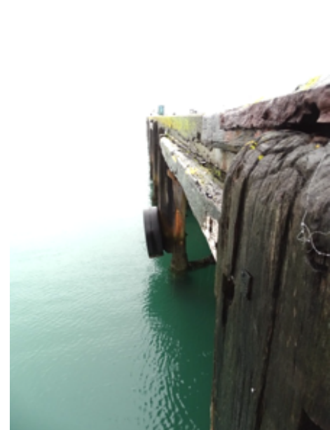
Figure 97. Existing timber fender on the head.
