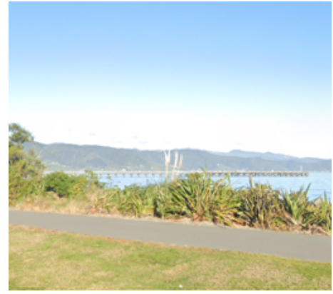
Figure 25. View of Petone Wharf from The Esplanade, approach from the west. Source: Google Street View, December 2021, accessed November 2021
