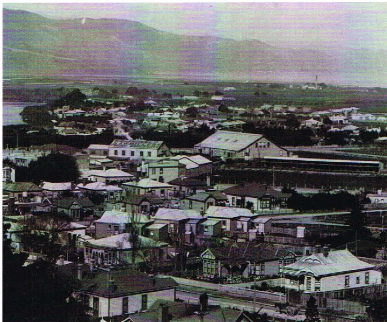
Photo 5. Alicetown Drill Shed photographed from approximately above the Hutt Railway Station, (now called Western Hutt Station), circa 1910.
