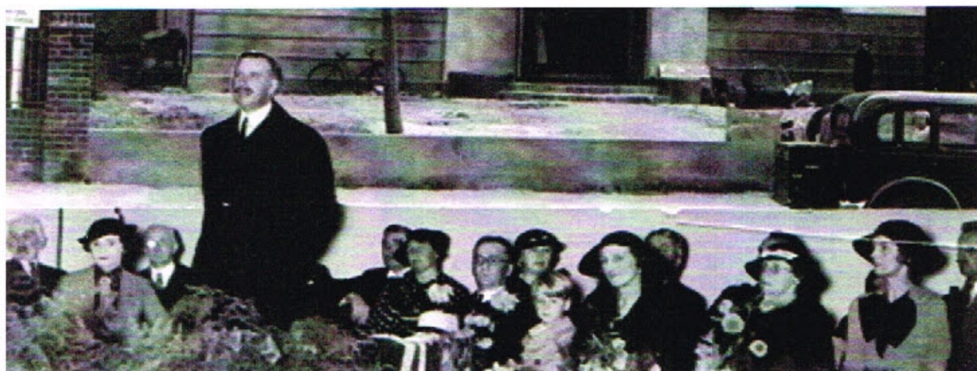
Photo 14. The Governor, Lord Galway, opening our old Hall in September 1936. This image is part of an Evening Post montage along with Photo A, on page 1.
