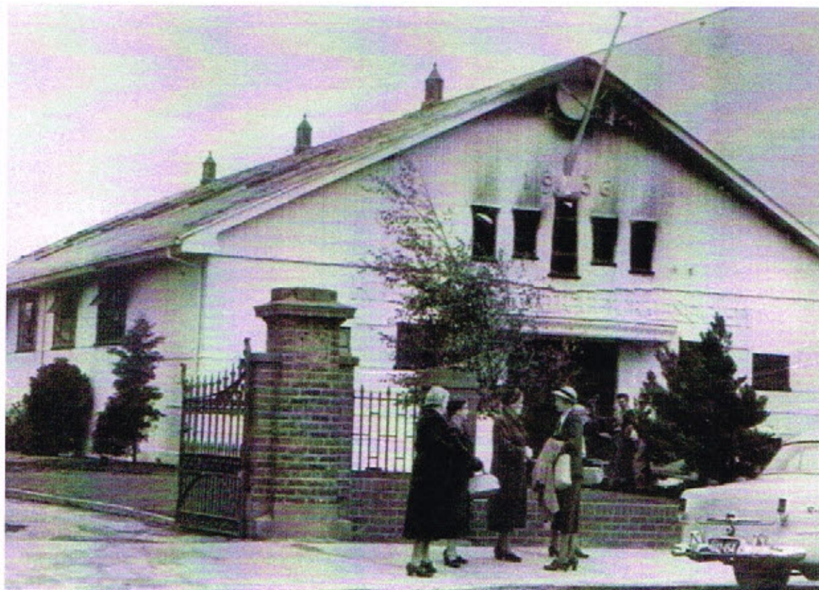
Photo 12. The Hall exterior the morning of the fire.
