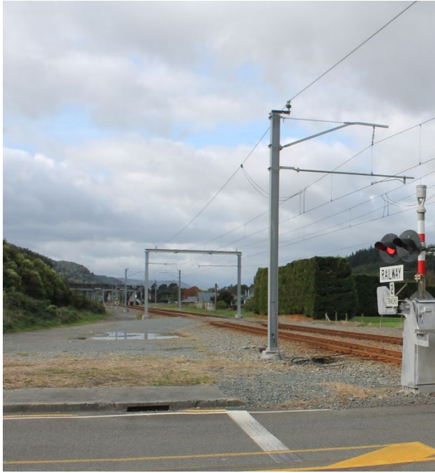
Figure 3-15: West Carriageway Approach Uptrack Sightline
