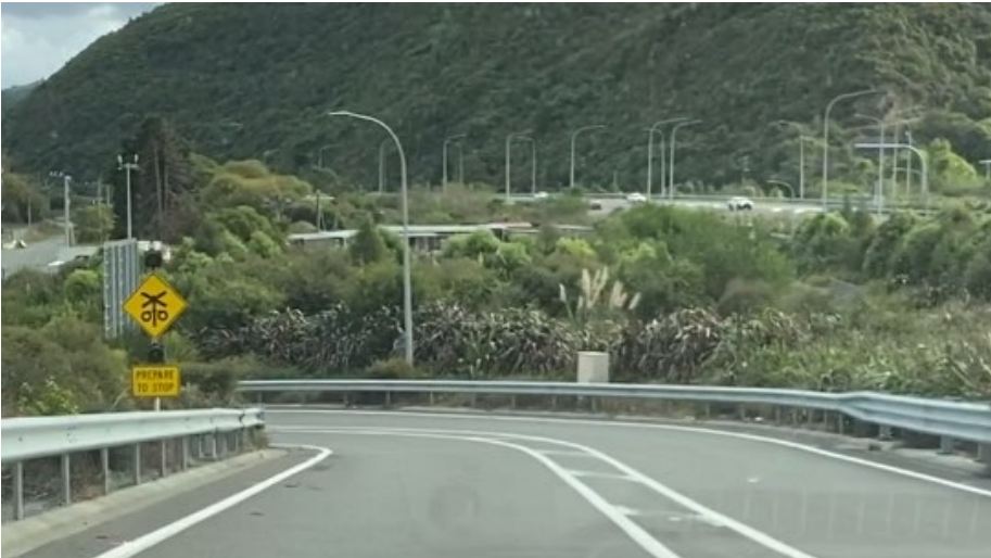
Figure 3-7: Active Warning Signage on Western Approach
