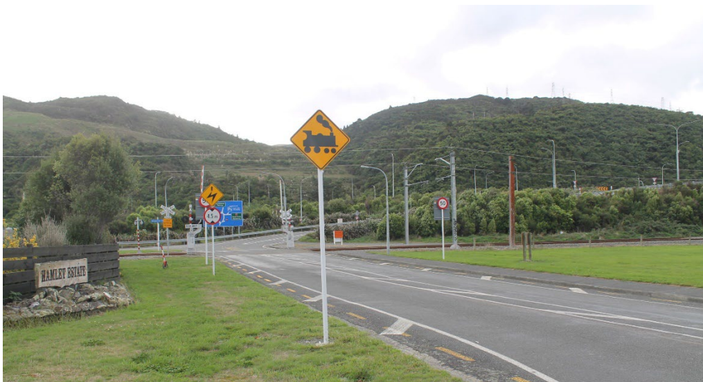
Figure 3-3: Manor Park Level Crossing View From East
