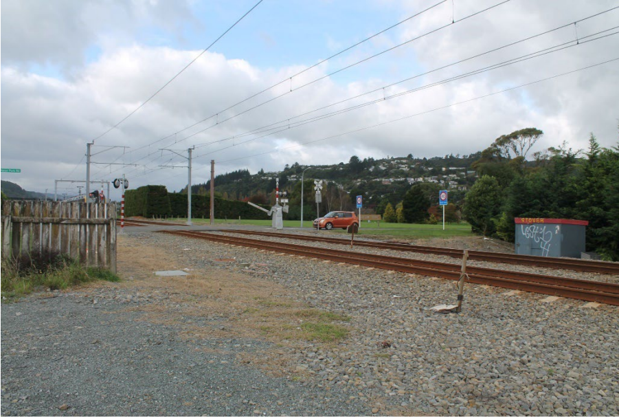
Figure 3-12: Benmore Crescent, Showing Lack of Rail Corridor Fencing
