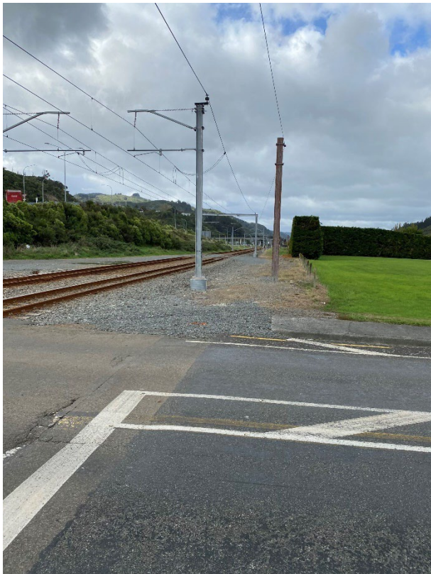
Figure 3-13: East Carriageway Approach Uptrack Sightline, also Showing Footpath Stopping Short of Rail Corridor
