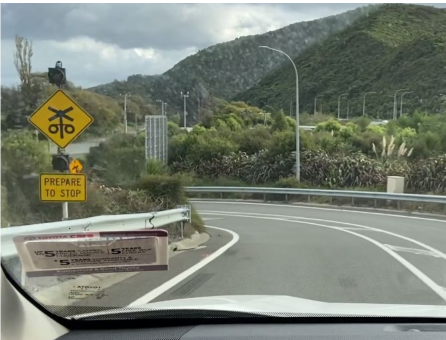
Figure 3-8: Curved Approach Limiting Forward Visibility of Crossing
