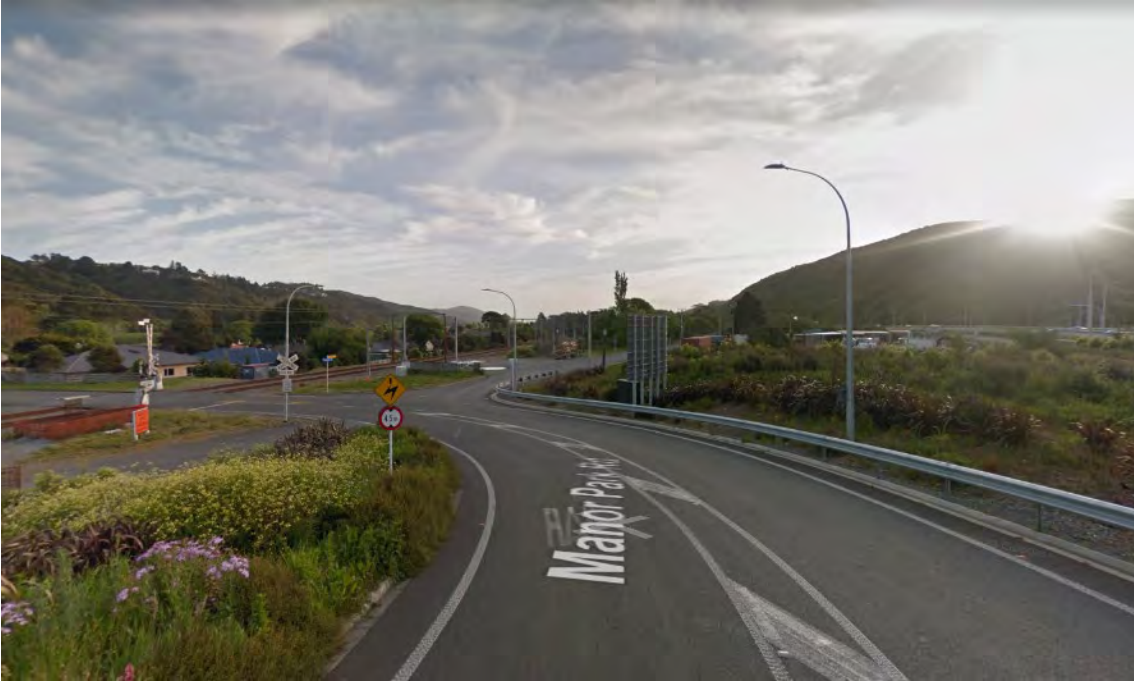
Figure 2-3 : View South on Manor Park Road towards Benmore Crescent Intersection (Google Earth)
