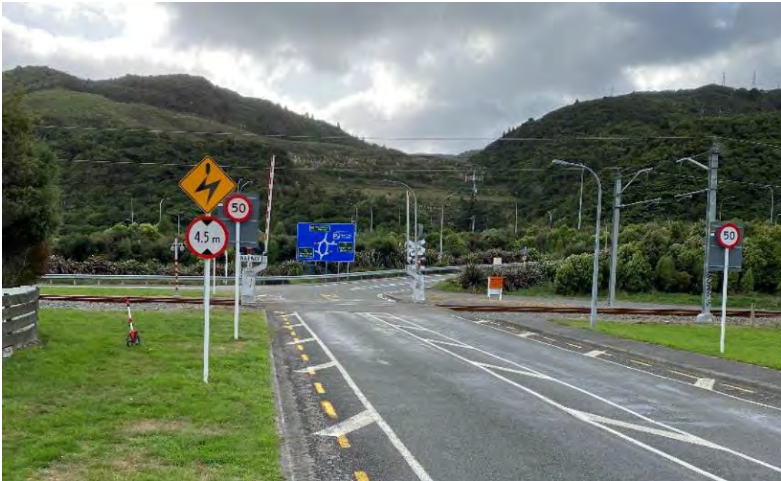
Figure 2-4 : View along Manor Park Road over the Rail Level Crossing towards the Benmore Crescent Intersection
