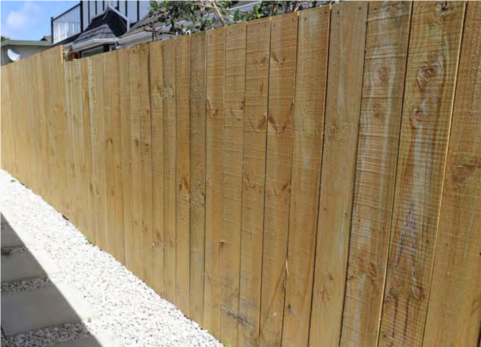
F4 - Fence 4 - 1.8m closeboard. Timber fence, 1.8m height, 150mm palings with no gaps between.
