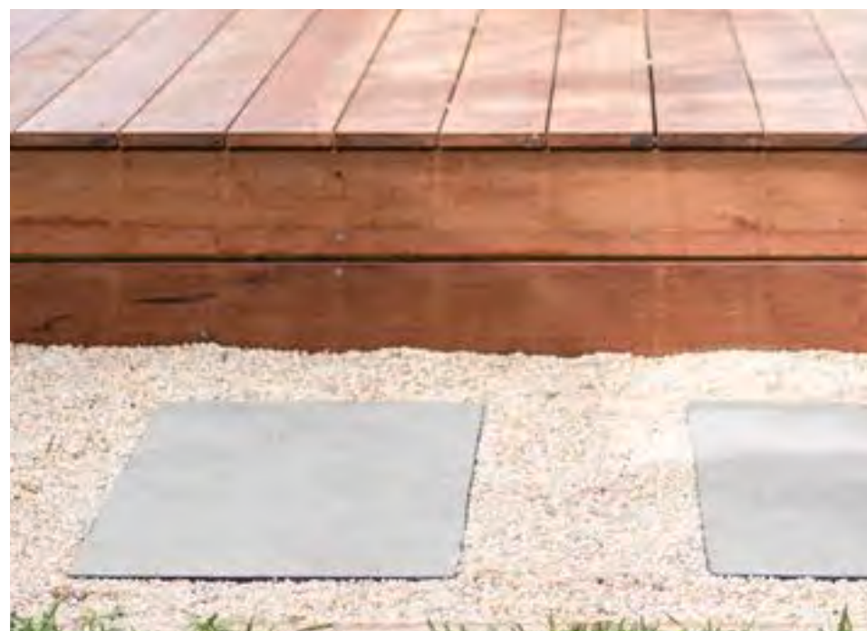
Ⓑ Surface B - Loose Pavers. Loose permeable pavers - see surface type C, set in either reinforced gravel or compacted lime chip - see surface type E so surfaces are flush.
