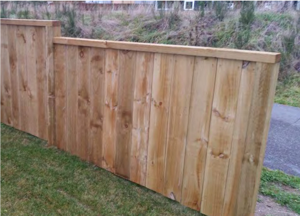
F1 - Fence 1 - 1.2m closeboard. Timber fence, 1.2m height, 150mm palings with no gaps between.
