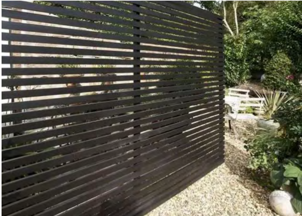
F3 - Fence 3 - 1.8m slat. Timber fence, 1.8m height, 50mm battens with 50mm gaps between.
