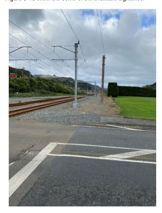
Figure 3-13: East Carriageway Approach Uptrack Sightline, also Showing Footpath Stopping Short of Rail Corridor
