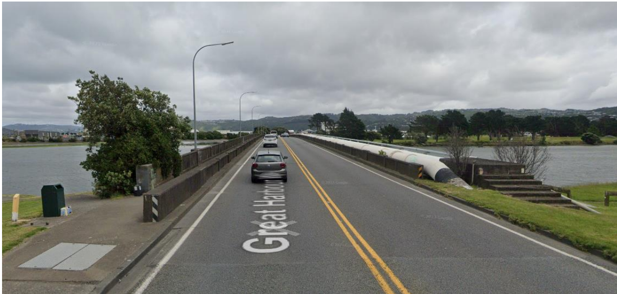
Figure 4-2: Waione Street Bridge - looking West
