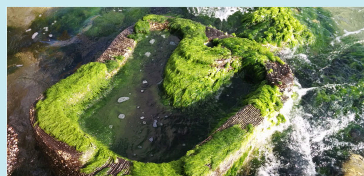
An example of a concrete tidal rockpool built into another coastal project, showing growth of plants and algae
