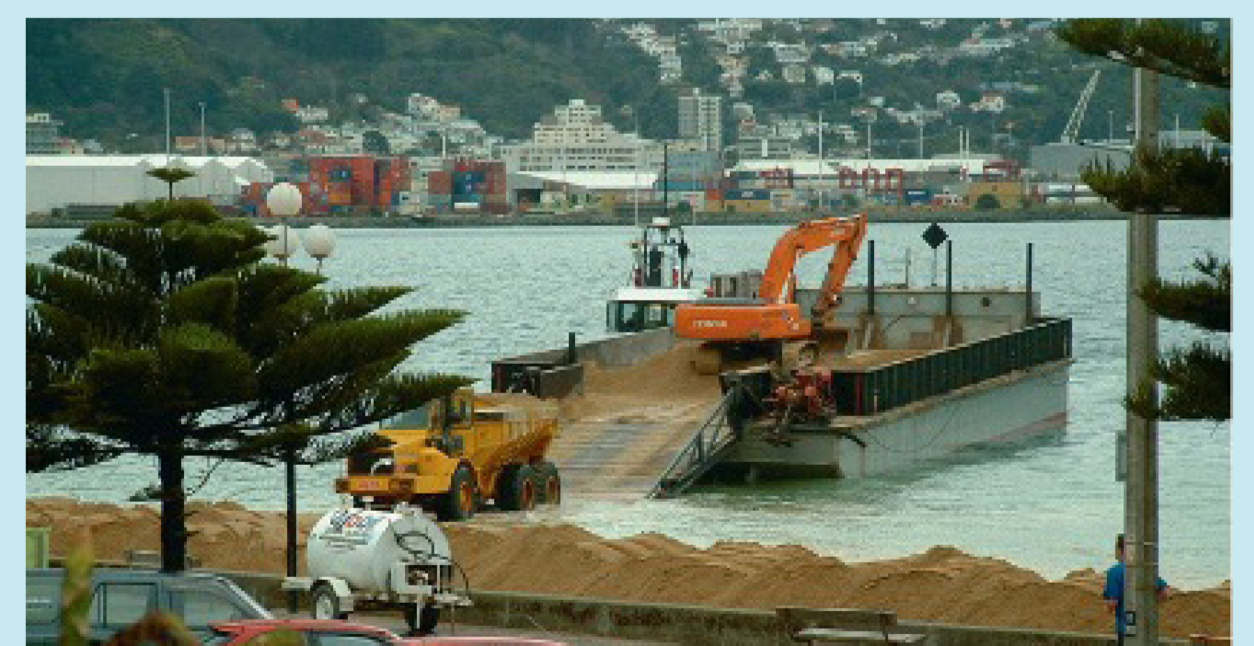
Oriental Bay is an example of a beach which has been re-nourished over several years
