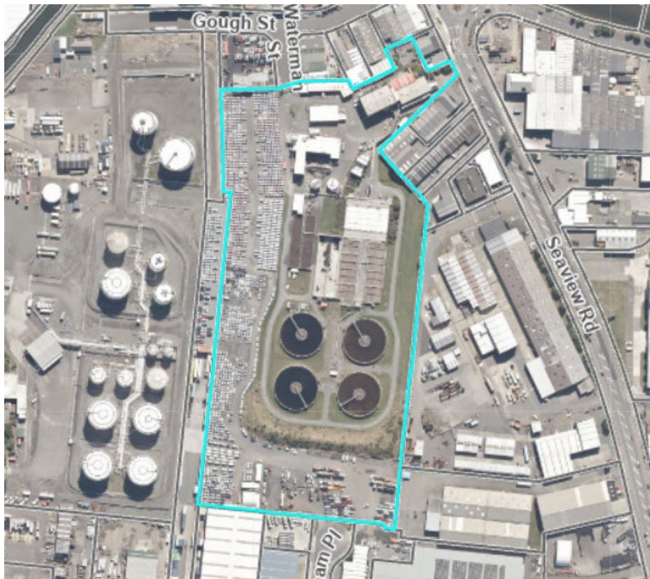
Seaview Wastewater Treatment Plant
