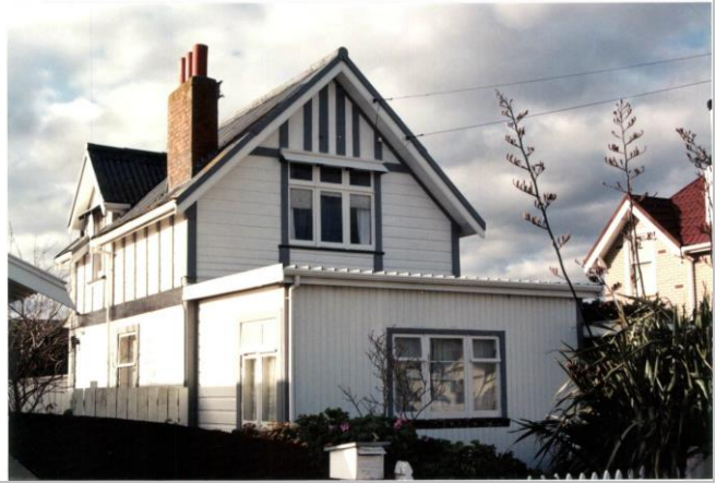
Figure 3: 43 Adelaide Street, 1994. Source: 1994 HCC Inventory
