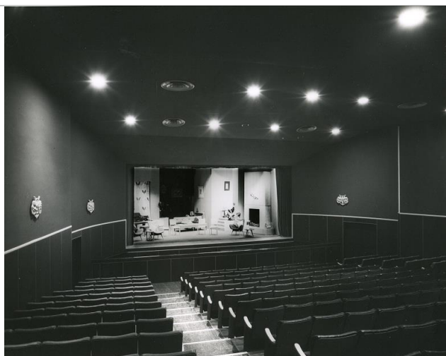
Figure 7: Interior of the theatre, undated. Source: Petone Settlers Archives
