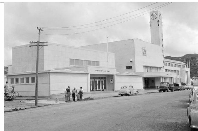
Figure 4: The completed set of civic buildings, including the Town Hall and Horticultural Hall (now demolished) in the foreground, c.1960. Source: HCC Archives
