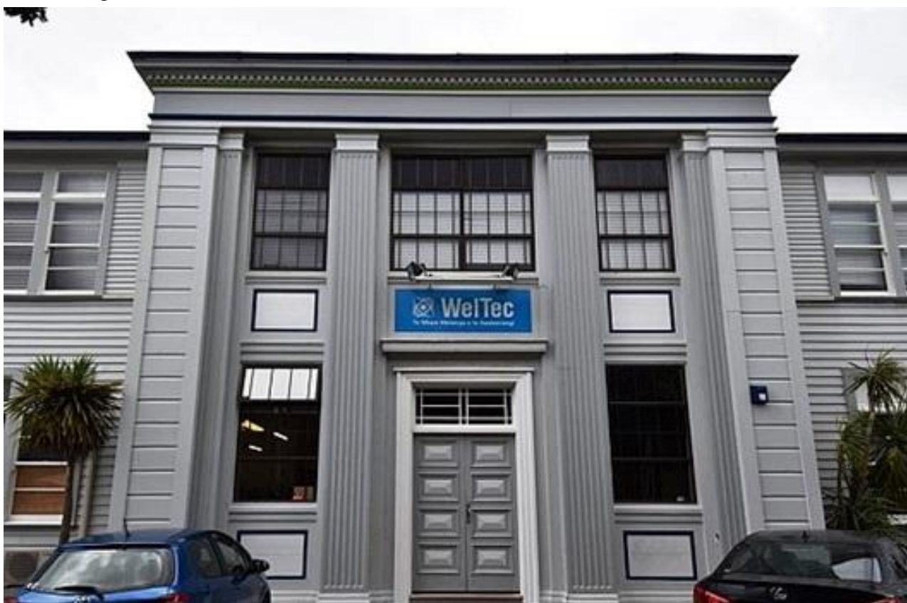
Figure 1: Former Classroom Building of the Petone Memorial College, HNZPT.
