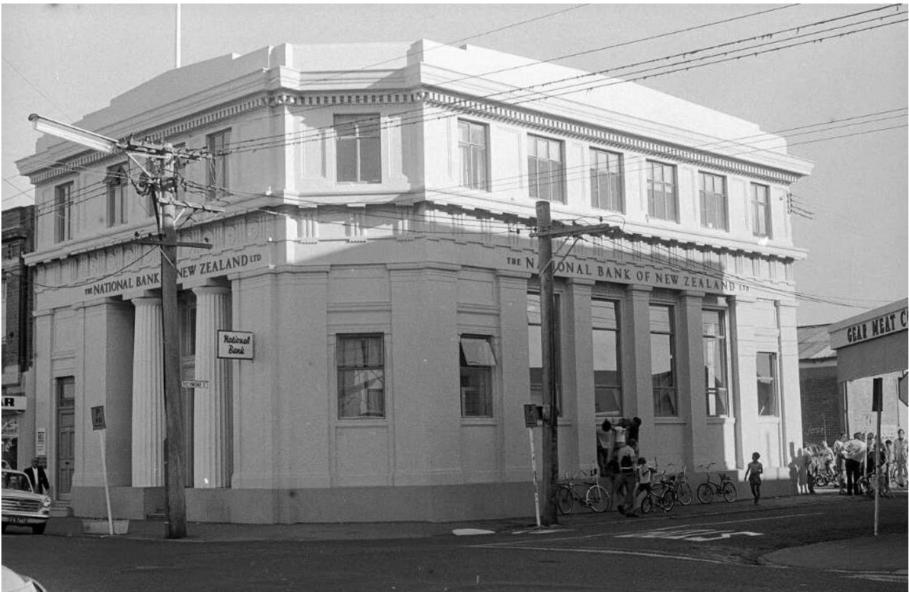
Figure 2: The National Bank Building at 226 Jackson Street, 1973. Source: ATL, ID: 1-4-021055-F
