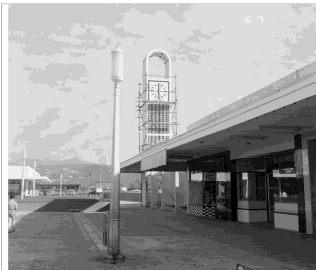
Figure 2: The post office under construction, 1959. Source: ATL, ID: PAColl-0614-1
