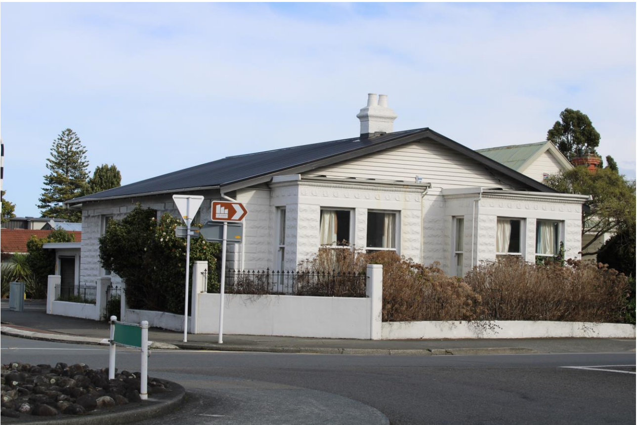
Figure 1: Offices, 64 Knights Road, Lower Hutt.
