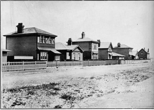
Figure 2: Some of the houses of the Heretaunga Settlement scheme photographed in 1909 (2-14 Patrick Street).
