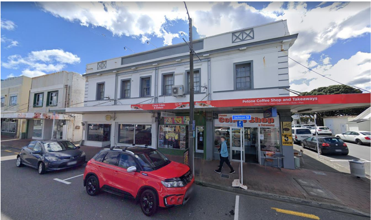
Figure 1: 257-263 Jackson Street, Petone Source: Google Streetview
