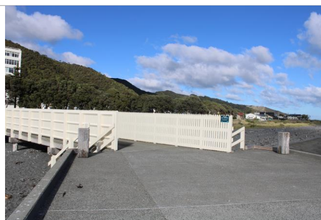
Figure 5: Rona Bay Wharf.
