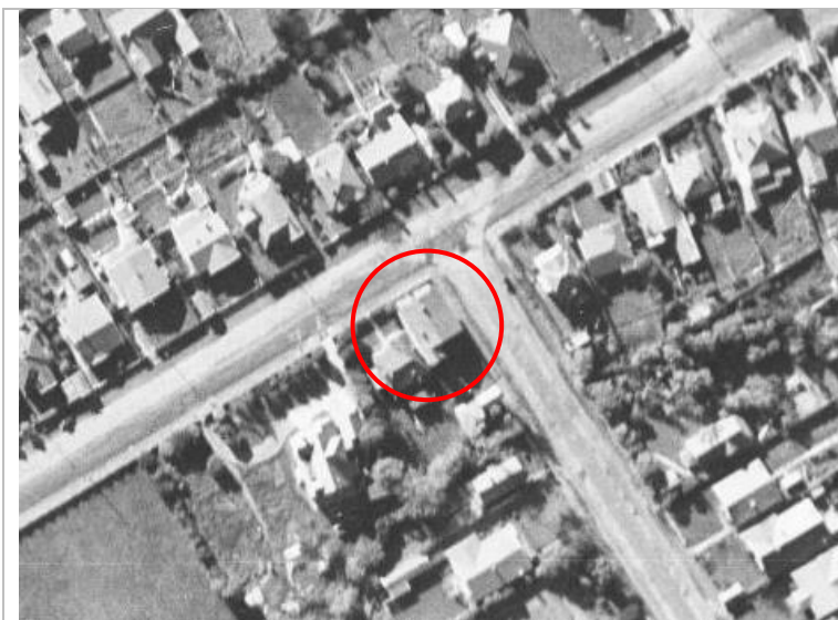
Figure 2: The Offices at 64 Knights Road, 1939. Source: Retrolens
