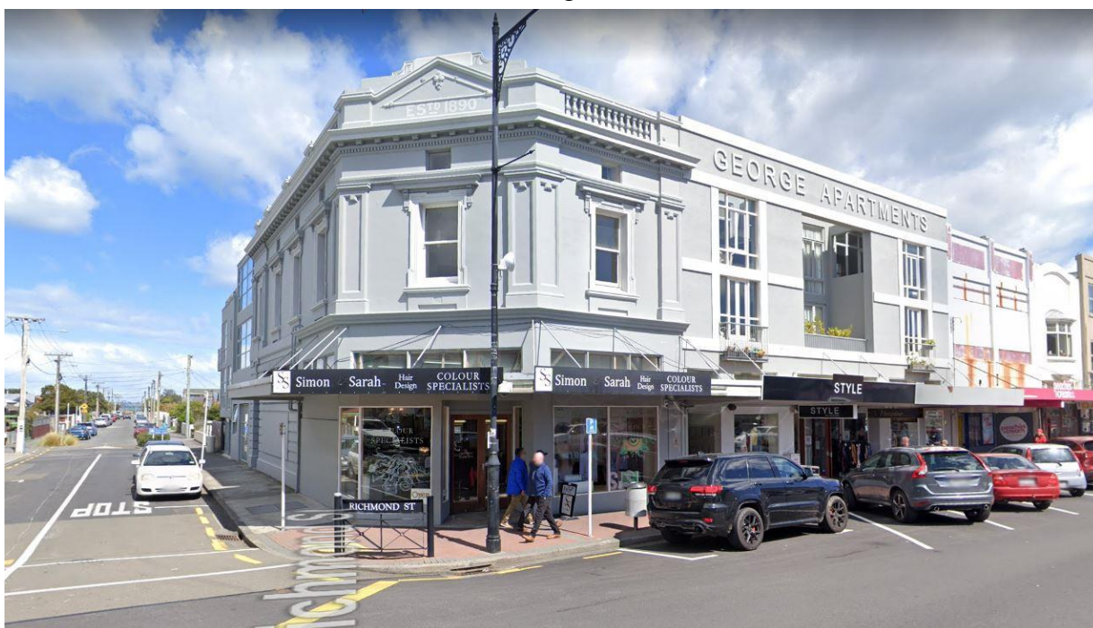
Figure 1: 224 Jackson Street, Petone Source: Google Streetview
