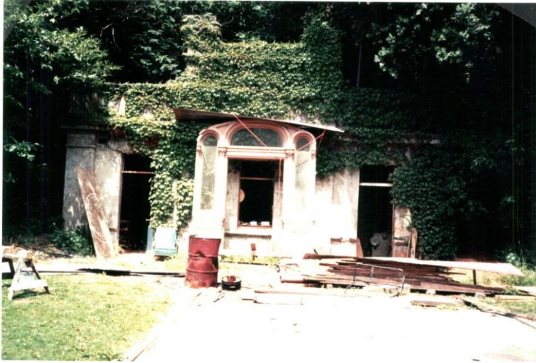
Figure 2: Balgownie Generator Building, c. 1994. Source: HCC Heritage Inventory, 1994
