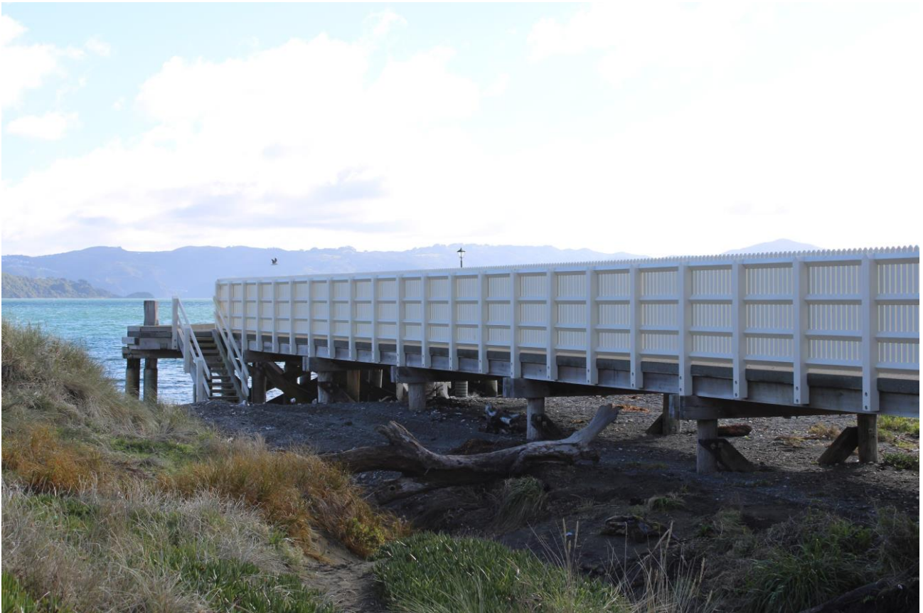
Figure 1: Rona Bay Wharf.
