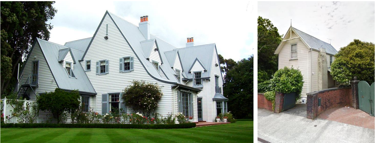
Figure 1: Vogel House at 75 Woburn Road (left), and the gatehouse (right) at 73 Woburn Road.
