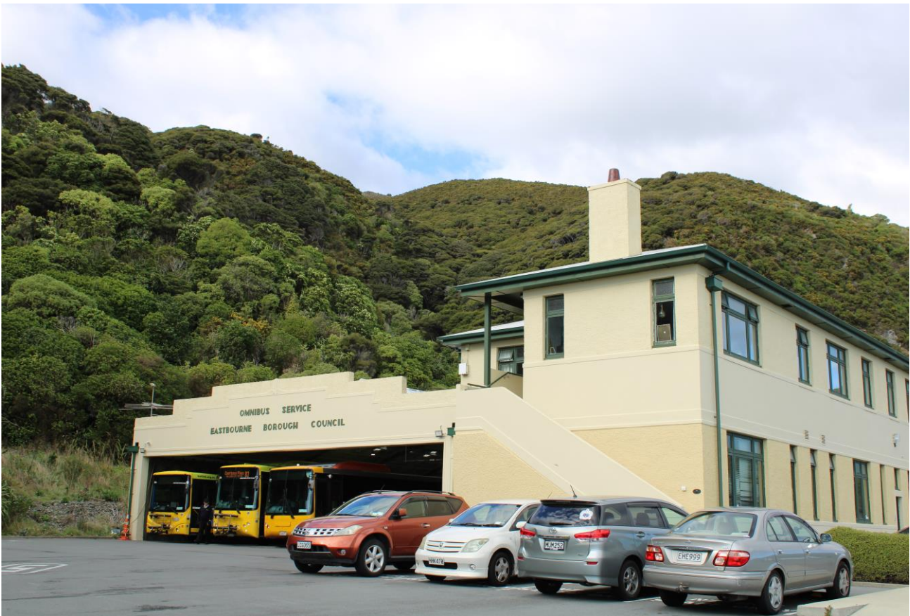
Figure 1: Eastbourne Bus Garage, 493 Muritai Road, Eastbourne.
