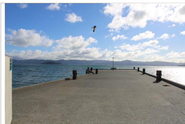
Figure 4: Rona Bay Wharf.
