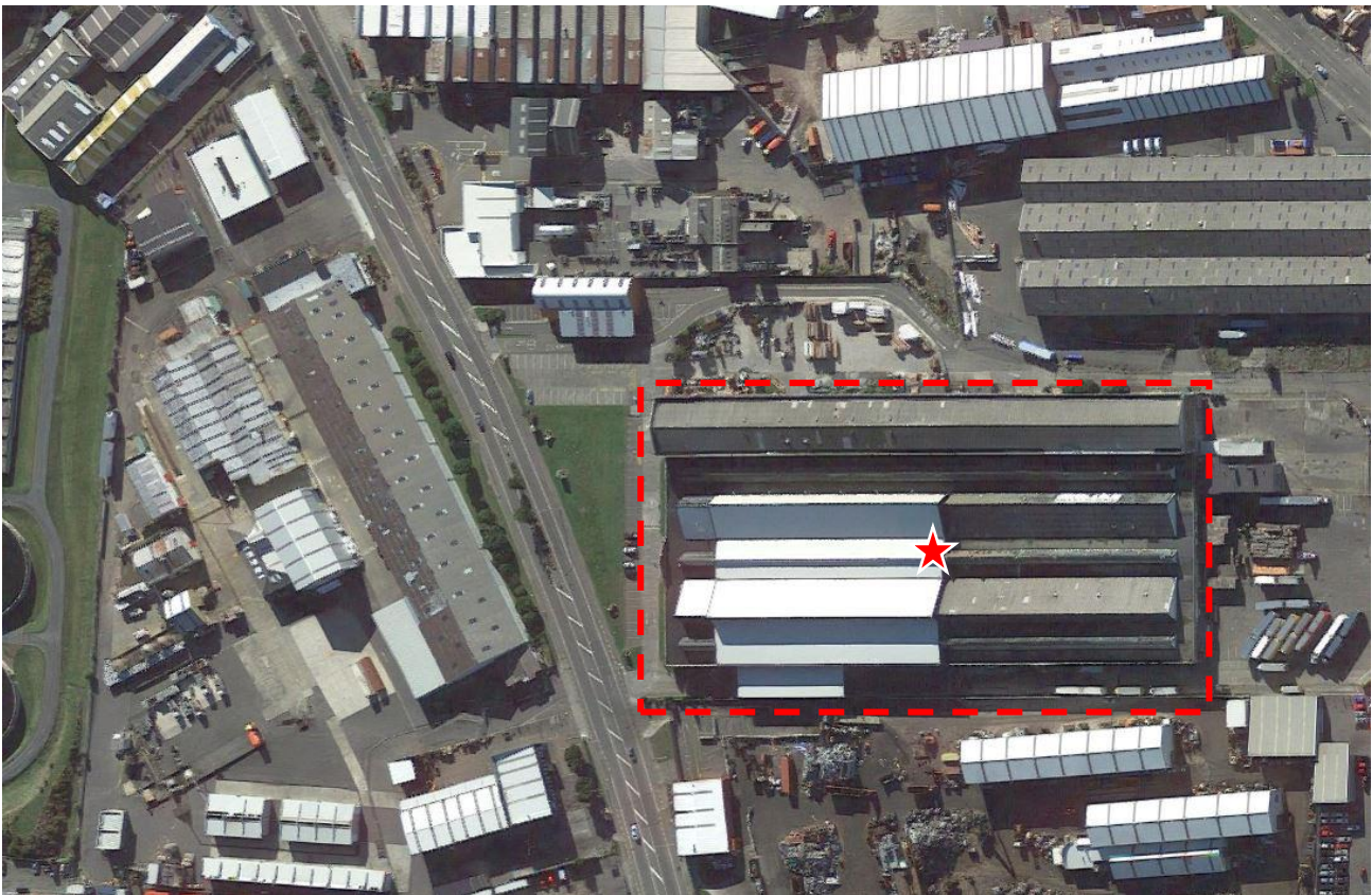
Figure 5: Aerial of the site with heritage structure indicated.
