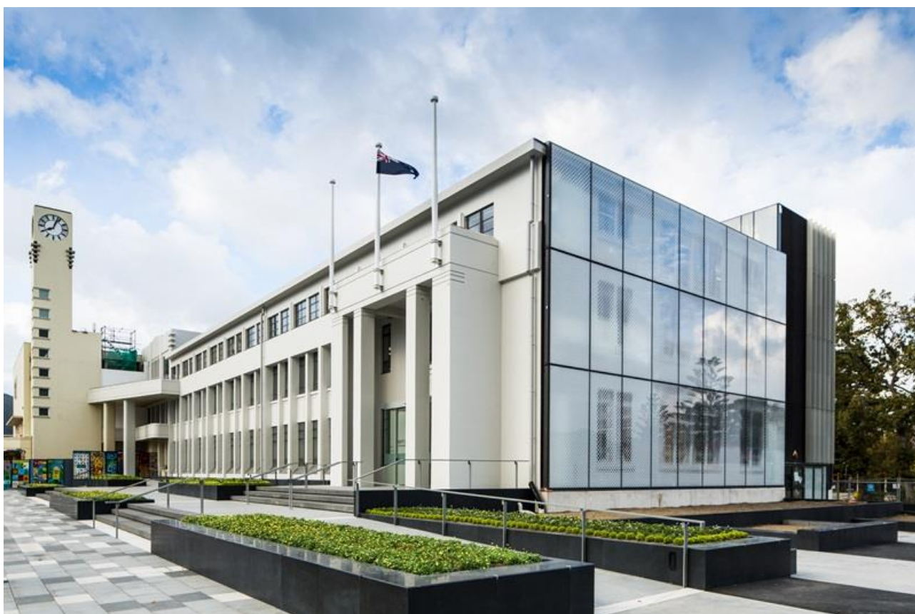
Figure 1: The Town Hall and Administration Block. Source: Naylor Love
