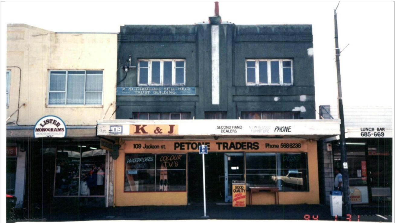
Figure 7: Sutherland Self Help Trust Store, 109 Jackson Street, photographed in 1994. Source: Ian Bowman
