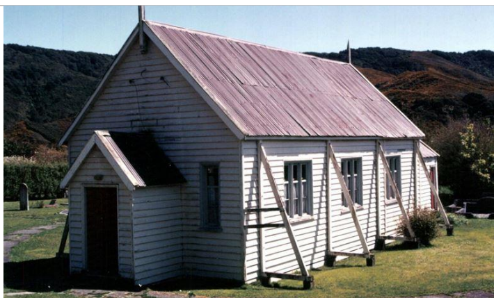
Figure 3: The church in 1994. Source: 1994 HCC Inventory
