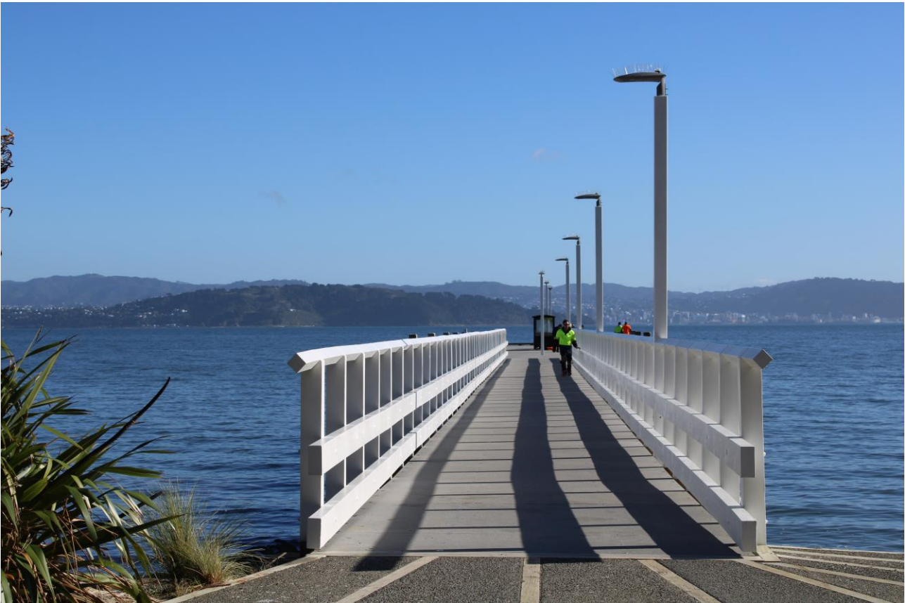
Figure 1: Days Bay Wharf, Days Bay.
