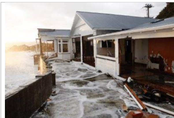
Figure 4: Beachamp Cottage after storm damage, 2013.
