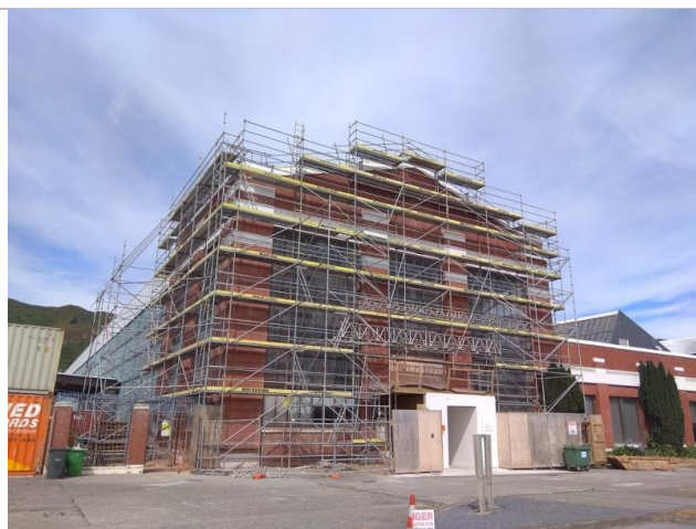
Figure 4: The workshops being upgraded, 2017. Source: Heritage Equip
