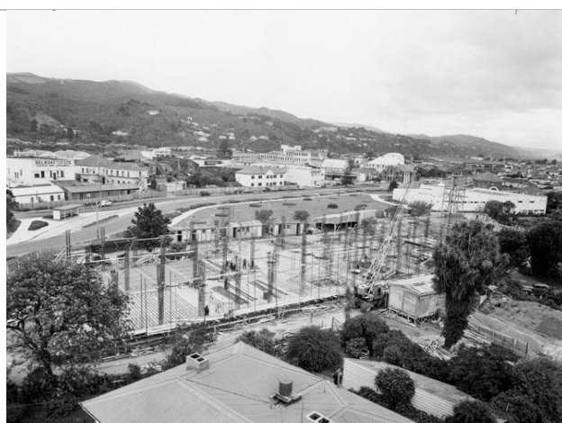
Figure 3: The buildings under construction, 1954. Source: HCC Archives
