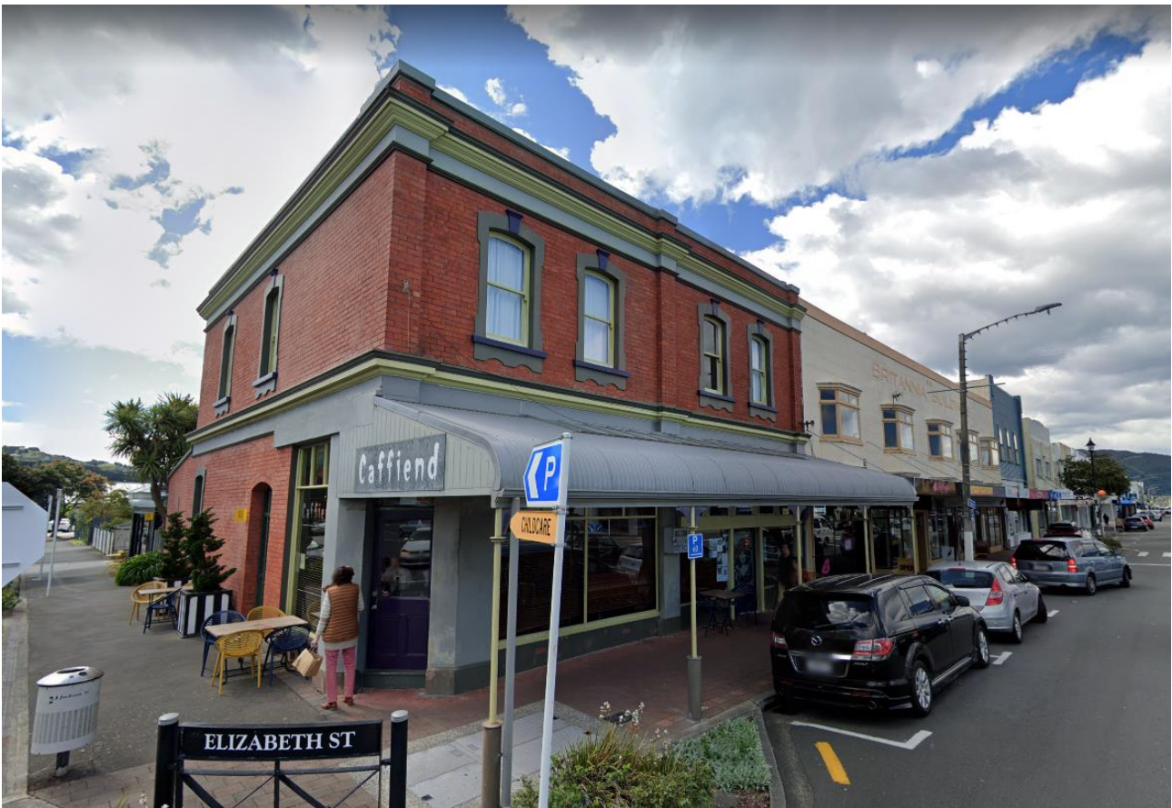
Figure 1: 233-235 Jackson Street, Petone Source: Google Streetview
