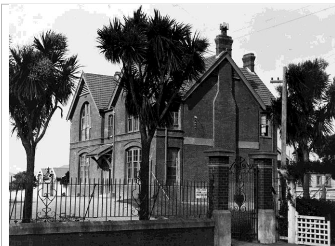
Figure 2: The original brick classrooms of the Petone Memorial Technical College, photographed in 1935 prior to their demolition. Source: ATL, ID: PAColl-6301-37
