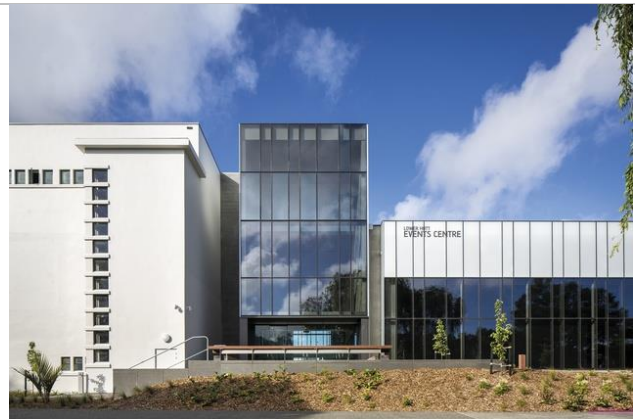
Figure 11: The Town Hall (left) and new Events Centre today after extensive redevelopment. Source: Naylor Love
