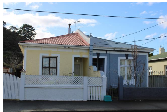
Figure 5: Semi-detached building on Riddlers Crescent.
