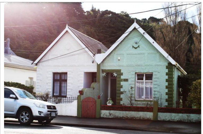
Figure 6: Semi-detached building on Riddlers Crescent.
