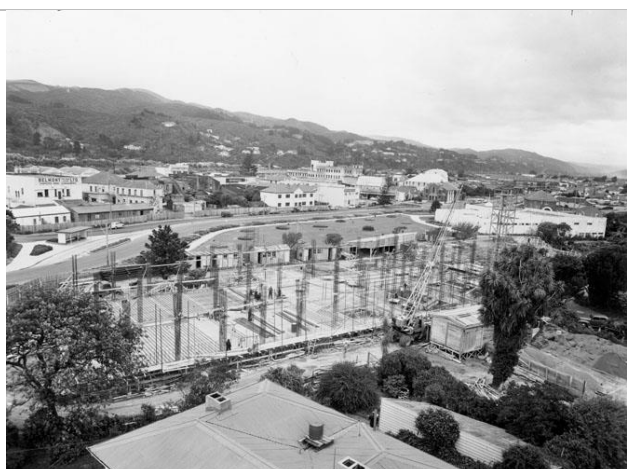
Figure 8: The buildings under construction, 1954. Source: HCC Archives
