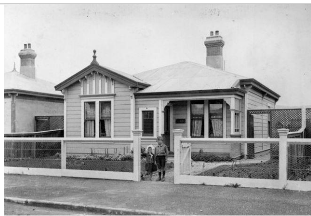
Figure 9: 13 Patrick Street, built in 1908 by the Labour Department. Source: ATL, ID: PA2-O-282-23-6
