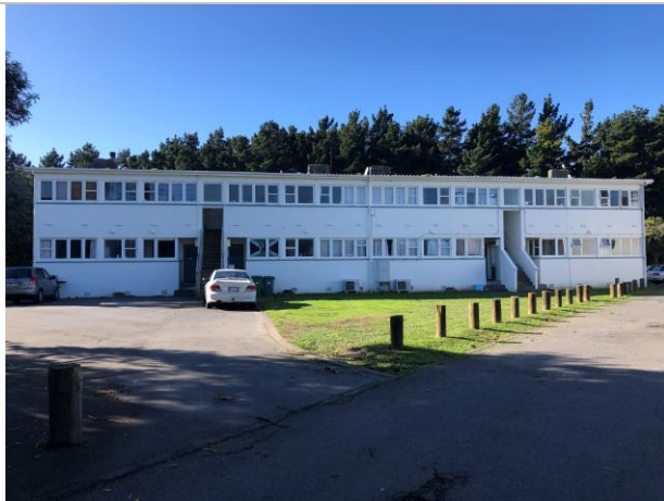
Figure 6: The two storey flats at Hardham Crescent.
