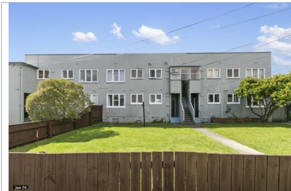
Figure 4: Block of flats on Scholefield Street.
