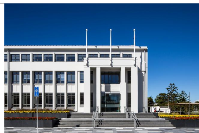
Figure 20: The Administration Block today after extensive redevelopment.
