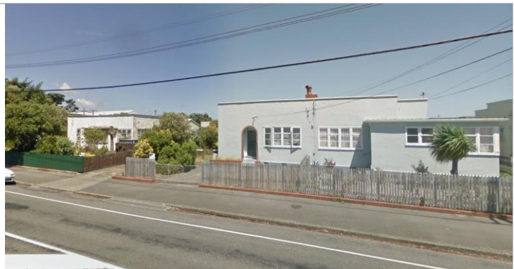
Figure 5: Single storey flats on Jackson Street.
