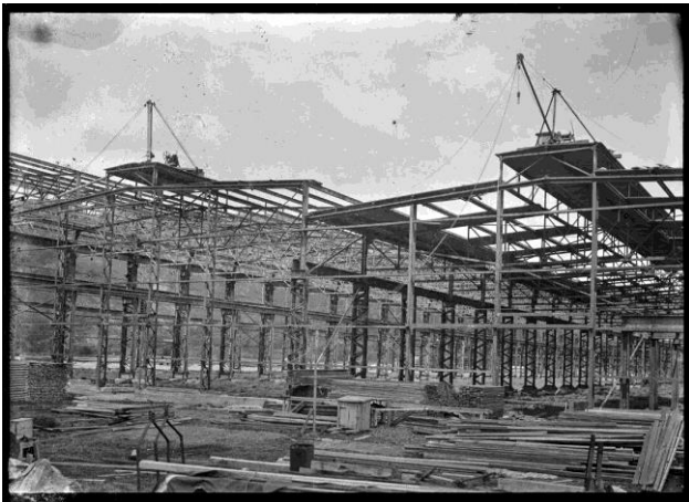
Figure 4: The Hutt Railway Workshops under construction in 1928.
