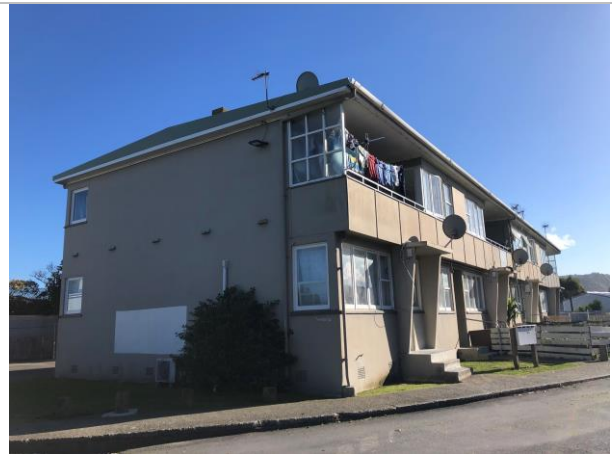
Source: The two storey flats at Hardham Crescent.
