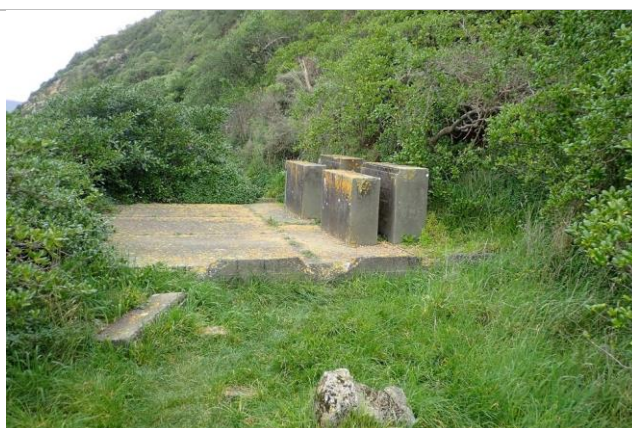
Figure 13: Remnants of the Degaussing Station. Source: Tracesofwar.com
