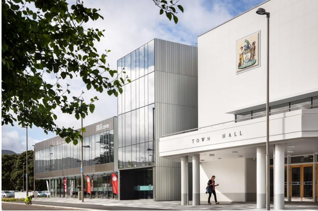
Figure 22: The Town Hall and new Events Centre today after extensive redevelopment. Source: Naylor Love
