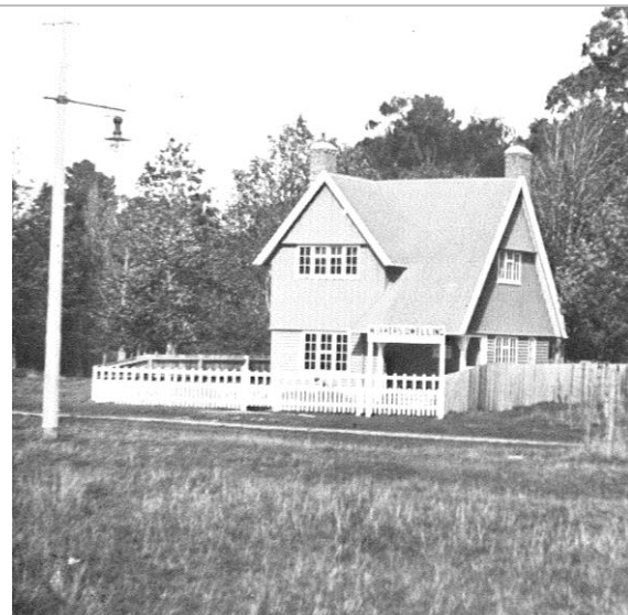
Figure 5: Full-scale 'Workers Dwelling' built for the International Exhibition at Christchurch held between November 1906 and April 1907, designed by Samuel Hurst Seager and Cecil Wood. Source: HNZPT 1984 Booklet
