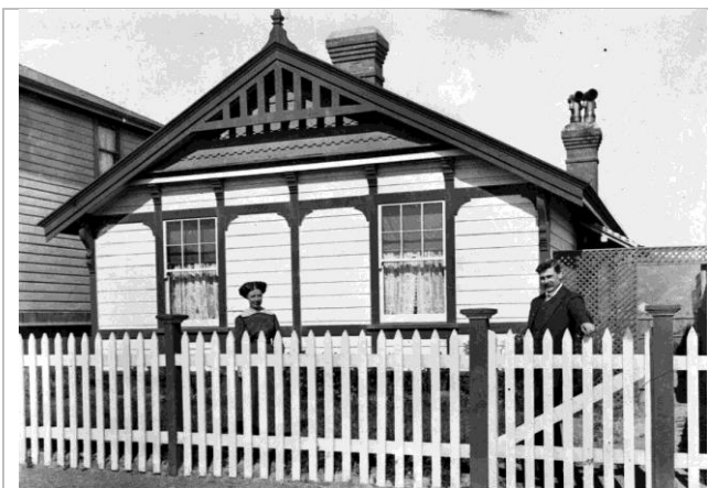
Figure 8: 2 Patrick Street, built in 1906 as part of the Heretaunga Settlement scheme, photographed in 1908. Source: ATL, ID: PA1-O-195-20-2
