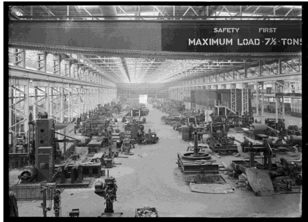
Figure 5: The interior of the completed workshops, 1929.
