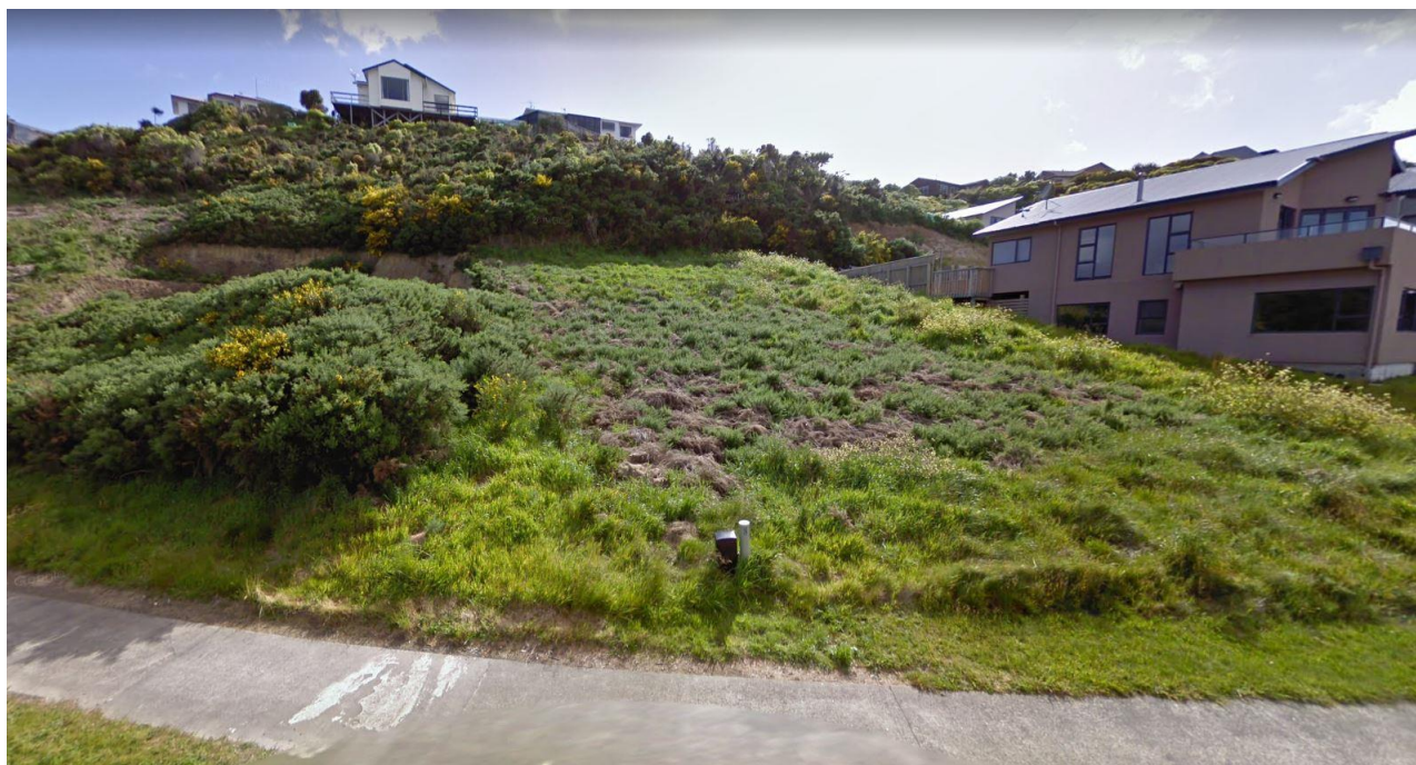
Figure 5: Cedar Street, Maungaraki, showing different stages of slope modification for residential development. Note cut slopes behind the house on the right, and in the plot to the left. (Image from Google Maps Street View).
