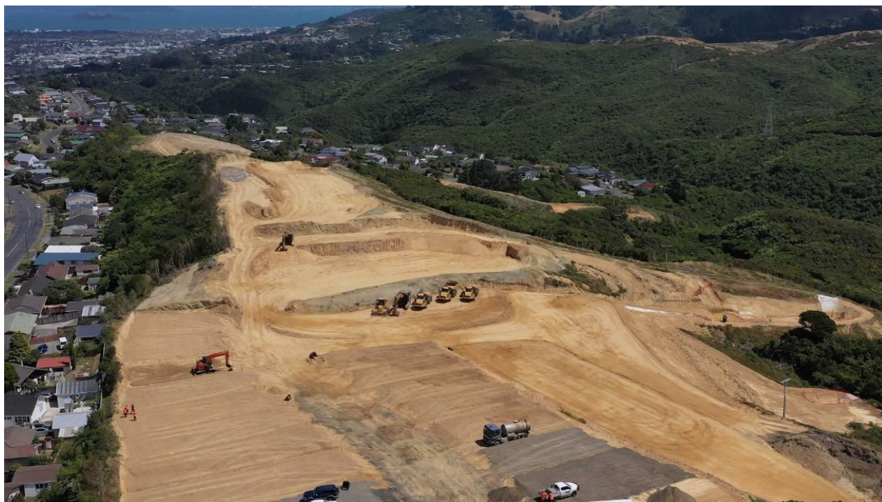
Figure 7: Slope modification, including some small residential cuts and fills, at a recent subdivision in Kelson. (Photo from Stuff).
