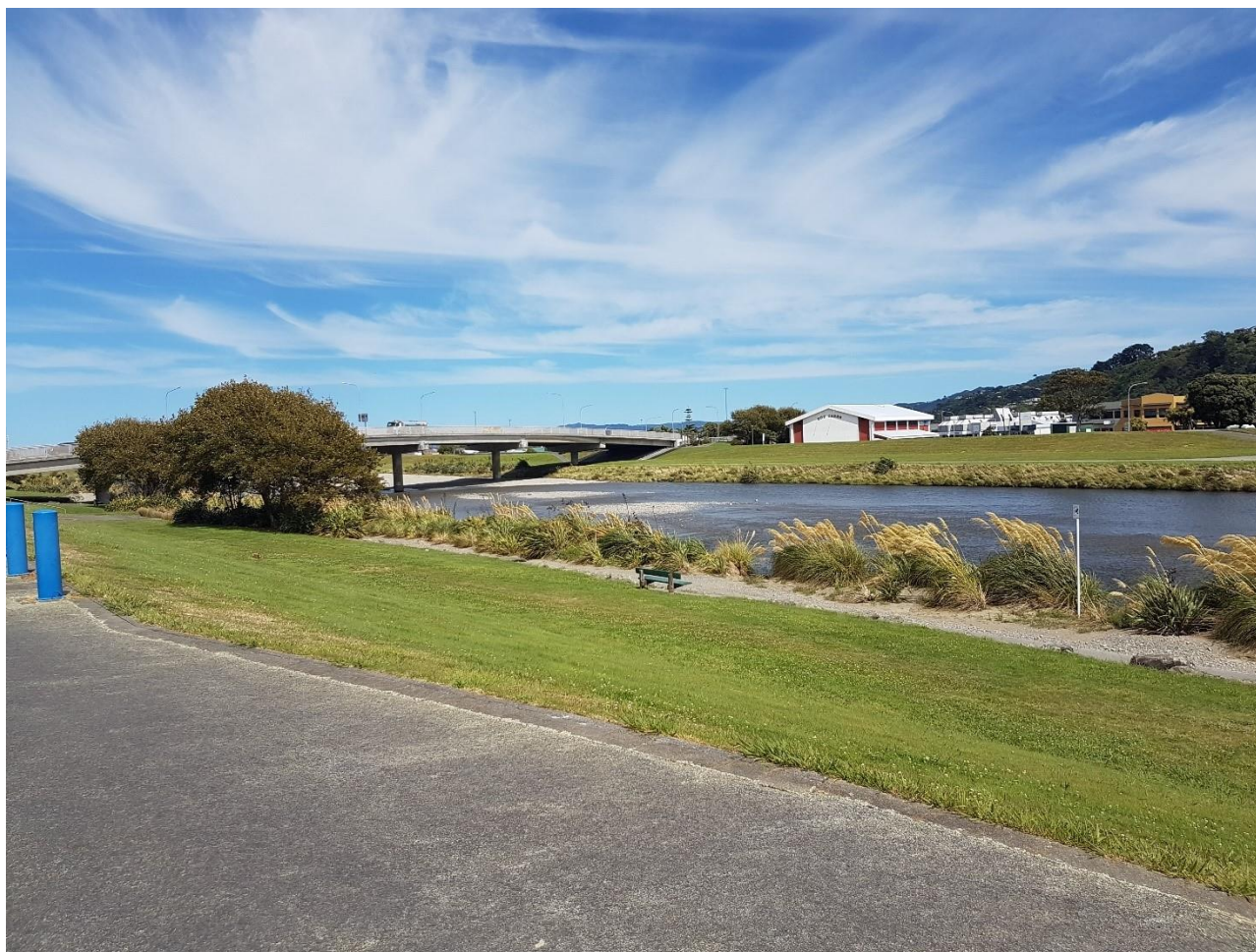
Figure 10: Stopbanks to either side of the Hutt River.
