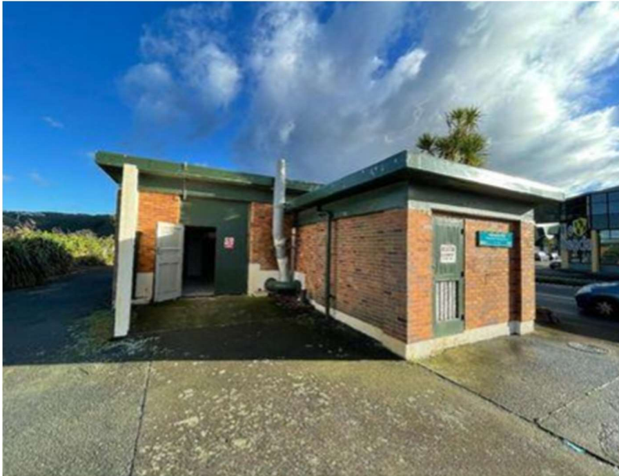
Figure 2 Esplanade West Wastewater Pumpstation
