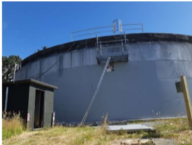
Figure 8 Gracefield Water Supply Reservoir
