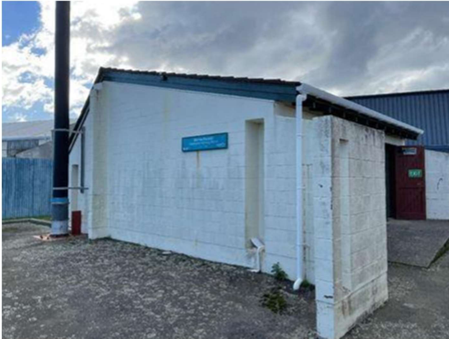
Figure 4 Marine Parade Wastewater Pumpstation
