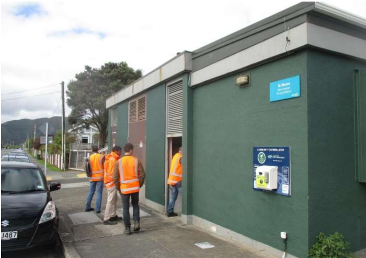
Figure 5 Te Mome Stormwater Pumpstation
