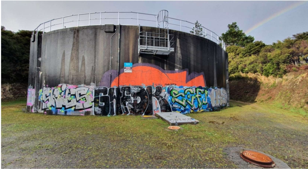
Figure 6 Gawler Grove Reservoir
