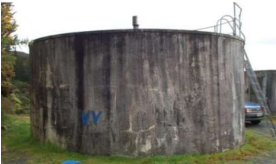
Figure 14 Rata Street Water Supply Reservoir
