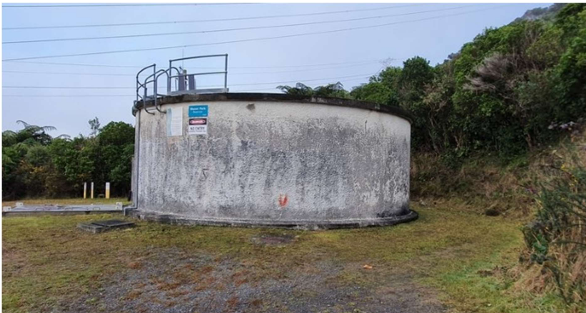
Figure 10 Manor Park Water Reservoir
