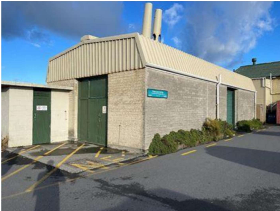
Figure 1 Esplanade Central Wastewater Pumpstation
