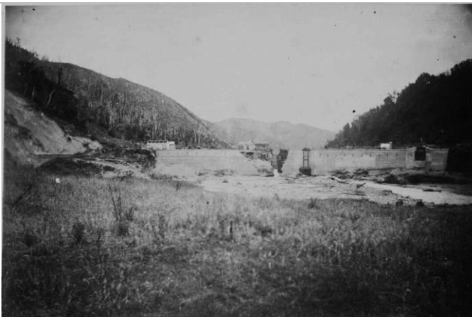
Figure 2: Damage to the Lower Dam while under construction, 1844.
