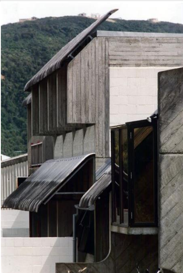
Figure 4: The strong geometric forms of raw concrete with original roofing to the office buildings, which has since been replaced, undated. Source: Moller Architects
