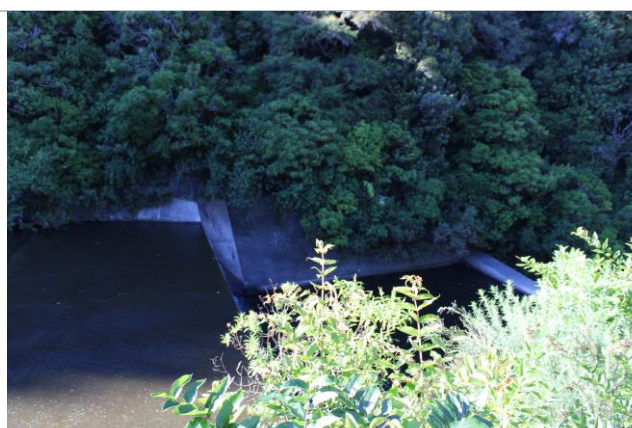
Figure 11: The spillway of the Lower Dam.
