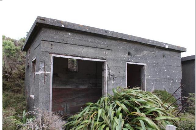
Figure 3: One of the intact reinforced concrete observation posts.
