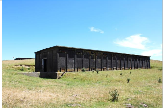
Figure 15: One of the longer flat-roofed ammunition stores. The top and bottom vents are clearly visible.
