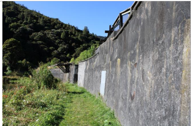
Figure 7: The reinforced concrete wall of the Lower Dam
