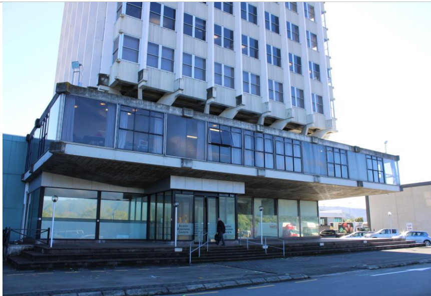
Figure 5: The cantilevered second floor 'plinth' to Avalon Studios tower.
