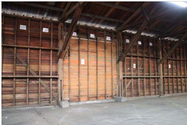
Figure 8: Internal timber wall structure of the warehouses showing a boarded up section of wall which used to house a sliding door.
