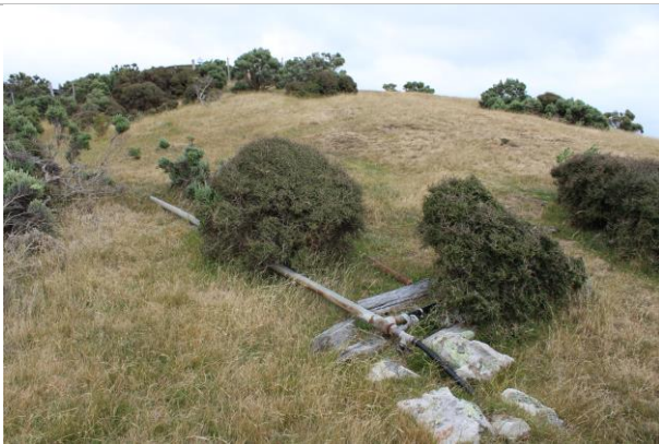
Figure 8: Extant pipes used to transfer water from the pumphouse at the bottom of the hill to the WWII bunkers at the top of the hill.
