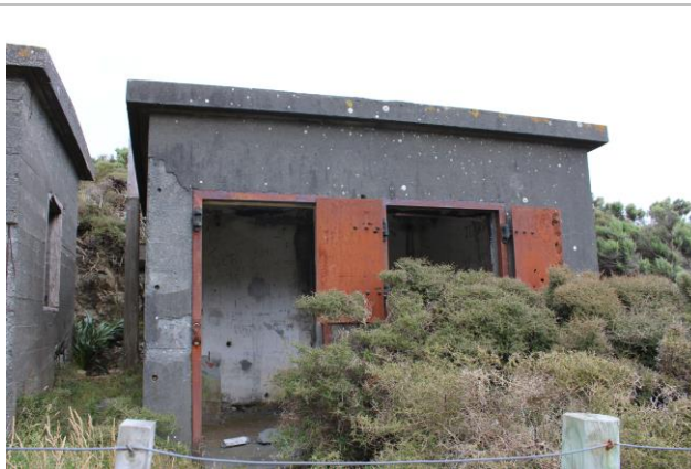
Figure 4: One of the intact reinforced concrete observation posts.
