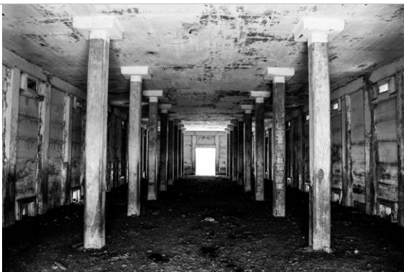
Figure 6: Interior of the flat-roofed ammunition stores, supported by concrete pillars.
