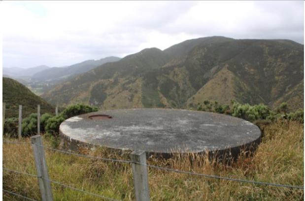
Figure 7: The water tank at the top of the hill which supplied the WWII bunkers.
