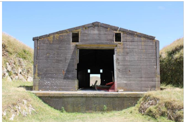
Figure 13: End elevation of one of the gabled ammunition stores, with earth mounds to either side.
