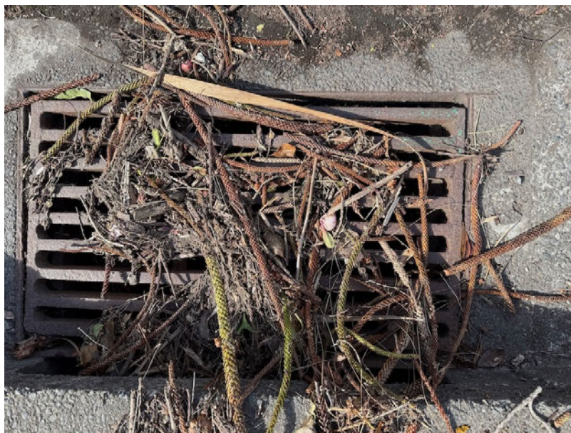
Photo 1. One of two blocked drain gratings at end of street
