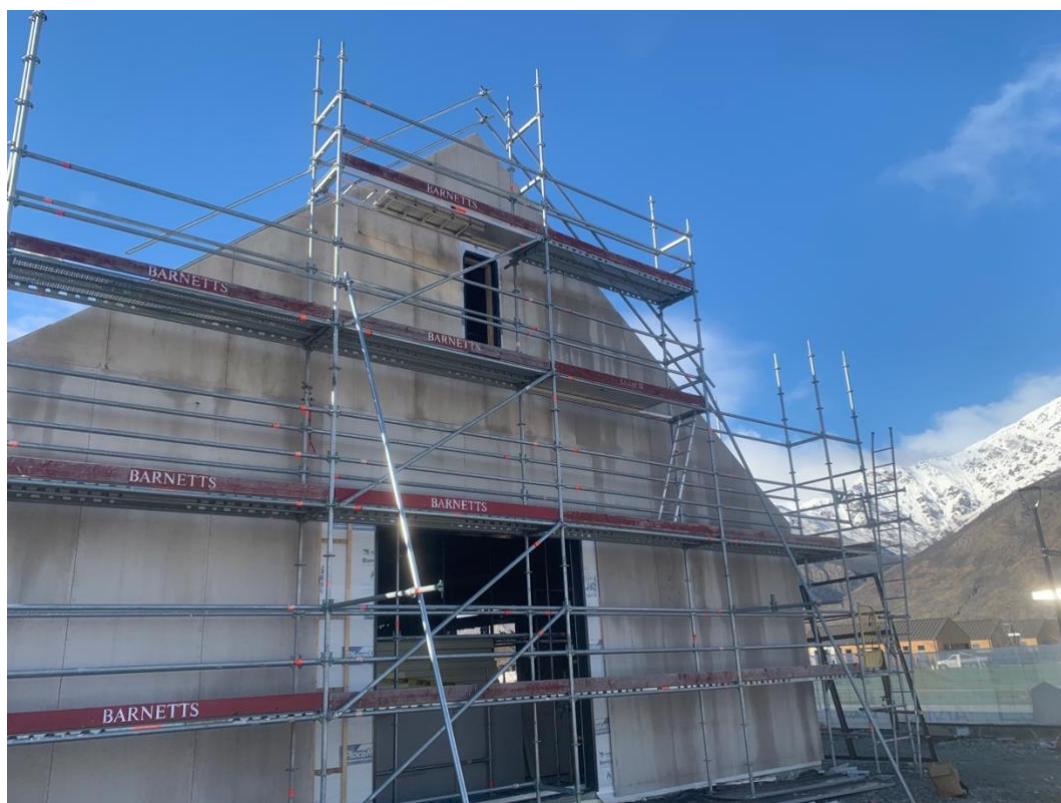
Figure 7 Photograph scaffold with outriggers, credit: Wain Chambers
