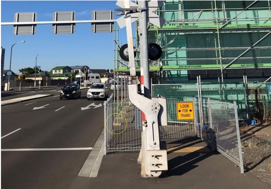
Figure 4 Scaffold obscuring signals for road traffic at a level crossing – view from rail
