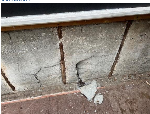
Figure 2 – Area of existing façade where the existing steel reinforcing has corroded causing expansion and breakout of existing concrete
