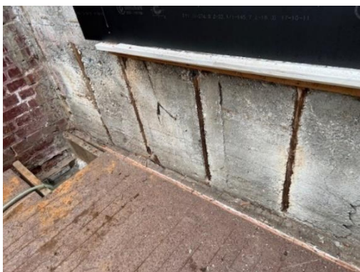
Figure 1 – General condition of existing façade being porous and Boney and generally in poor condition
