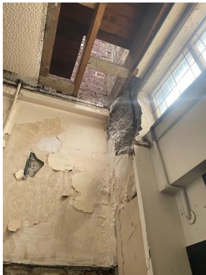
Figure 3 – Existing column where significant breakout has occurred due to corrosion of existing reinforcing steel.
