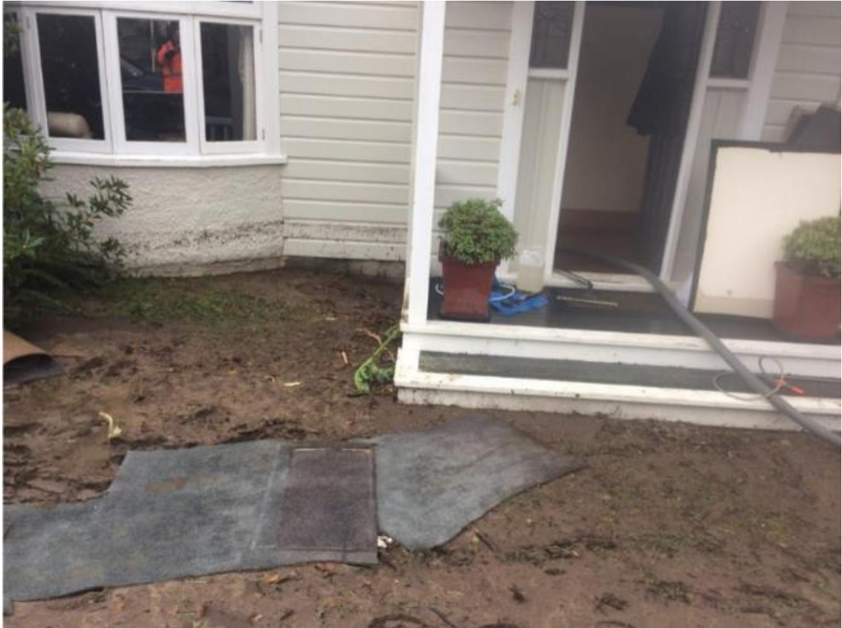
Figure 28 Flooding at 94 Muritai Rd during 7 April 2019 storm event
