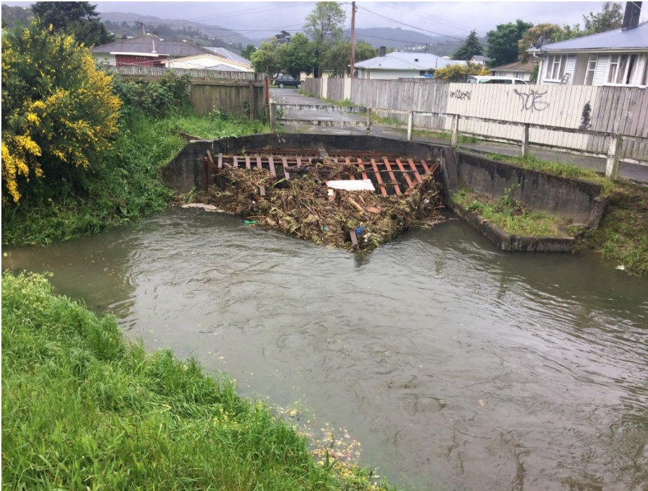
Figure 4-50: Stokes Valley Stream – trash screen near Kamahi Park following the 15 November 2016 rainfall event.
