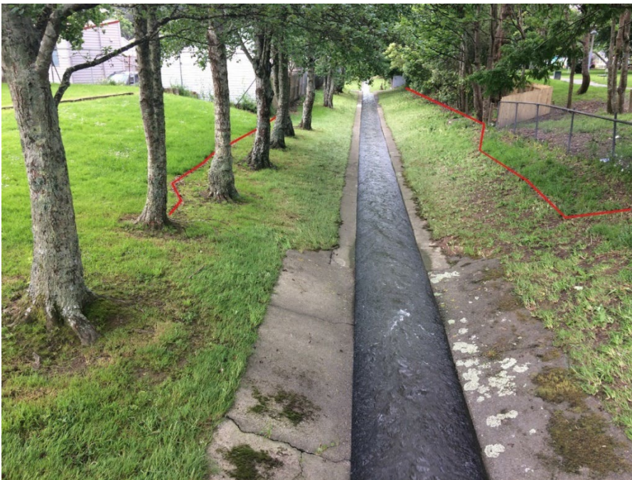
Figure 4-33: Stokes Valley Stream near Delaney Park following the 15 November 2016 rainfall event.
