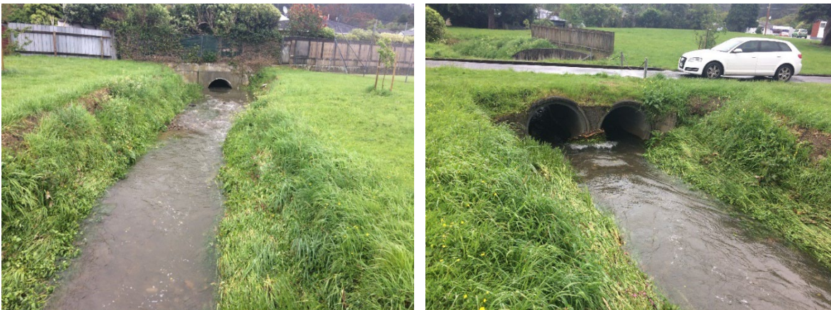
Figure 4-46: Upstream at Kamahi Park, 1200mm culvert (left), downstream Twin 1200mm barrels under crossing (right)
