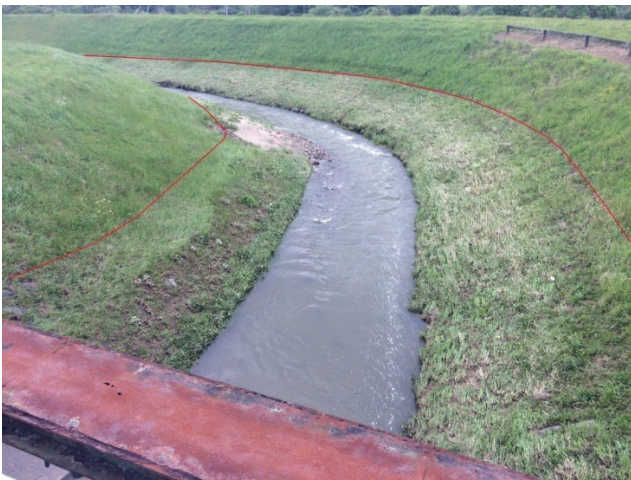
Figure 4-22: Stokes Valley Stream looking downstream from Eastern Hutt Road.
