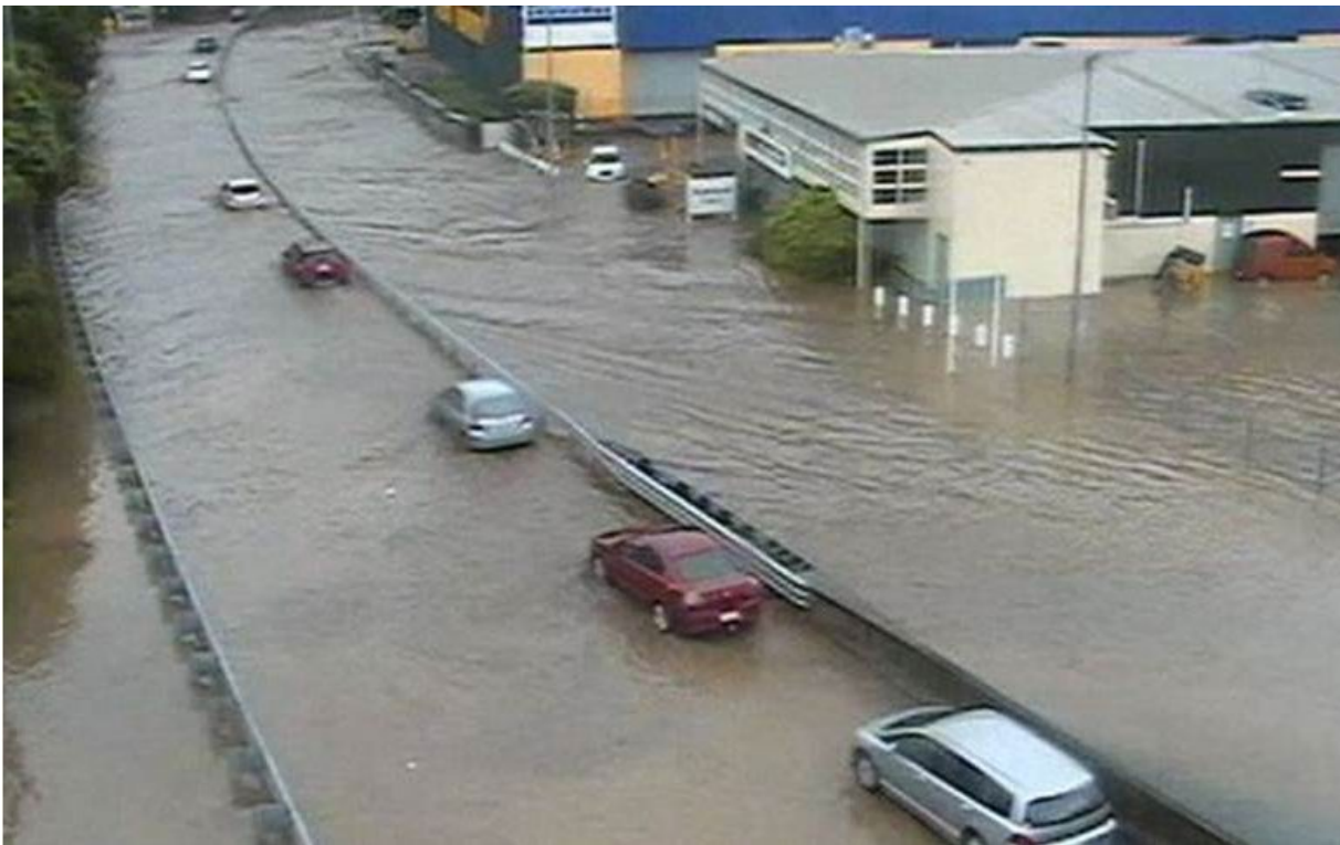
Figure 2-2 Flooding from the Korokoro catchment on SH2 near Ulrich Aluminium (14 May 2015).
