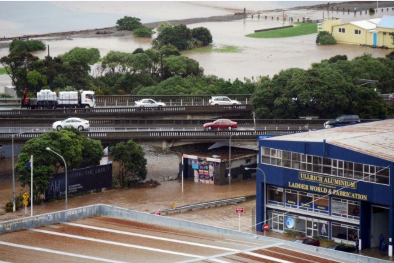
Figure 2-3 Flooding on SH2 during the 14 May 2015 event
