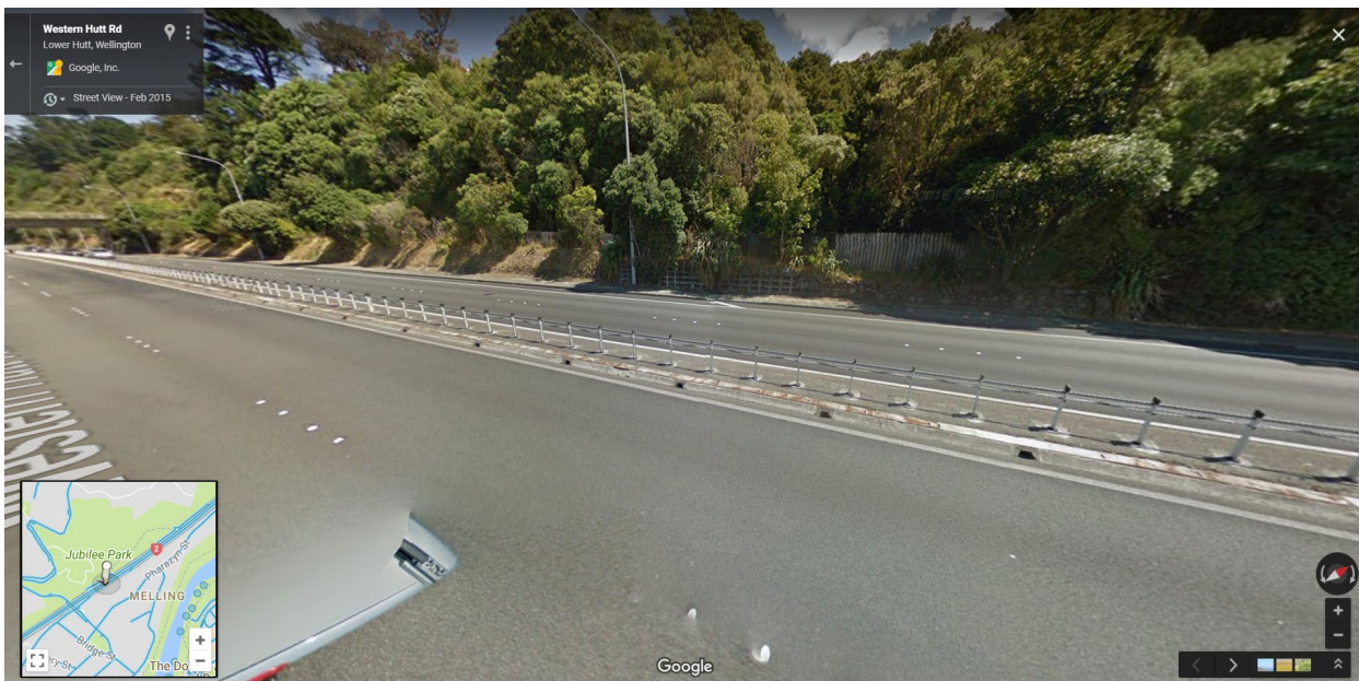
Figure A1 SH2 southbound lane, showing small drainage inlets near Melling. Image from Google Street View.
