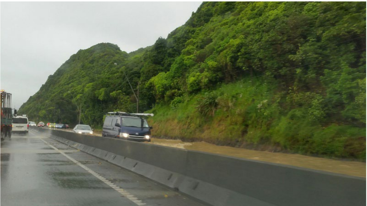
Figure 5-21 SH2 Flooding in the north bound lane (Radio New Zealand, 2016), Photographer Kate Gudsell
