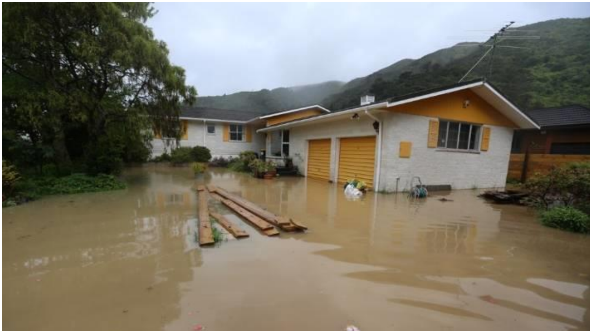
Figure 2-4 Impact of the Waiwhetū Stream Bursting its Banks During 2016 Event. Photo from Cameron Burnell quoted in (Weekes, 2016).
