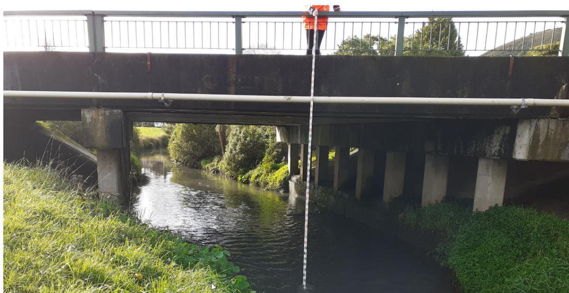
Figure 3-11 Cleary St bridge site photo
