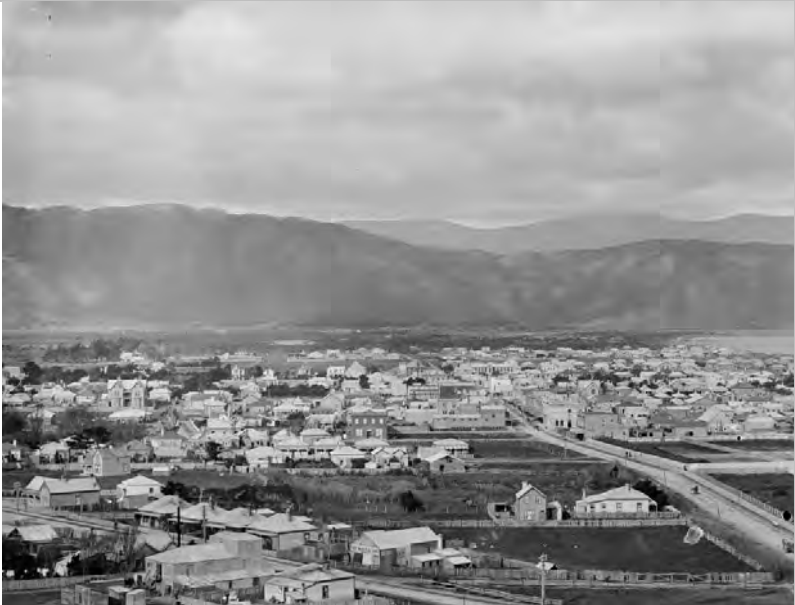
Figure 4: Looking across Jackson Street, 1902. Source: ATL
