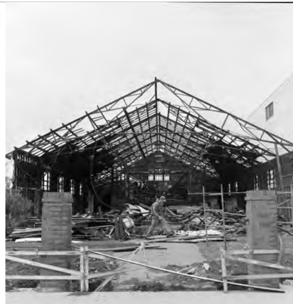
Figure 17: Demolition of the Horticultural Hall in 1958 after fire damage.
