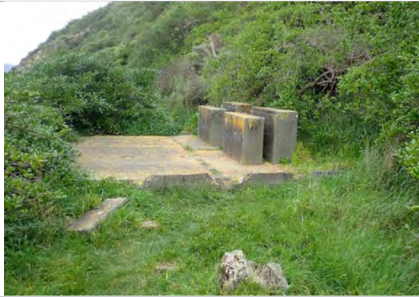
Figure 14: Remnants of the Degaussing Station. Source: Tracesofwar.com
