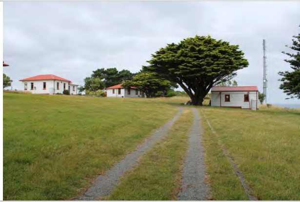
Figure 13: The original road leading towards the collection of buildings.
