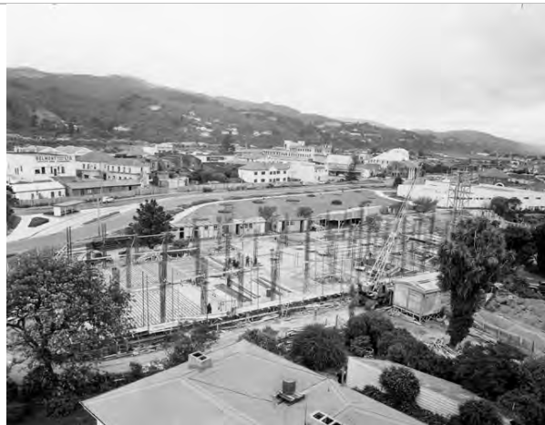
Figure 9: The buildings under construction, 1954. Source: HCC Archives
