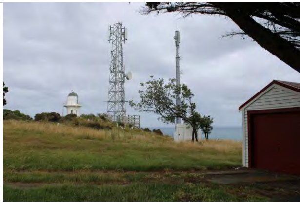
Figure 15: Radio mast and cellphone towers on the site.
