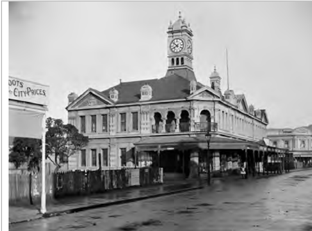
Figure 5: The Petone Council Chambers on Jackson Street (now demolished), c.1913. Source: ATL
