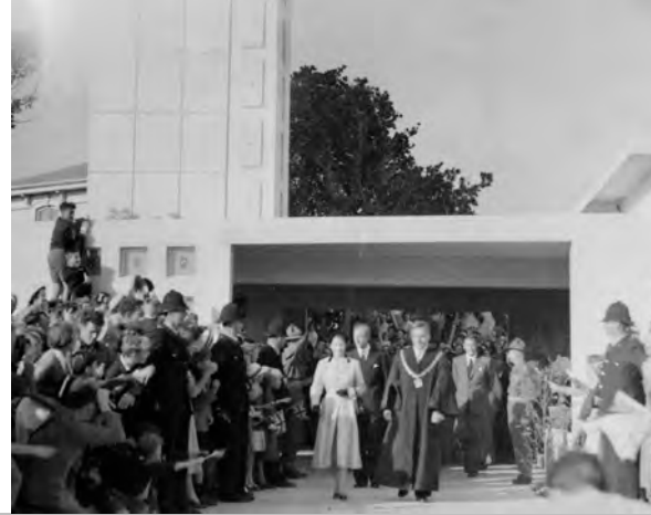
Figure 7: QEII visits the completed church, 1953. Source: HCC Archives
