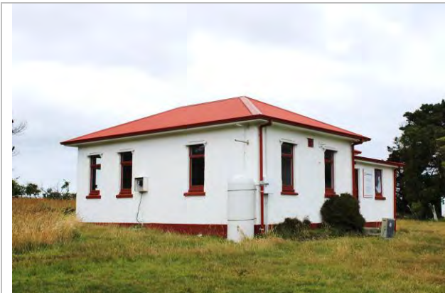
Figure 11: The powerhouse, restored by the Friends of Baring Head conservation group with new interpretative material installed inside for visitors.
