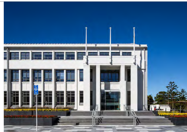
Figure 21: The Administration Block today after extensive redevelopment. Source: Architecture Now
