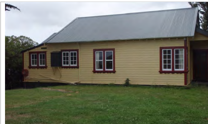
Figure 7: The Caretakers Cottage.
