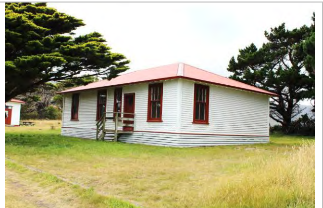
Figure 12: One of the 'keepers cottages, restored by the Friends of Baring Head conservation group.
