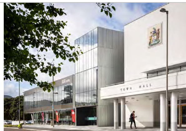
Figure 23: The Town Hall and new Events Centre today after extensive redevelopment. Source: Naylor Love
