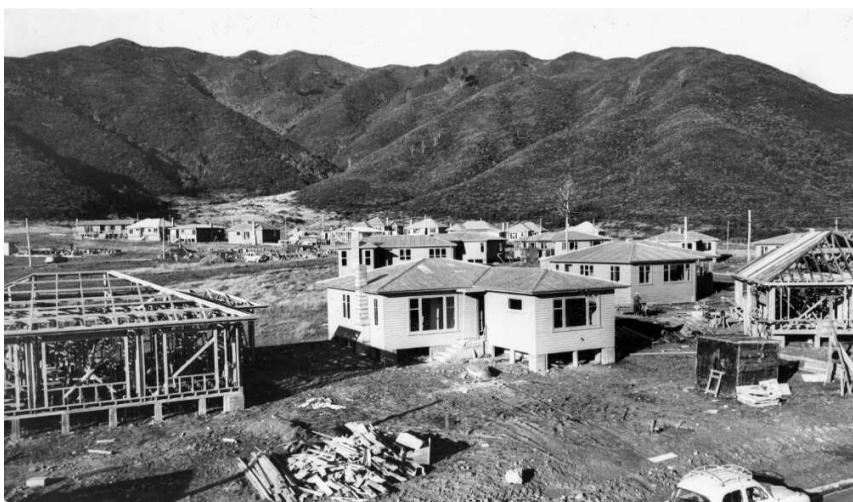
Figure 6: Houses being built in Wainuiomata, 1961. Source: ATL PAColl-9150-10
