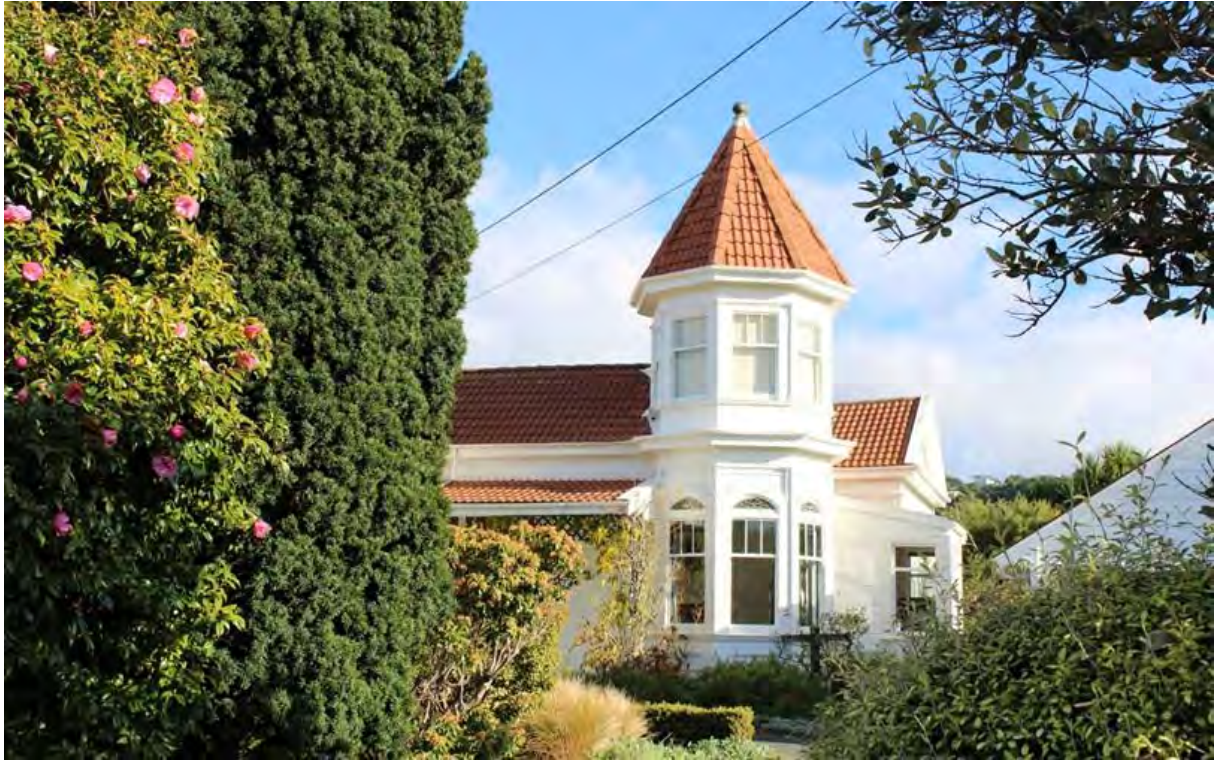
Figure 1: House at 57 Britannia Street, Petone.
