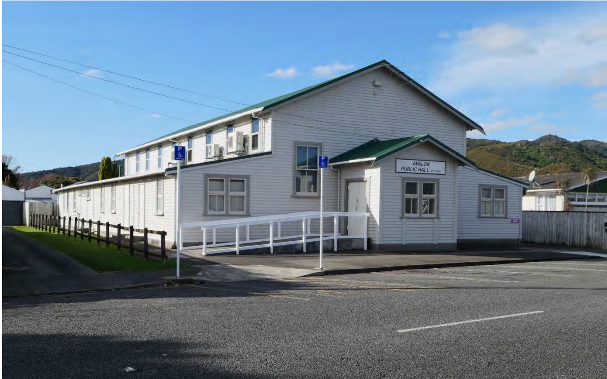
14 Mabey Road (Avalon Hall), June 2024
