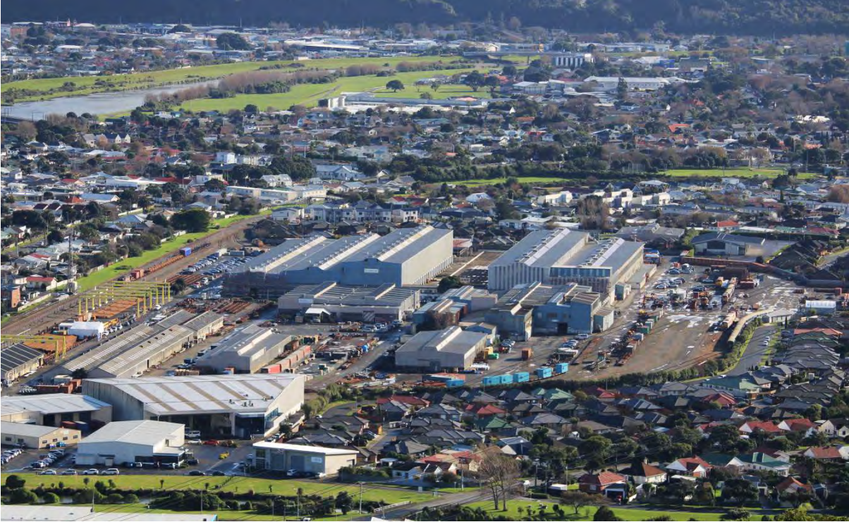
View of workshops, date unknown (courtesy of WSP)
