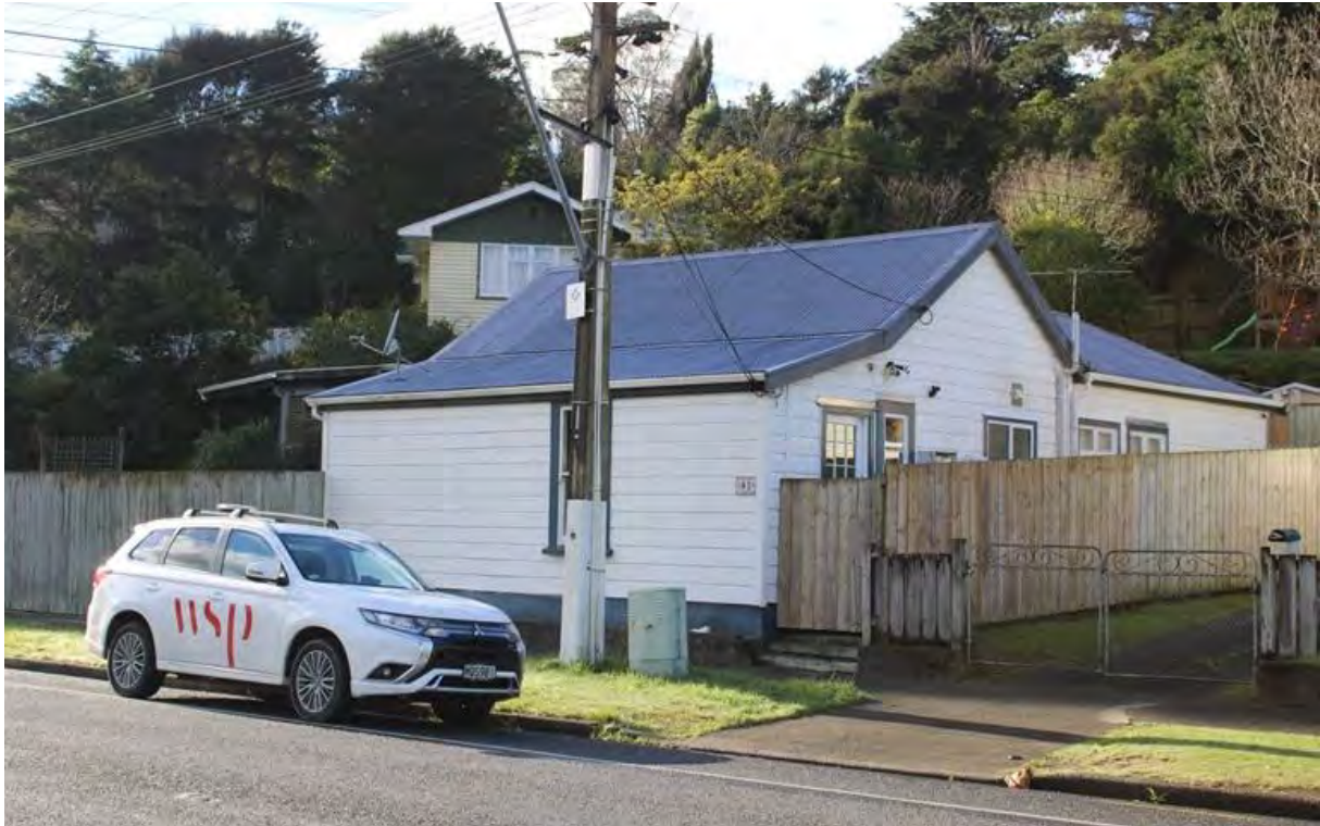
Figure 1: Old Stokes Valley School House, 81 Stokes Valley Road.
