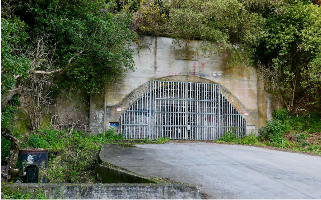
The northern portal of the tunnel, July 2024
