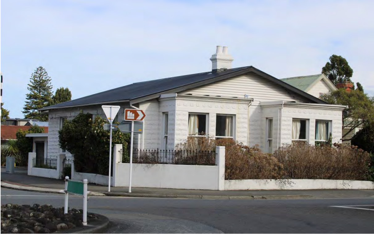
Figure 1: Offices, 64 Knights Road, Lower Hutt.
