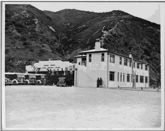
Figure 2: The Eastbourne Bus Garage, 1939. Source: ATL, ID: 1-2-050282-F.
