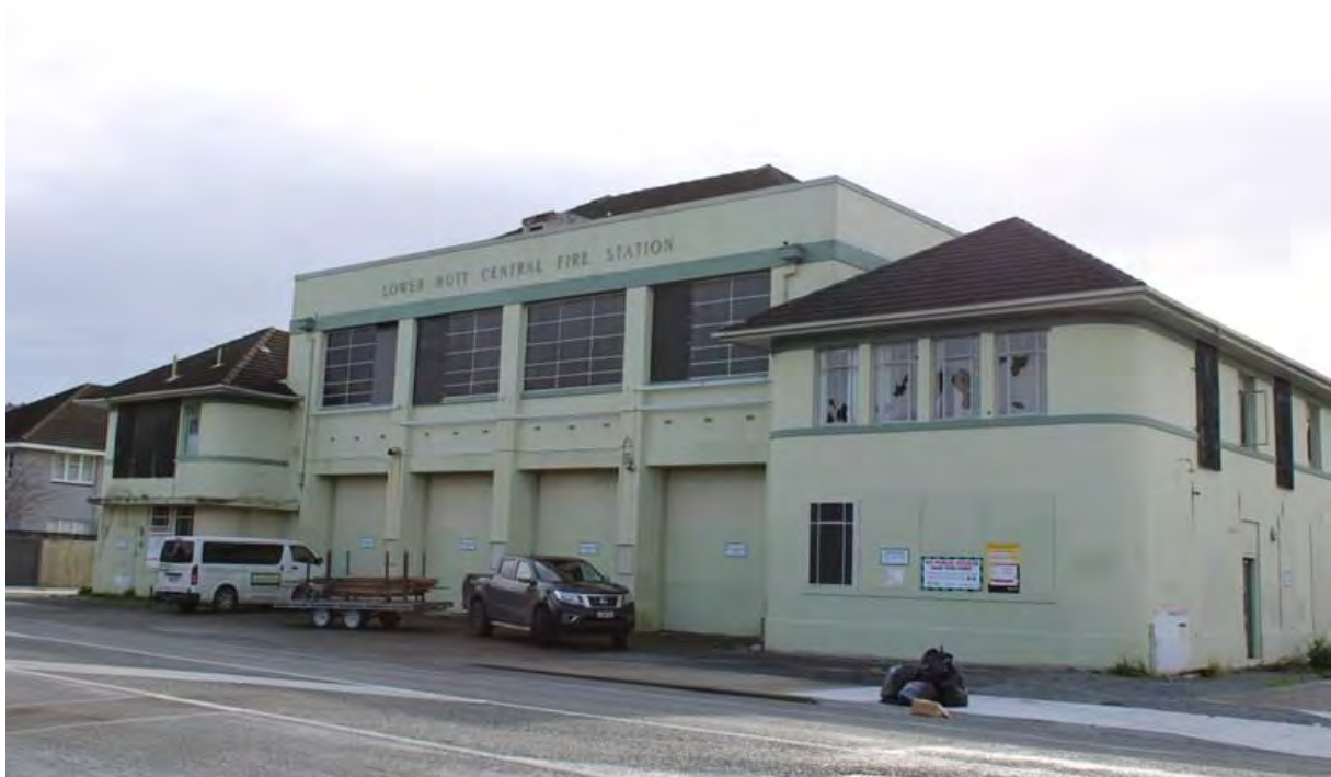
Figure 1: Lower Hutt Fire Station, Hutt Central.
