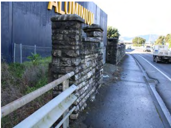
Figure 4: The northern section of wall with vertical posts and coping.
