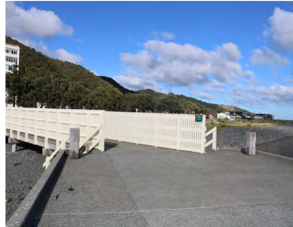
Figure 5: Rona Bay Wharf.
