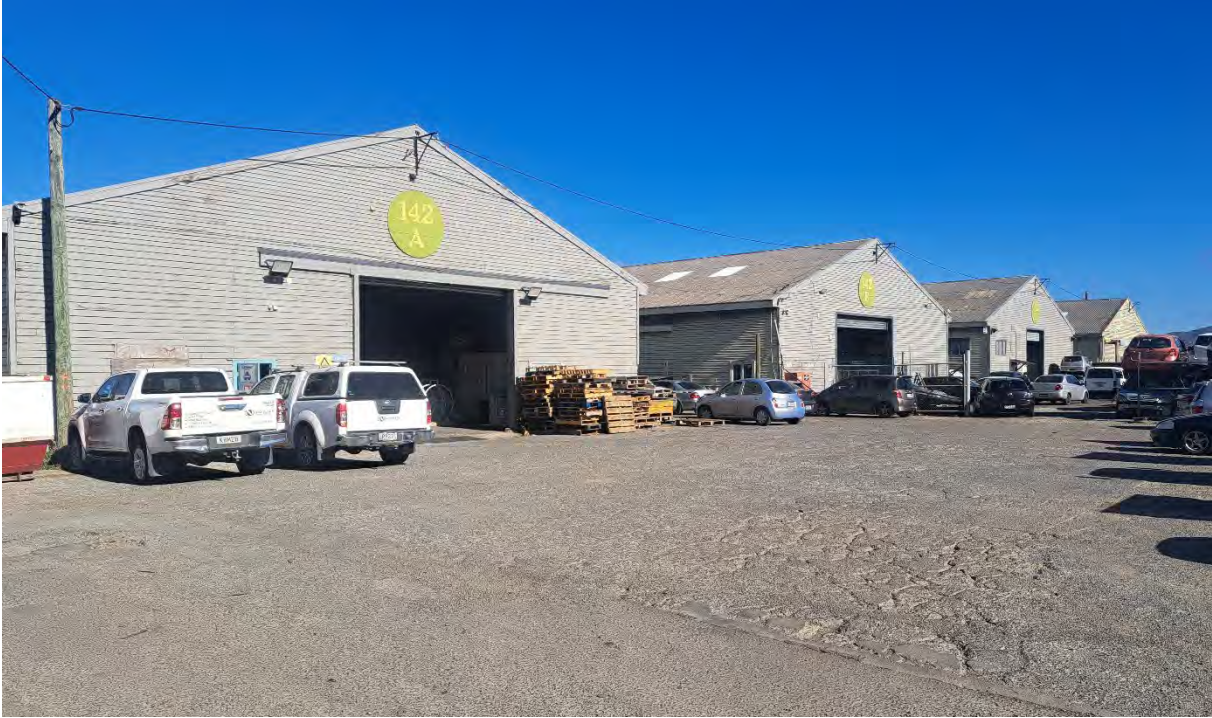
Warehouses, 142 Hutt Park Road, April 2024
