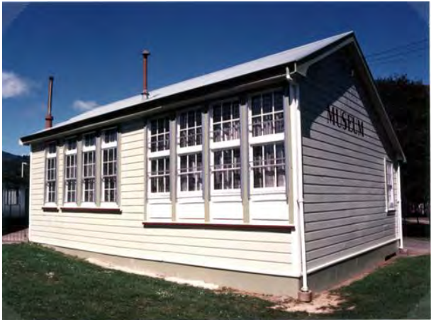
Figure 3: The schoolhouse, now used as a museum, in 1994. Source: 1994 HCC Inventory.
