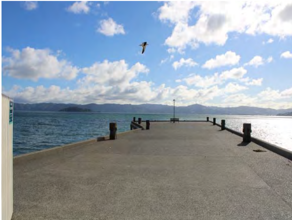
Figure 4: Rona Bay Wharf.
