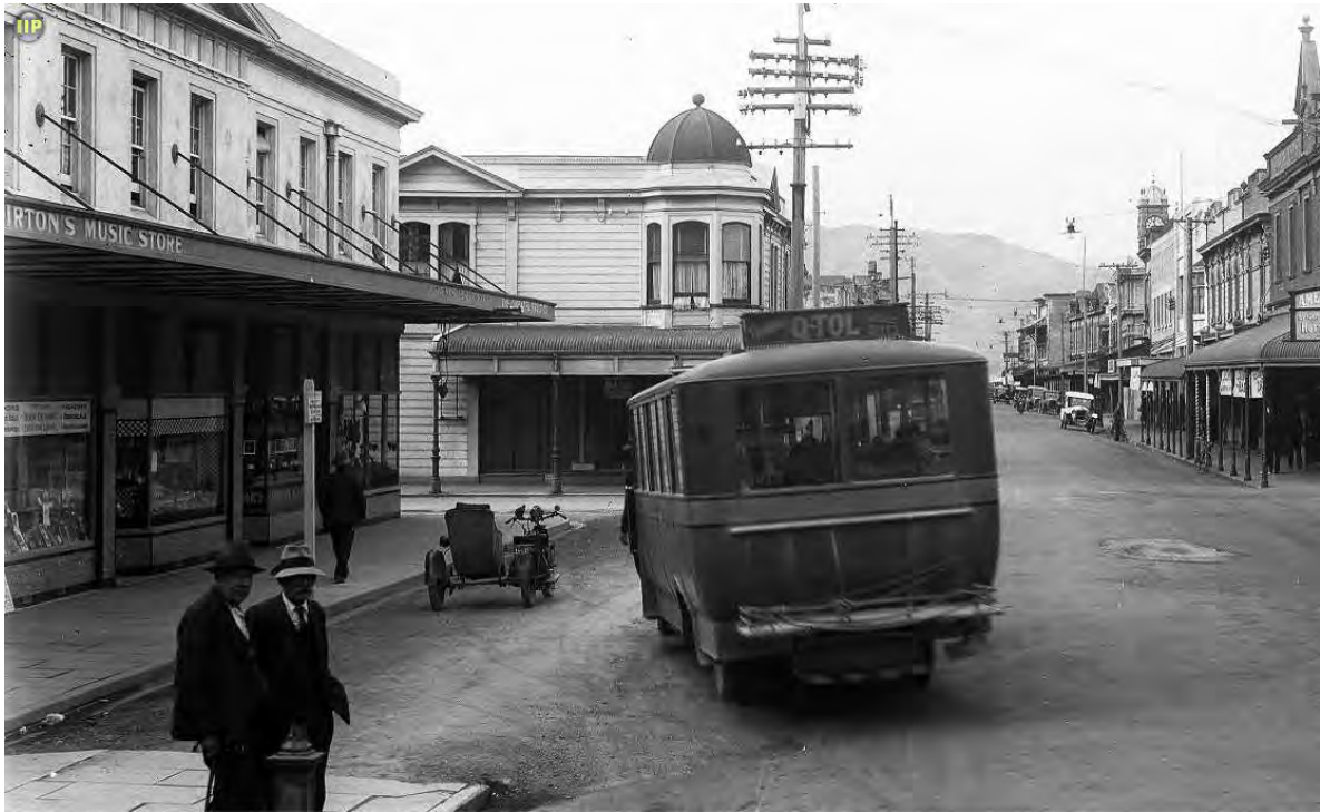
131-141 Jackson Street (left), 1929, showing the new street width set by the building. (1/2-049106-G, S.C. Smith, Alexander Turnbull Library)
