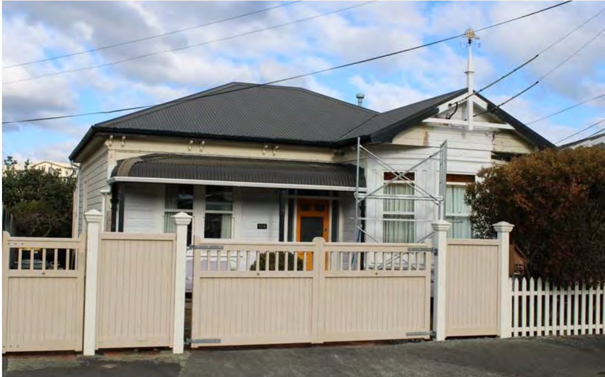
Figure 1: 184 Hutt Road, Lower Hutt.
