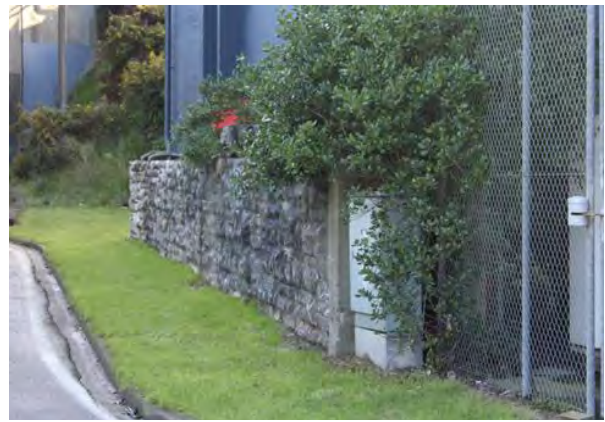
Figure 5: The southern section of wall with no posts or coping.
