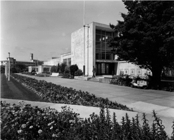
Figure 4: The completed buildings, 1966. Source: HCC Archives.
