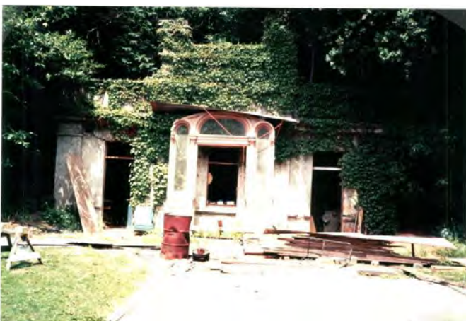
Figure 2: Balgownie Generator Building, c. 1994. Source: HCC Heritage Inventory, 1994.
