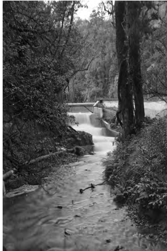
Figure 3: The Korokoro Dam, 1912. Source: ATL, ID: APG-0133-1-2-G.
