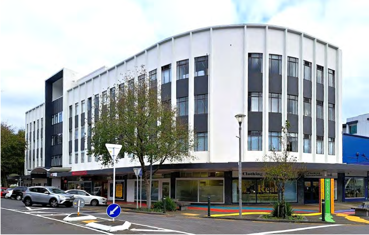
2-18 Laings Road, Hutt Central, June 2024
