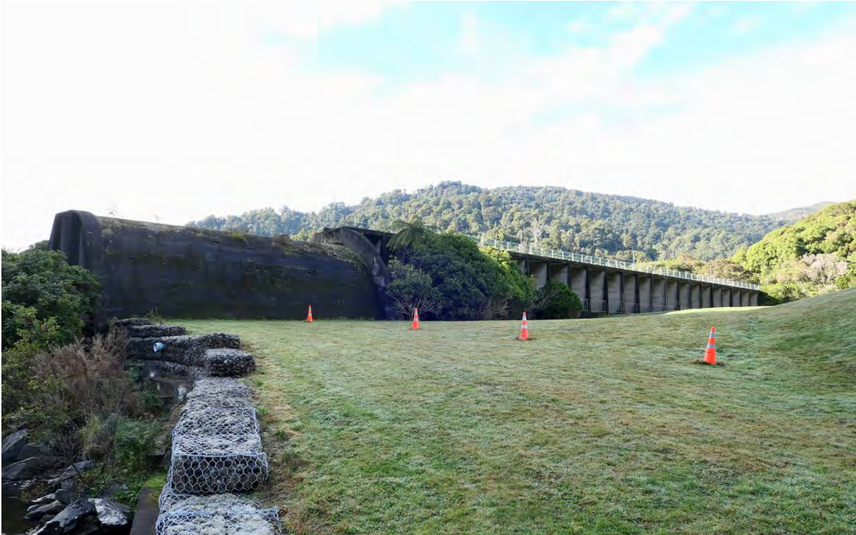
Morton Dam, June 2024
