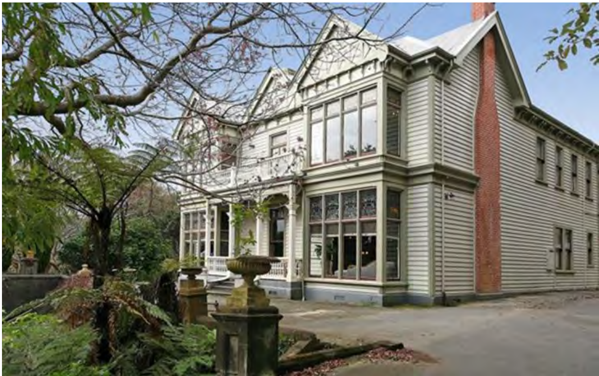
Figure 1: Balgownie House, 16 Hamerton Street.
