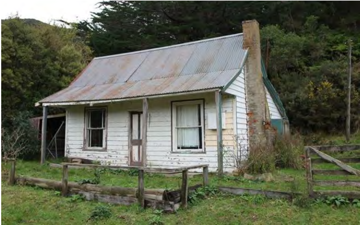
Figure 1: Jacksons' Farm Cottage at 728 Coast Road, Wainuiomata, 2008.
