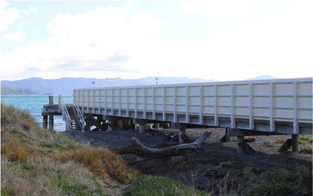
Figure 1: Rona Bay Wharf.
