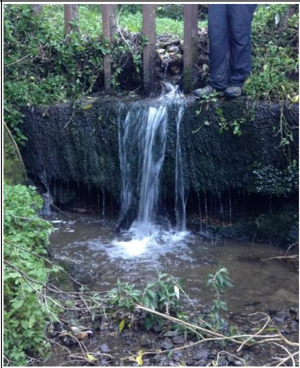
Photo 30: Fish Barriers: A concrete bund and debris trap in stream B immediately upstream of the culvert beneath SH2.
